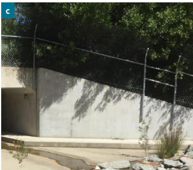
Figure 5 A variety of escape structures on the Pacific Highway upgrade: an escape ramp at Woolgoolga (a), escape hump at Halfway Creek (b), and a culvert wing-wall drop-down at Urunga (c). Escape poles for koalas (d) were installed on the Compton Road upgrade in Brisbane. (Sandpiper Ecological)
