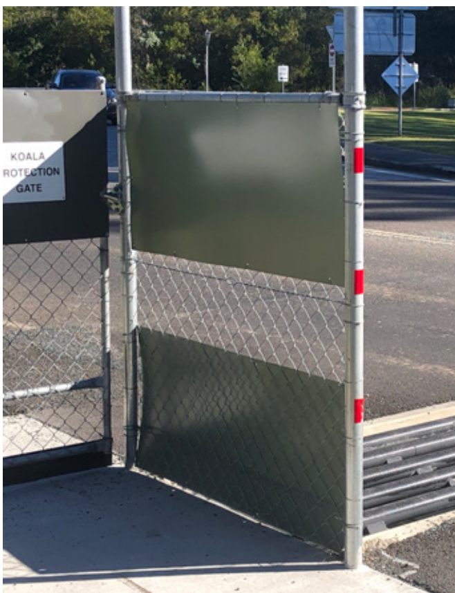
Figure 4 Koala grids have been installed at numerous locations where continuous fencing encounters a crossroad, such as in Byron Local Government Area. (Sandpiper Ecological)
