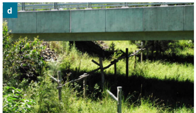
Figure 2 Koalas have been recorded using crossing structures at numerous locations across NSW including a land bridge near Sleepy Hollow (a), and box culverts near Halfway Creek (b) and Warrell Creek (c). Bridge underpasses, such as at Pine Creek complete with refuge poles and timber post-and-rail furniture (d), provide koalas safe passage under highway corridors. (Sandpiper Ecological)
