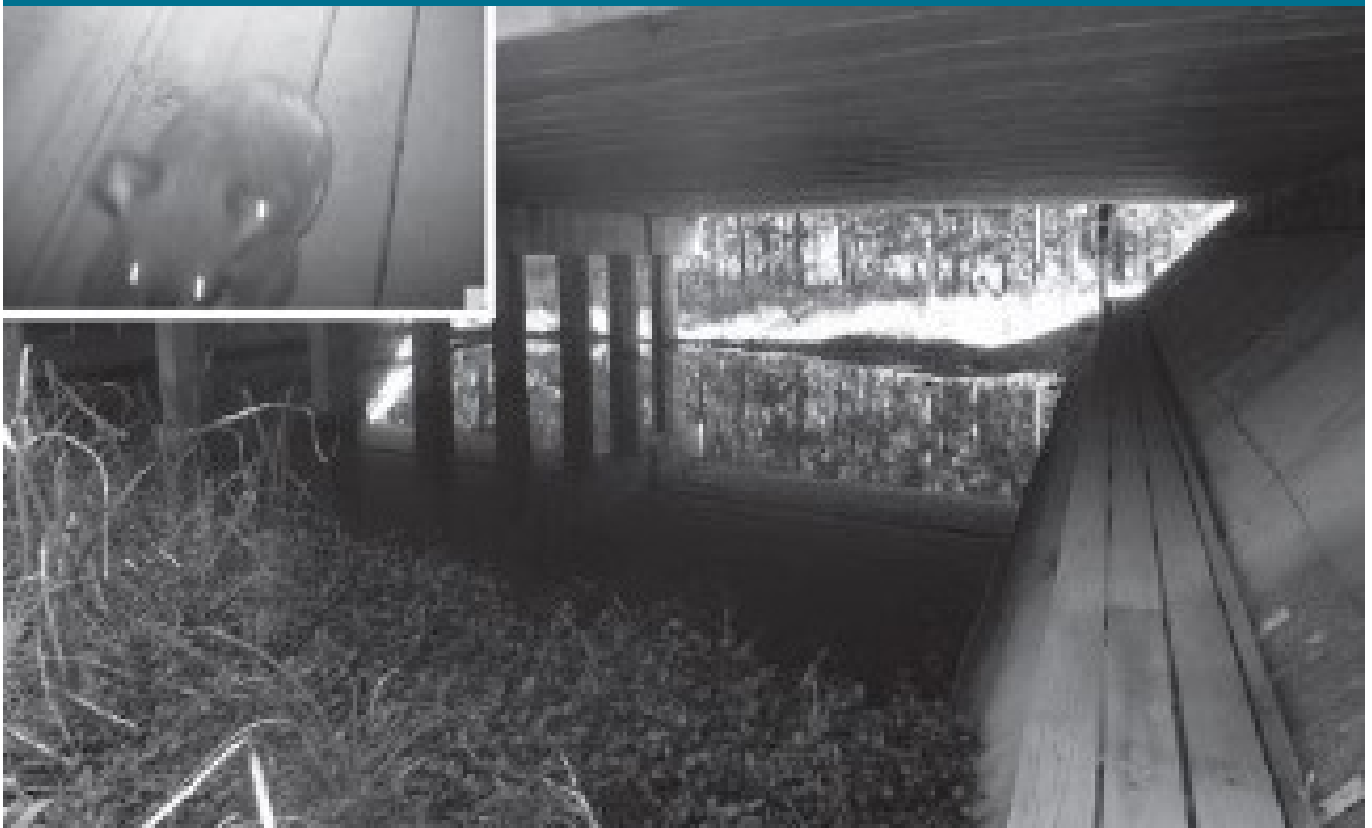
Figure 3 Ledge along the edge of a bridge batter and photograph of koala using the ledge. (Sandpiper Ecological)
