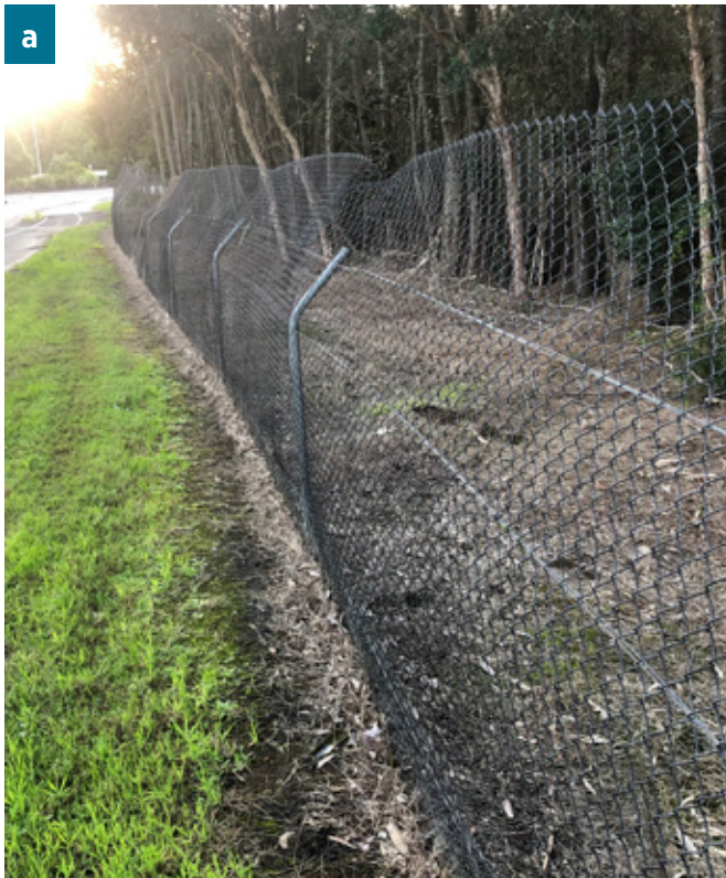
Figure 1 Floppy-top wildlife fencing (a) and 1.5-metre-high chain-mesh fence with flashing (b), feature on long sections of the Pacific Highway upgrade in northeast NSW. (Sandpiper Ecological)
