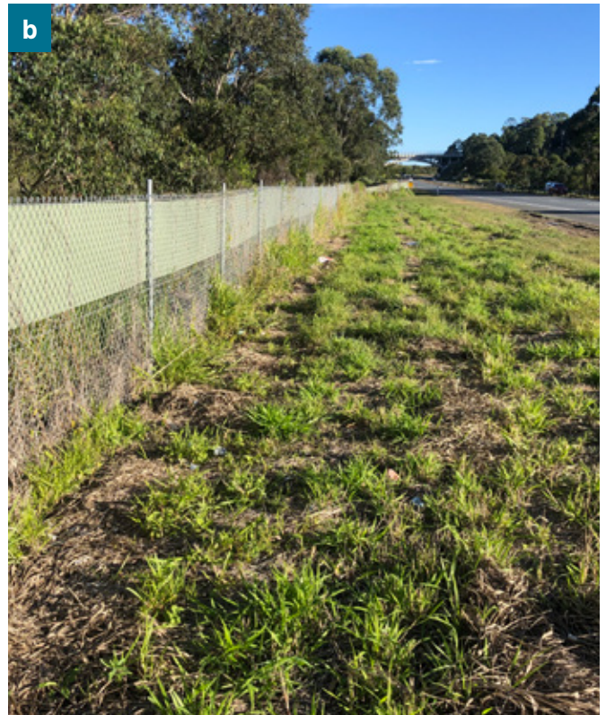
Figure 1 Floppy-top wildlife fencing (a) and 1.5-metre-high chain-mesh fence with flashing (b), feature on long sections of the Pacific Highway upgrade in northeast NSW. (Sandpiper Ecological)
