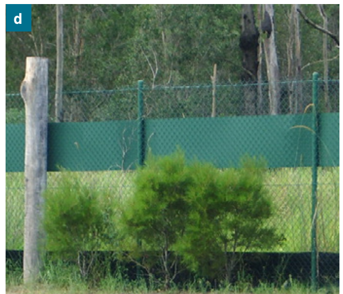
Figure 5 A variety of escape structures on the Pacific Highway upgrade: an escape ramp at Woolgoolga (a), escape hump at Halfway Creek (b), and a culvert wing-wall drop-down at Urunga (c). Escape poles for koalas (d) were installed on the Compton Road upgrade in Brisbane. (Sandpiper Ecological)
