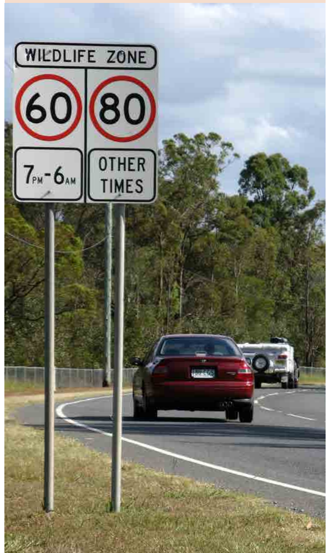
Figure 3 A static sign used in a seasonal speed-reduction trial. (Deidre de Villiers)
