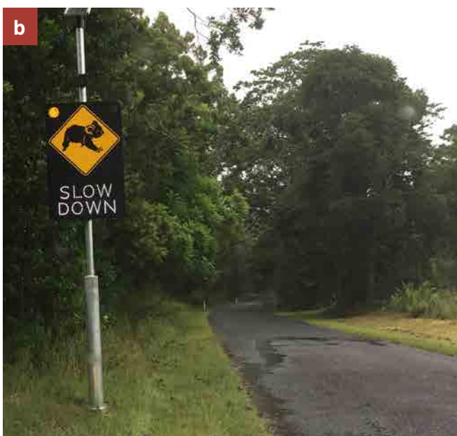
Figure 1 Example of a static koala sign (a) and a dynamic koala vehicle-activated sign (b) installed in the Ballina Local Government Area. (Sandpiper Ecological)
