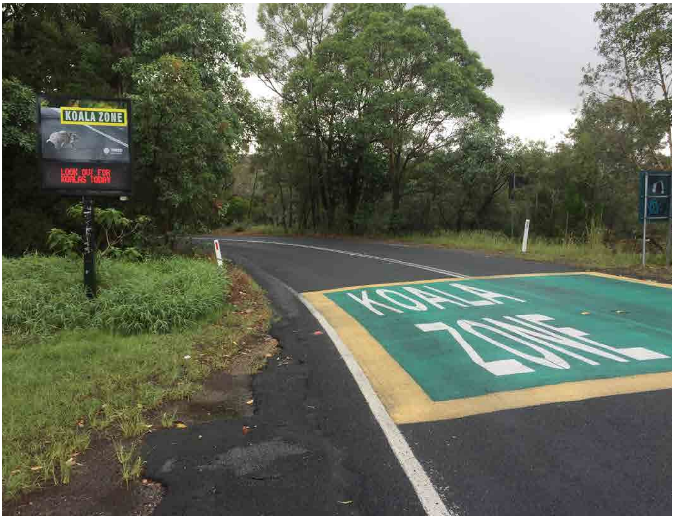
Figure 4 Koala zone road surface marking adjacent to a variable message sign installed in the Tweed Local Government Area. (Sandpiper Ecological)
