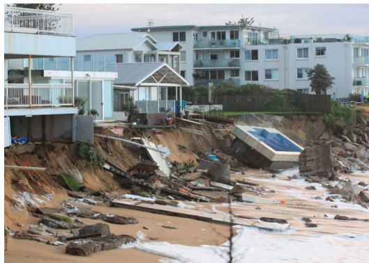
Damage to beach front homes at Collaroy. Source: Peter Rae (taken 2016)
