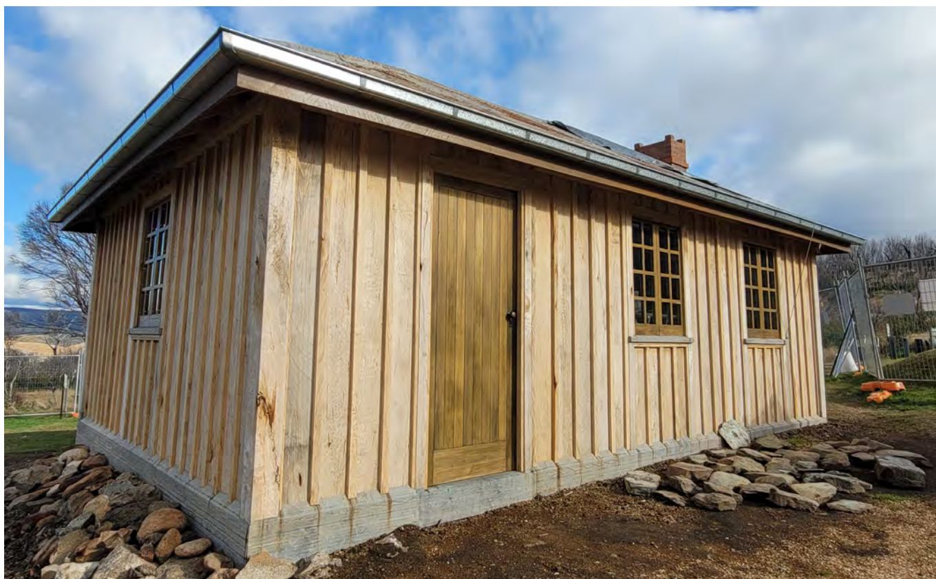
Newly completed Sawyers Rest Hut. Photo: M Bowden/EES Resort Round-up Winter 2022
