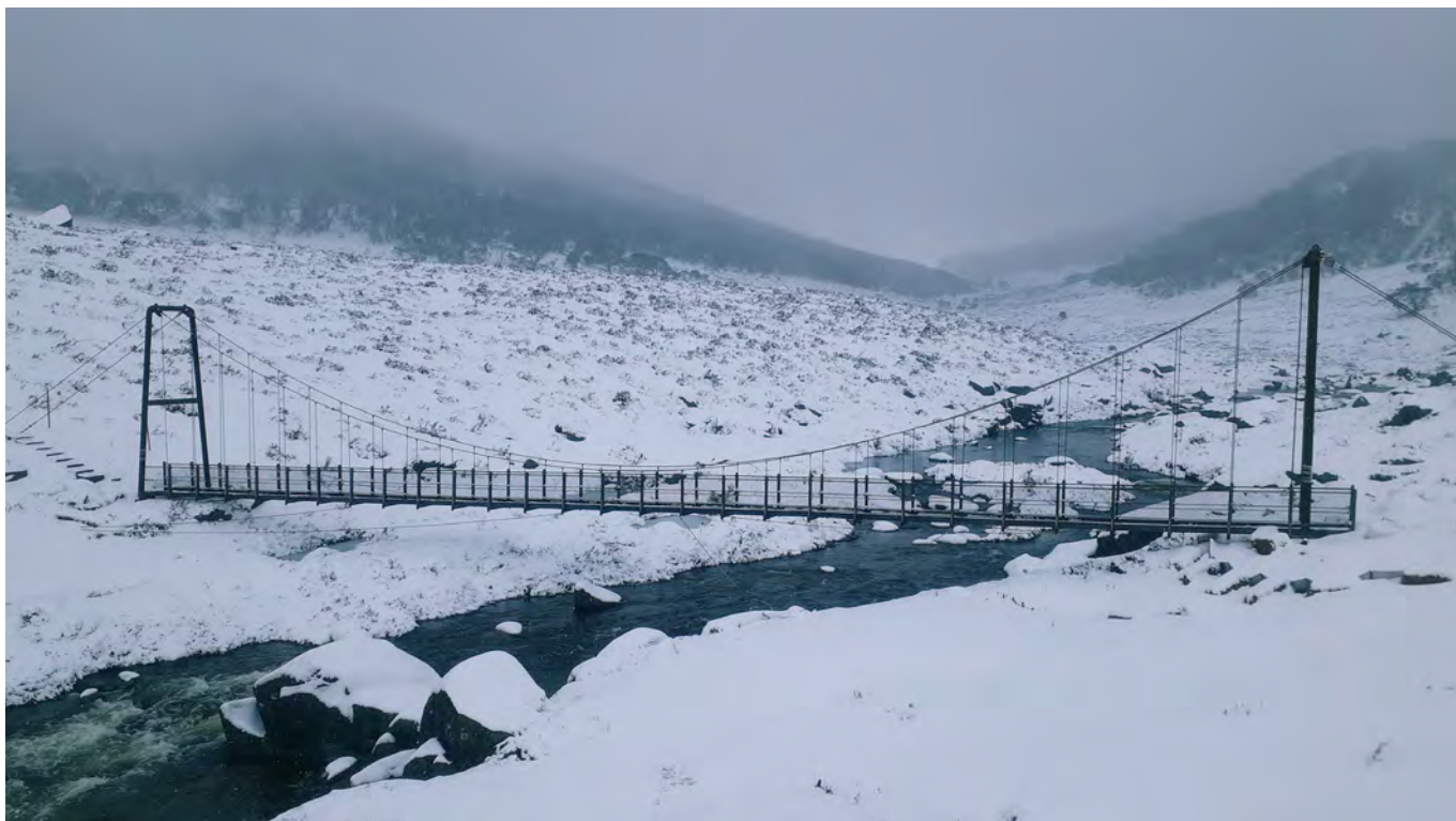
Spencers Creek suspension bridge. Photo: A Cahill/EES
