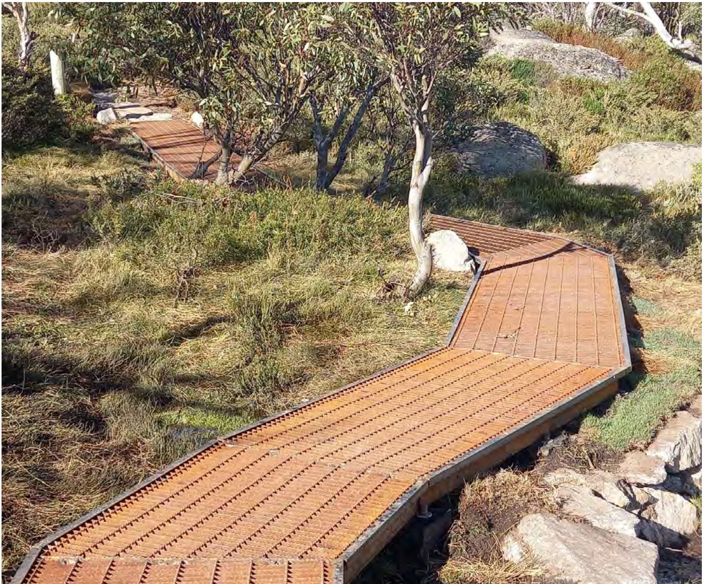
Steel mesh elevates the Porcupine walking track above the sensitive alpine bog habitat. Photo: G Harmer/EES
