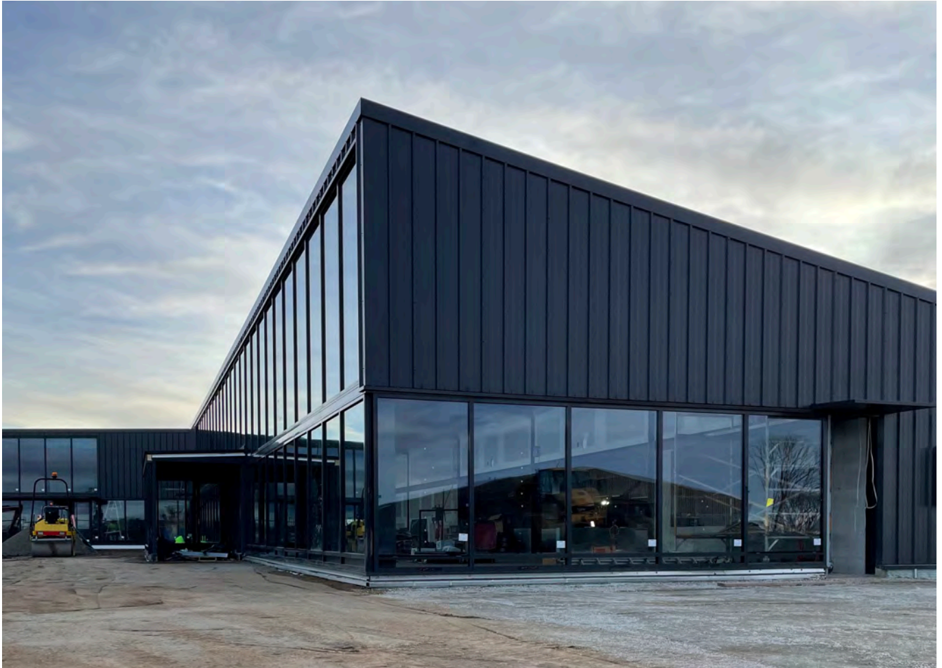
The new Selwyn Complex is nearing completion. Photo: Selwyn Snow Resort
