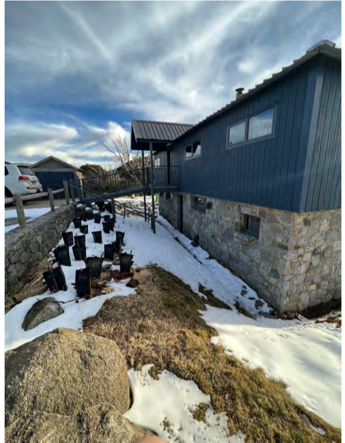
Moerlina Lodge after revegetation works. Photo: N Maude
