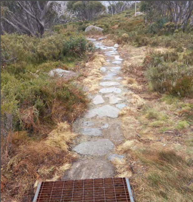
Porcupine paving Photo: G Harmer/EES
