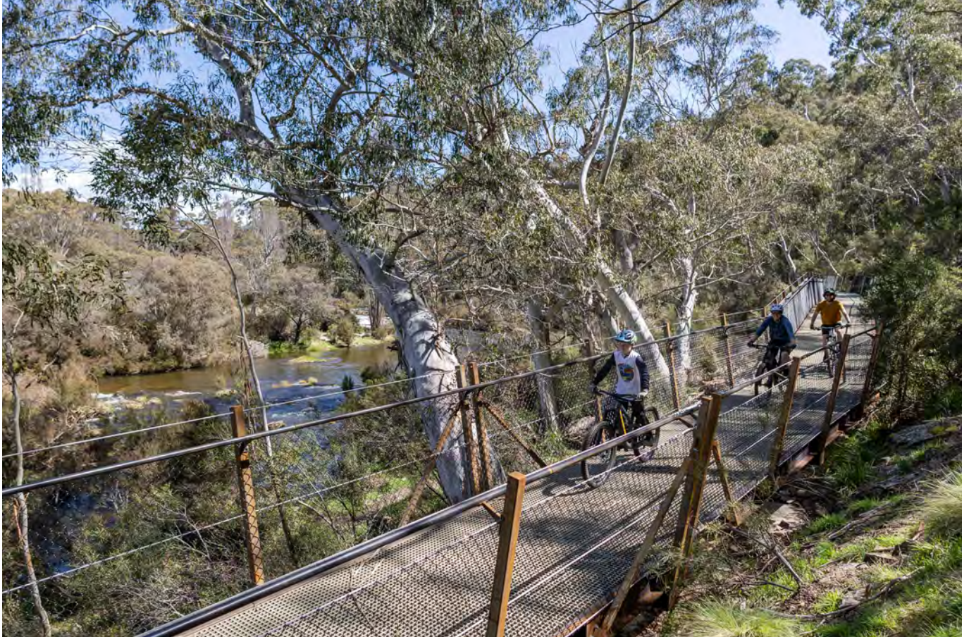
Elevated section near Thredbo River picnic area. Photo: B Ferguson/EES
