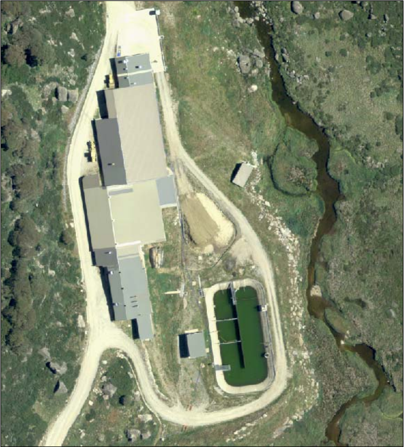
Map 3. Aerial photo of Perisher Valley Sewage Treatment Plant.
