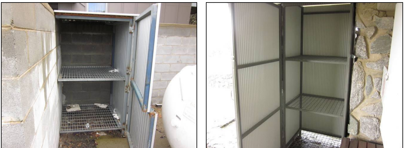
Figure 12 – Waste room interiors showing shelving (photos Tom Pinzone/OEH)
