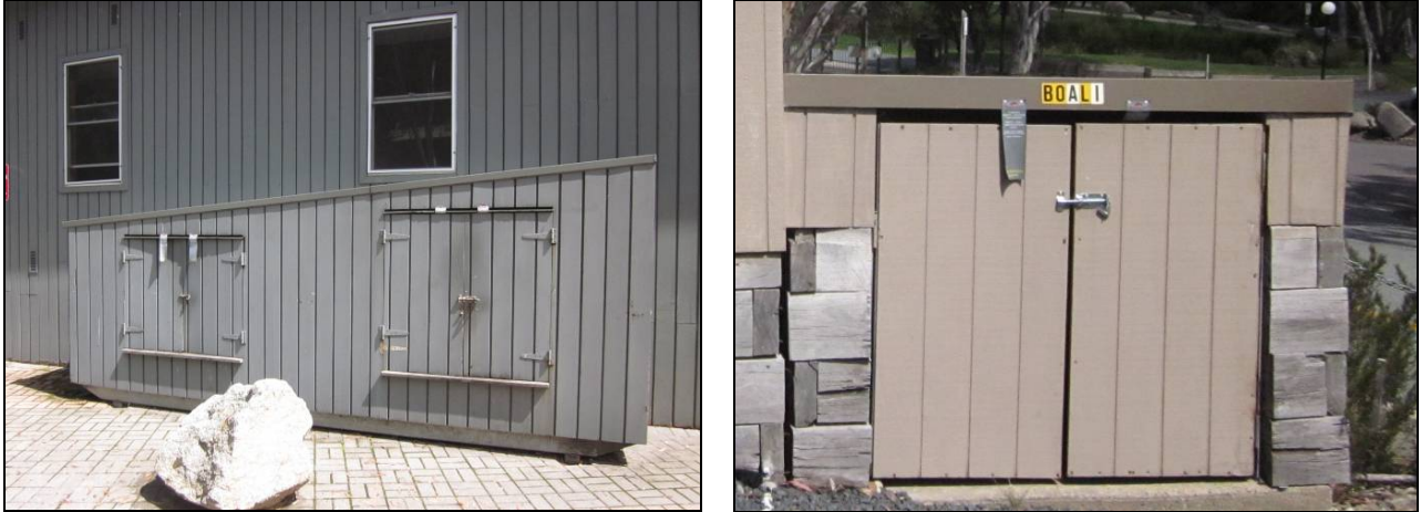
Figure 5 – Acceptable cladding examples (photos Tom Pinzone/OEH)
