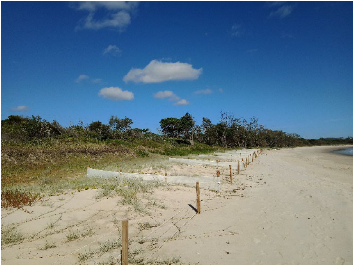
Photo 7 North-easterly alignment of existing sand-trap fencing, Sandon Beach, 2023
