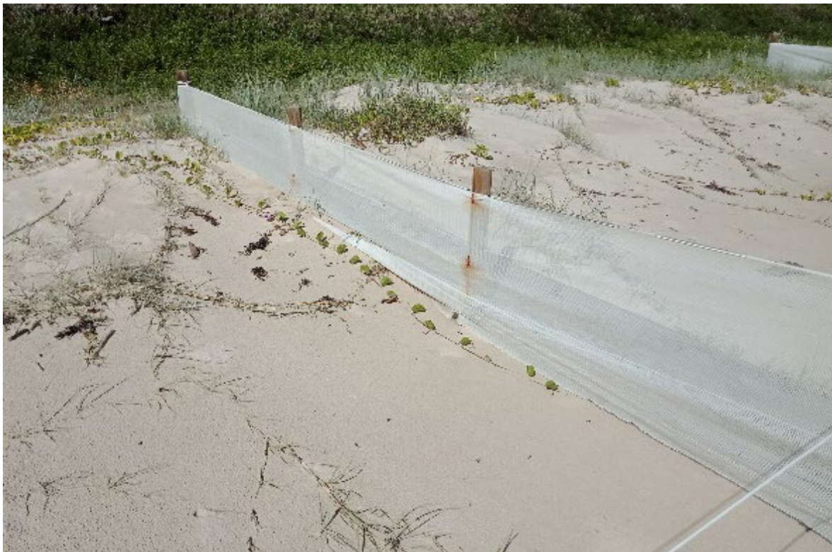
Photo 8 Close-up view of a sand-trap fence, Sandon Beach, 2023
