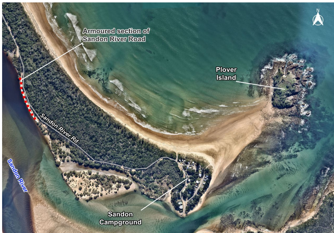
Figure 2 Aerial view showing section of Sandon River Road armoured with rock protection, 2024
