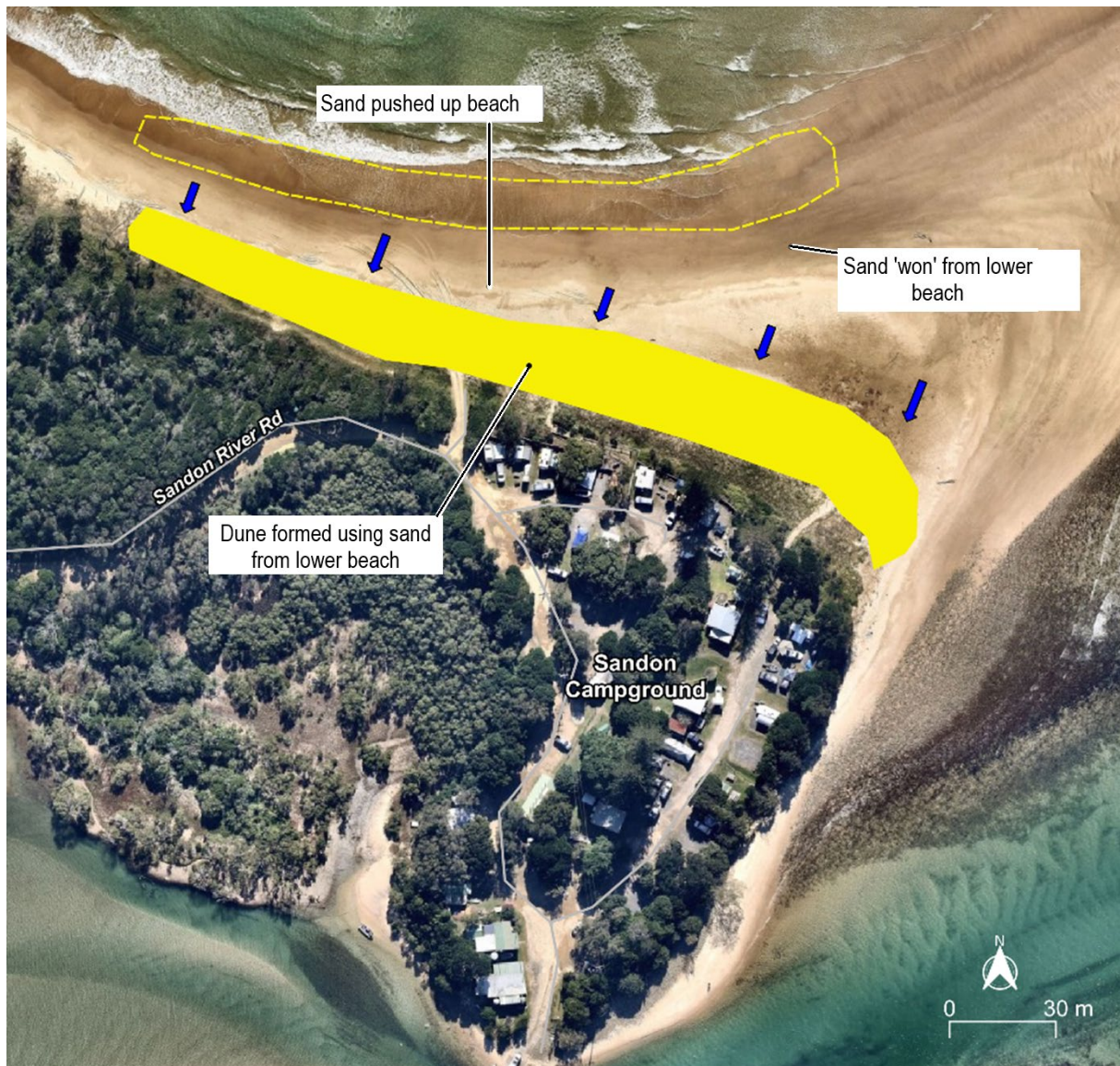
Figure 11 Aerial view showing location of potential beach scraping area to protect against erosion
