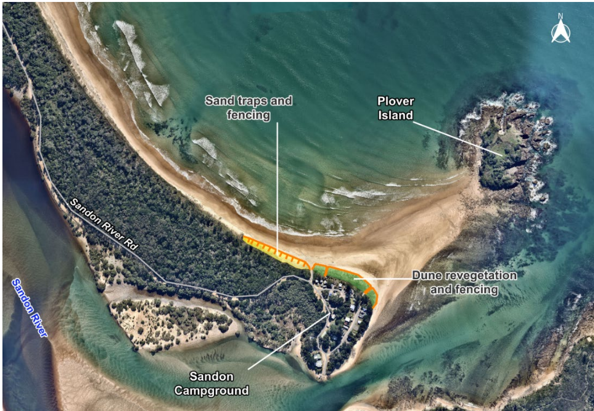
Figure 1 Existing dune stabilisation works, Sandon River campground, 2024
