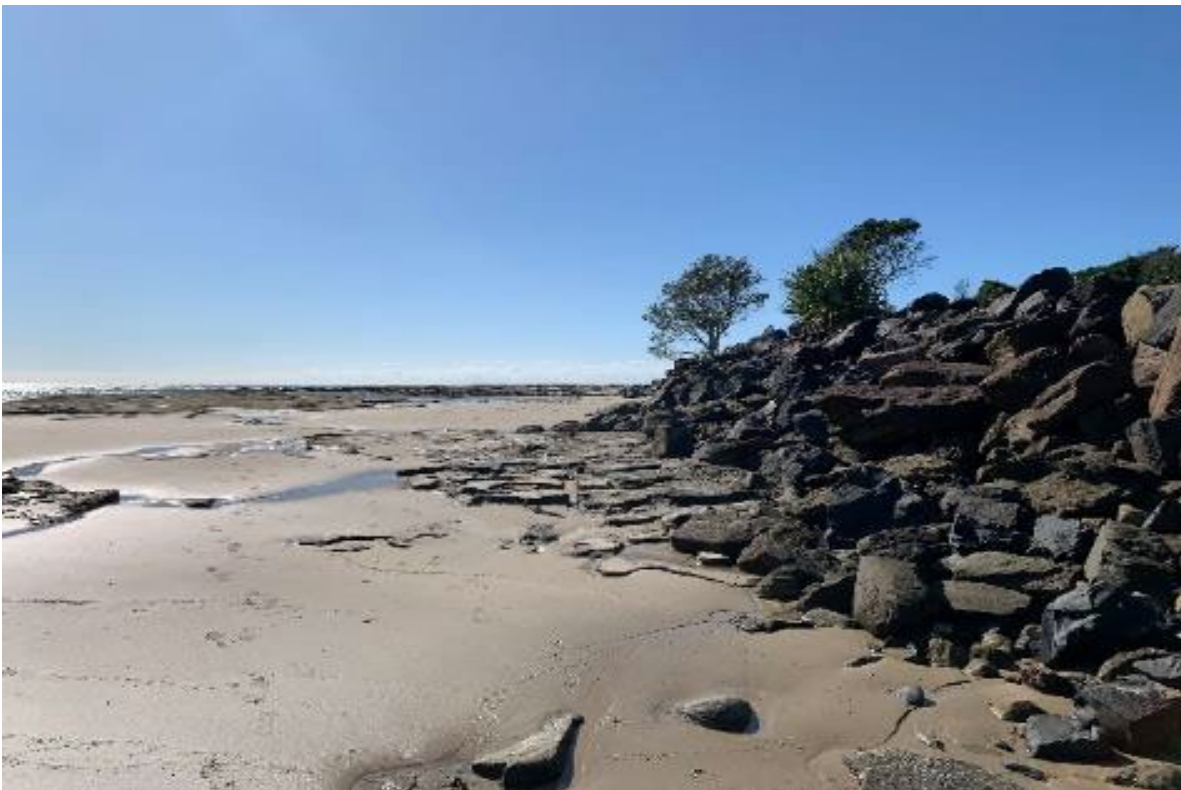
Photo 5 Seawall at Woody Head – photo locations indicated in Figure 2 (July 2020)
