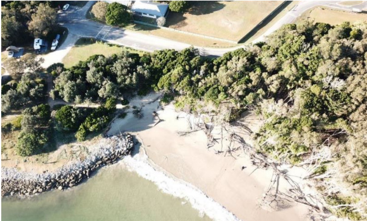
Photo 9 Woody Bay seawall end effects (June 2022)
