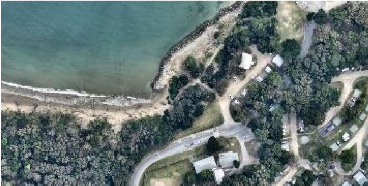
Photo 11 End effect erosion at the western end of the seawall in 2022. Source: Nearmap, 11 September 2022
