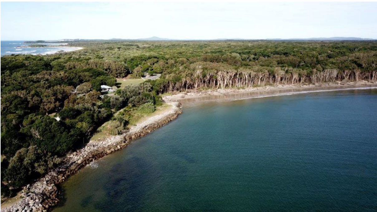
Photo 8 Woody Bay shoreline recession aerial view showing seawall and impacts on vegetation (June 2022)
