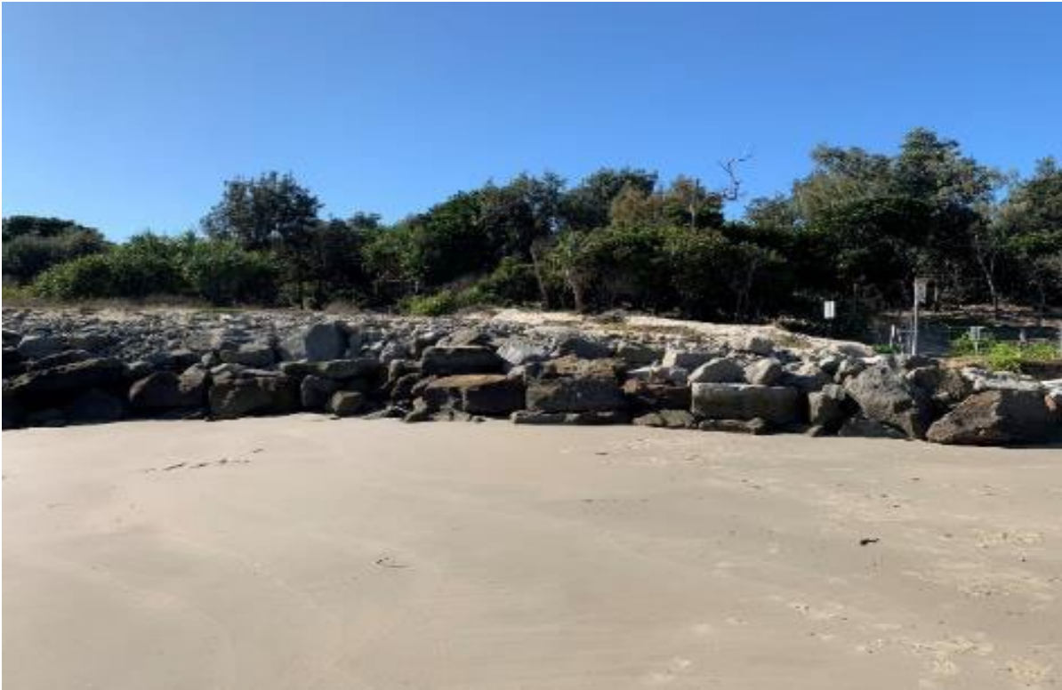
Photo 4 Seawall at Woody Head – photo locations indicated in Figure 2 (July 2020)
