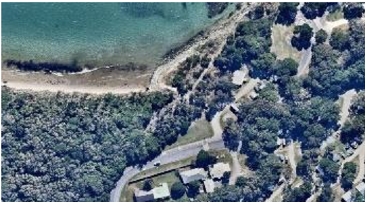
Photo 10 End effect erosion at the western end of the seawall in 2016. Source: Nearmap, 28 May 2016
