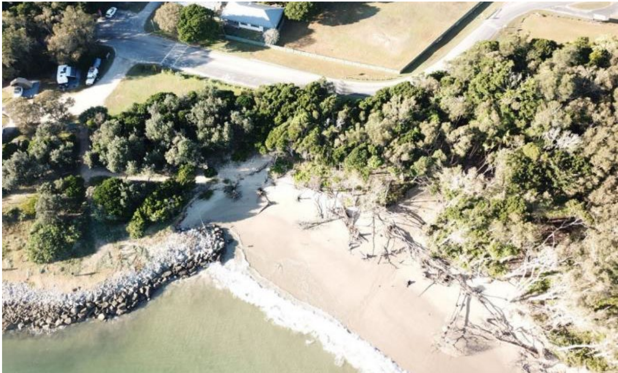
Photo 9 Woody Bay seawall end effects (June 2022)
