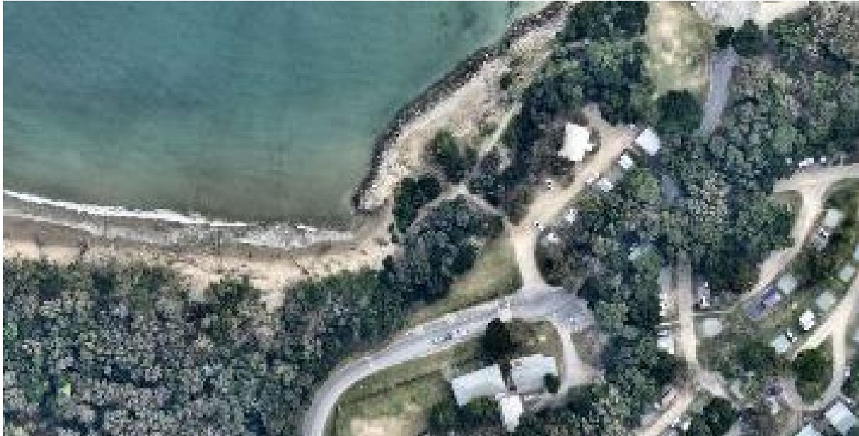
Photo 11 End effect erosion at the western end of the seawall in 2022. Source: Nearmap, 11 September 2022
