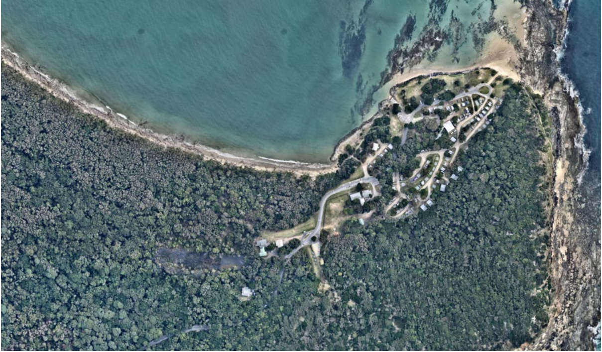
Photo 24 September 2022 – visible beach recession and increasing seawall end effects
