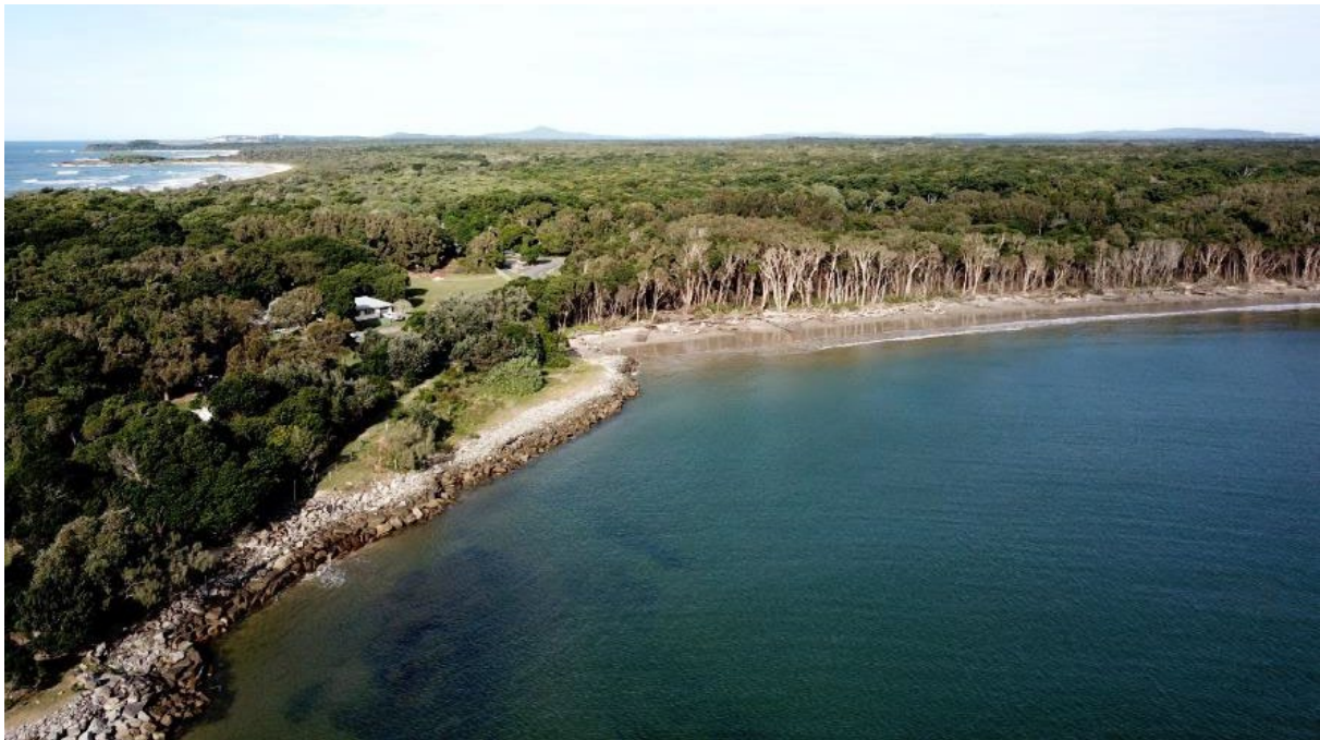
Photo 8 Woody Bay shoreline recession aerial view showing seawall and impacts on vegetation (June 2022)
