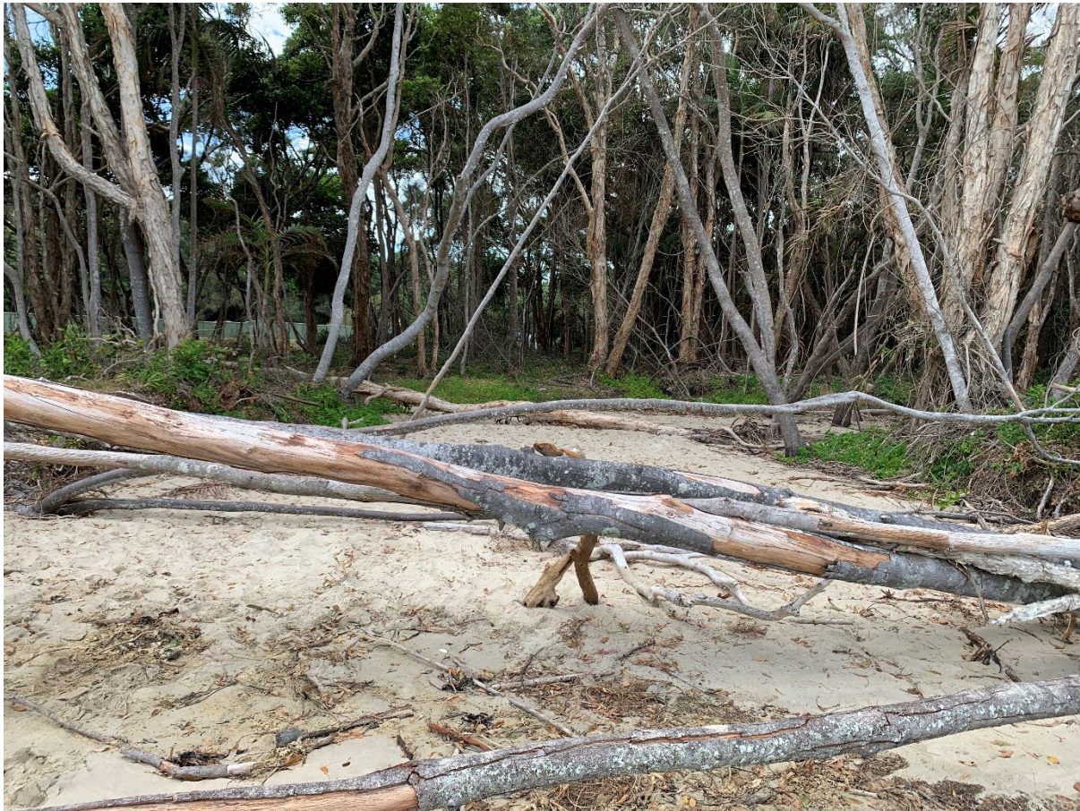
Photo 6 Surface water breakout to beach (November 2022)
