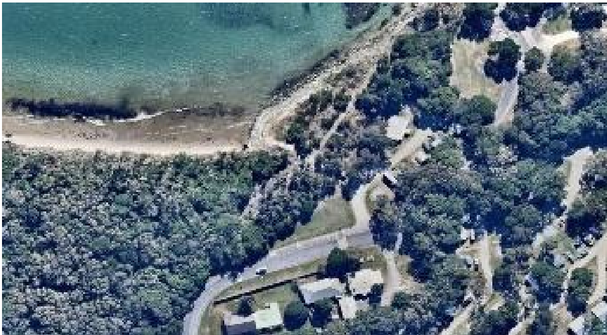
Photo 10 End effect erosion at the western end of the seawall in 2016. Source: Nearmap, 28 May 2016
