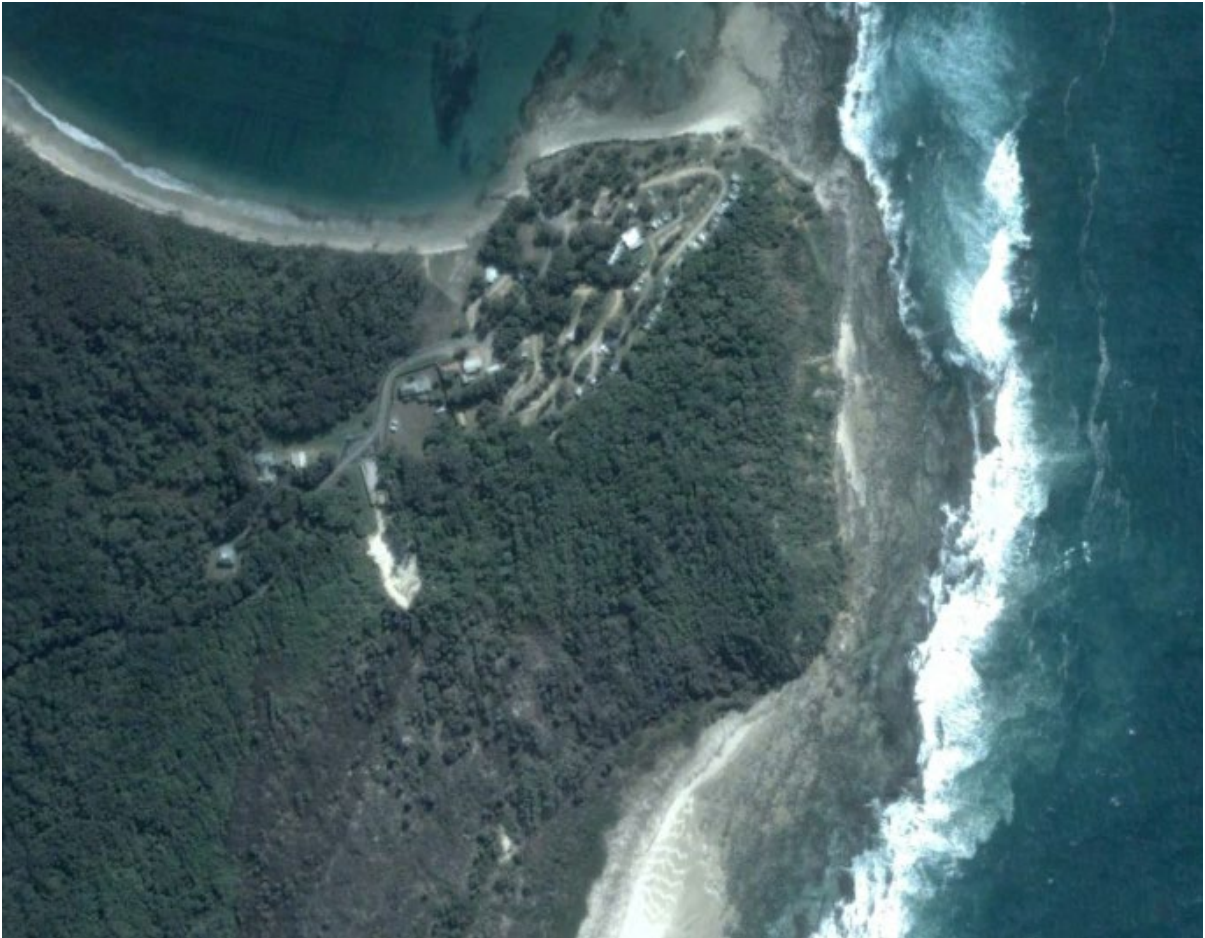
Photo 21 July 2006 – showing clearing for construction of artificial dune (western extent of Woody Bay is not included in the aerial photograph)
