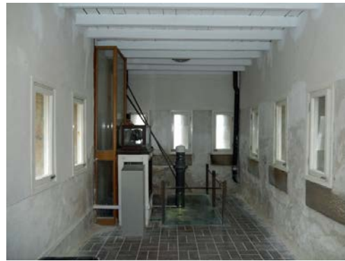
(d) Tide Gauge Room looking north-west, showing tide gauges
