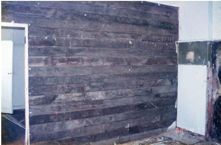
Figure 45 The timber partition formerly dividing Rooms B6 and B7 (NPWS 1997)
