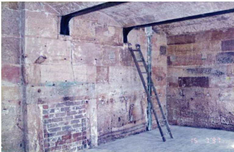
Figure 46 Room B6/B7 after removal of render, showing bricked up fireplace (NPWS 1999)
