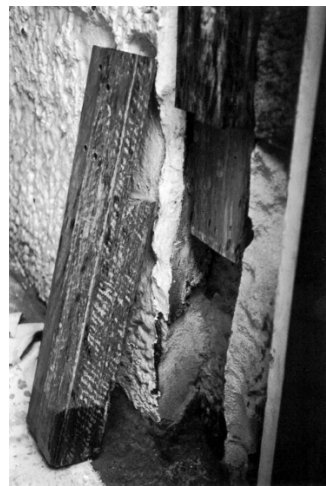
(f) Door jamb with new base ready to splice
