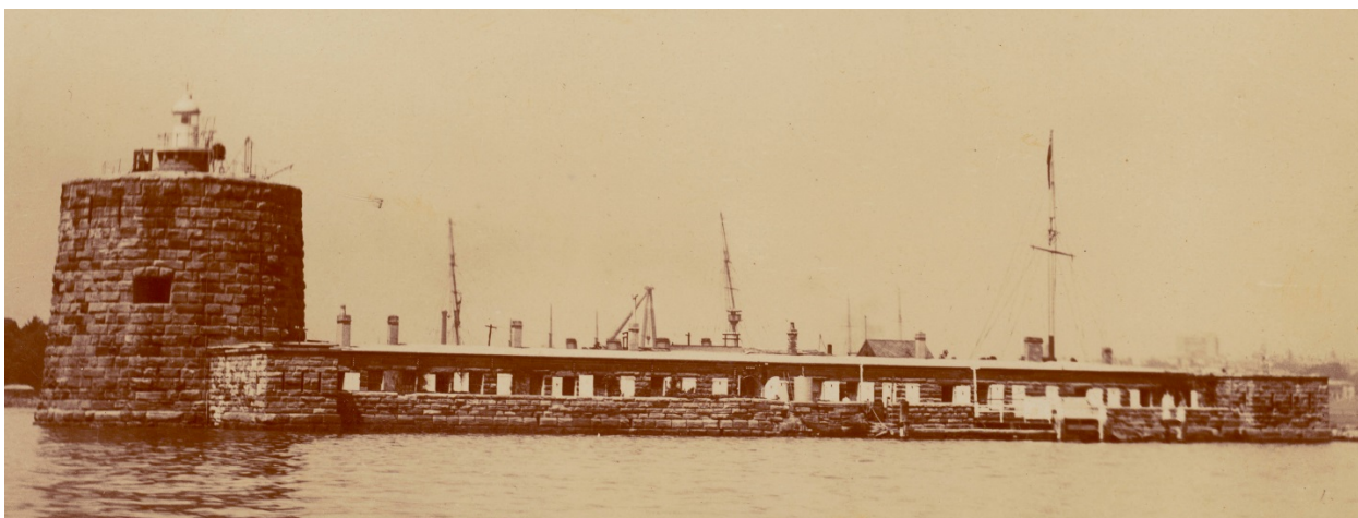
Figure 18 Fort Denison after 1915, showing the new light, reconstructed Tide Gauge Room and the new wharf (State Library of NSW, Star Photo a_089117u)
