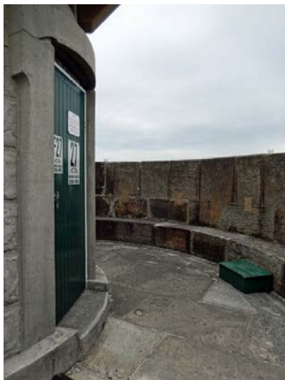
(e) Tower terreplein and parapet, with lantern structure (left) and firing step
