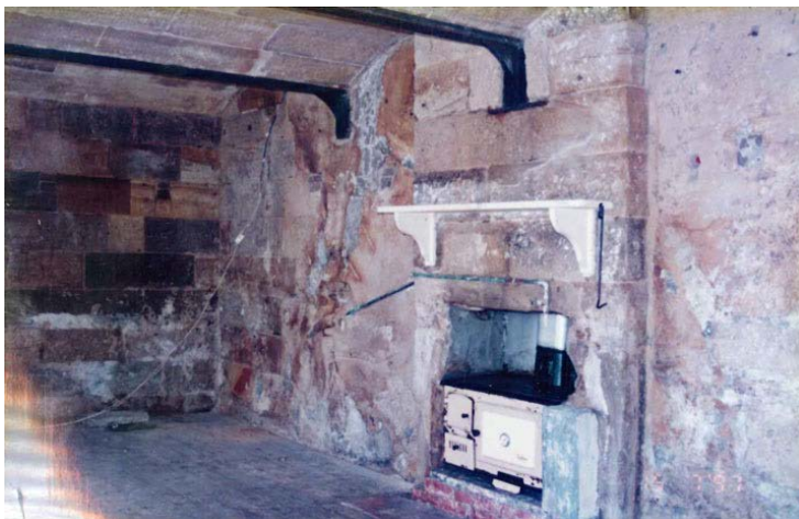
Figure 40 Room B4 looking east, after removal of render (NPWS 1997)
