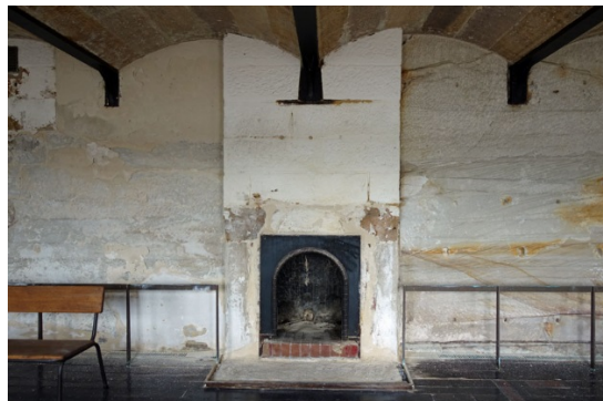
(h) Detail of fireplace in Room B5
