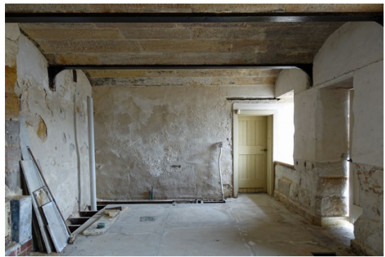
(d) Room B4 looking south-west
