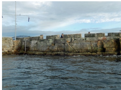
(f) Battery from the east (2016)
