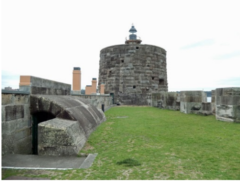
(a) Battery looking north-east
