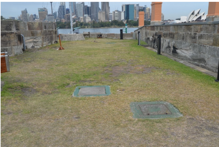
Figure 63 View south-west along the battery towards the bastion, with the barracks to the right. Several service and tank access points are visible in the foreground (Casey & Lowe 2018)
