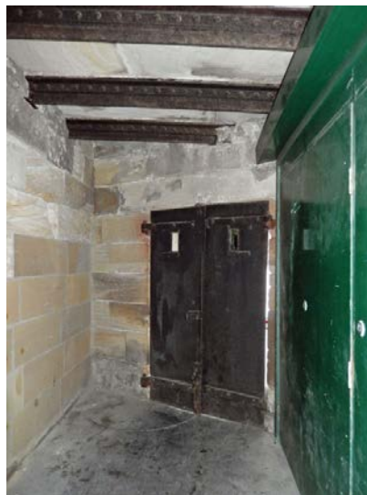
(d) Room W3 looking south-east
