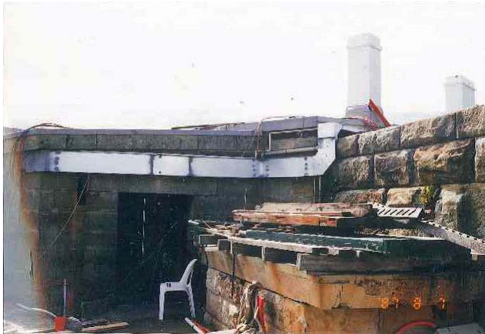
Figure 57 The water tanks in the slip yard removed (NPWS 2000)
