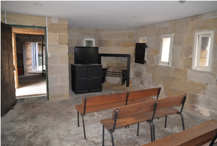
Figure 73 Interior view of West Room W1, looking south. Most of the interior fabric, including the sandstone wall surfaces, was replaced in the 1970s and a new concrete floor installed in 1983 (Casey & Lowe 2018)
