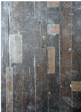
(e) Detail of floorboards in Room B5 (2018)
