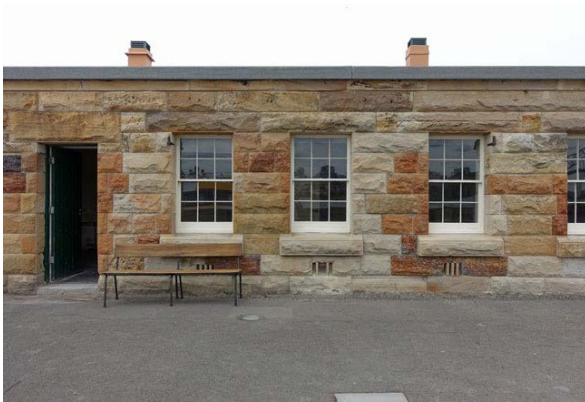
(c) Typical elevation of barracks outside Room B5 (2018)
