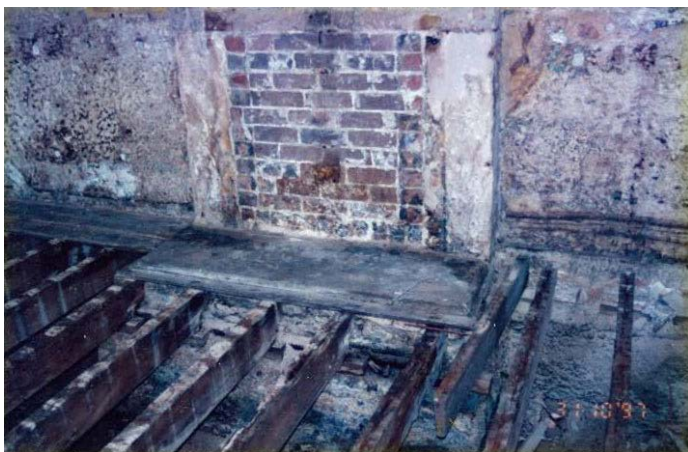
Figure 32 Floor structure in Room B6/B7 after removal of floorboards (NPWS 1997)
