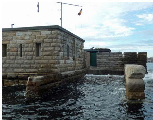
(f) Exterior of West Room, slipway and slip yard looking east
