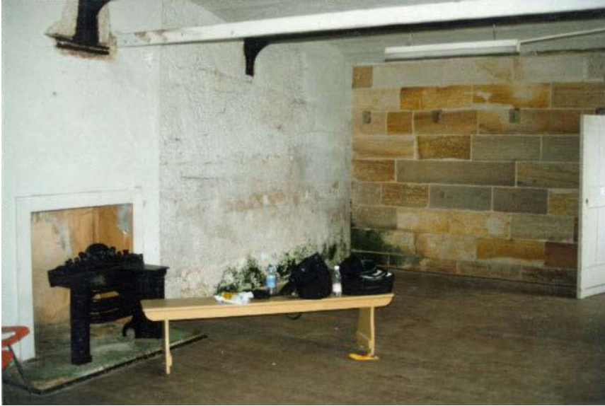
Figure 48 Room B11 after metal conservation, showing high level timber rail (NPWS 1997)
