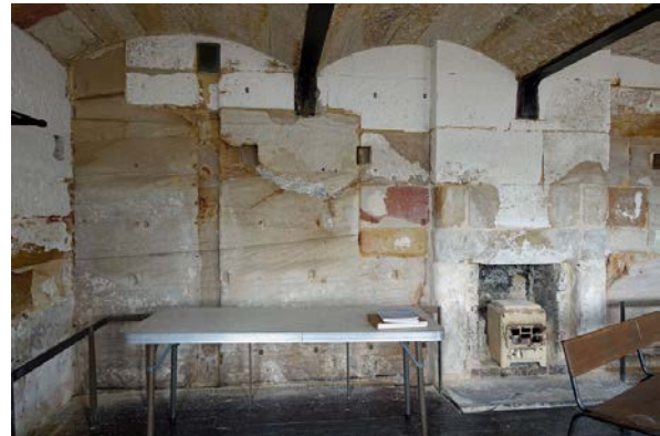
(d) Room B6/B7 looking south-east, showing fireplace and chases for floor vents (2018)
