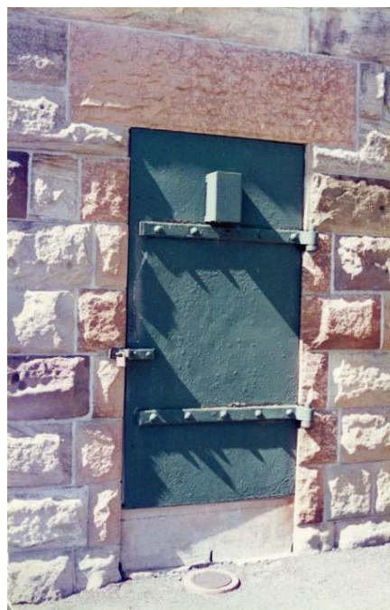
Figure 50 Room B15 (left) before conservation and fitting out, and the former external door to this room converted for an explosives store with a reused iron shutter (NPWS 1997)
