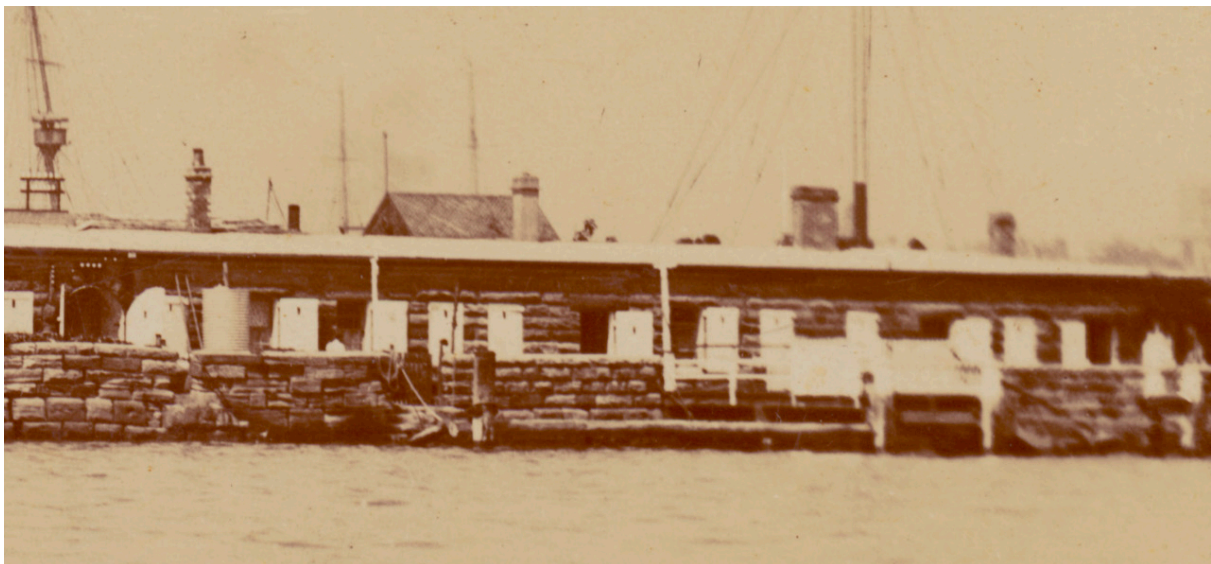
Figure 52 Photo taken after 1913 showing original landing steps on left and 1901 wharf on right (Detail from State Library of NSW, Star Photo a_089117u.)
