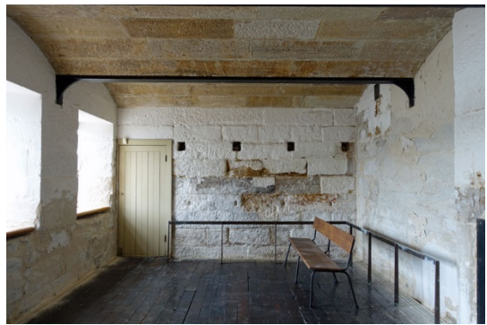
(f) Room B5 looking north-east
