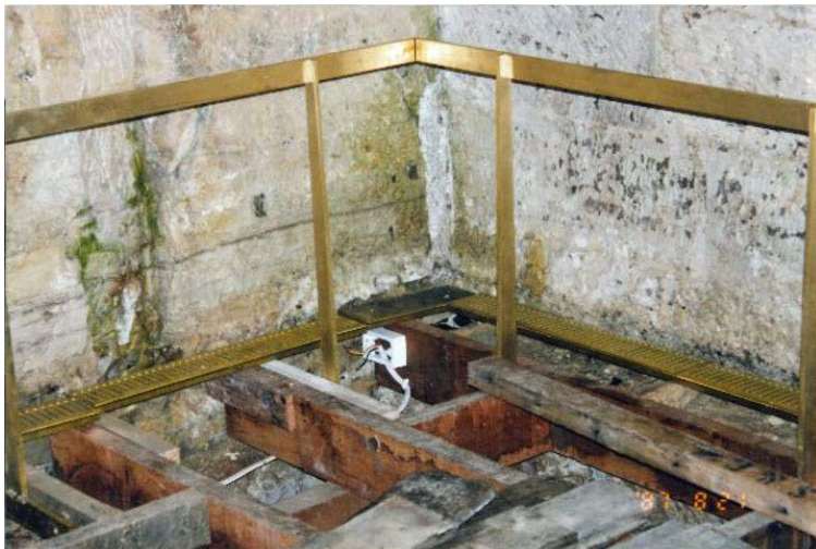
Figure 44 Installation of brass ventilation grilles and balustrades, Room B5 (NPWS 1999)
