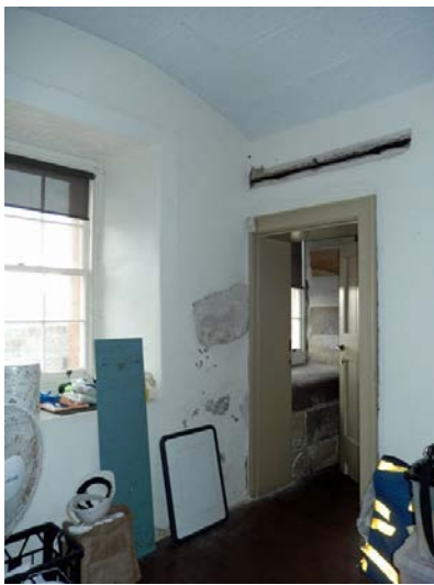
(c) Room B12 looking north
