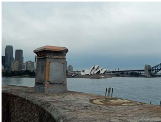
(c) Parapet and chimney on tower terreplein
