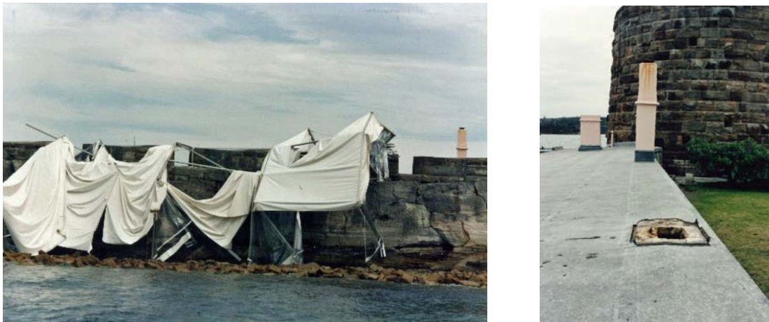
Figure 30 Storm damaged marquee (left) and detail of missing chimney demolished by the same storm (NPWS 1996)
