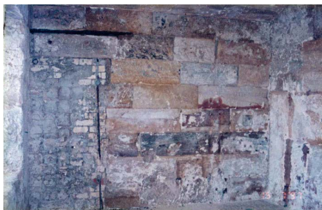
Figure 35 Room B2/B3 looking north (left) showing partition and tiling being removed, and north-east wall (right) after render removal, showing bricked up former doorway (NPWS 1997)
