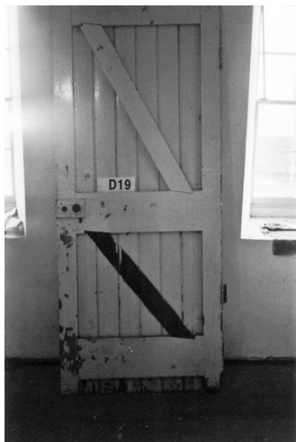
(e) Door removed
