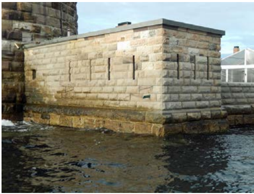
(c) Tide Gauge Room exterior from north
