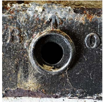
Figure 36 Room B2/B3 looking east (left), following the removal of render in 1997, showing the plumbing manifold embedded in the wall (NPWS 1997), and detail of the Board of Ordnance stamp on the plumbing manifold (right) (Orwell & Peter Phillips 2018)
