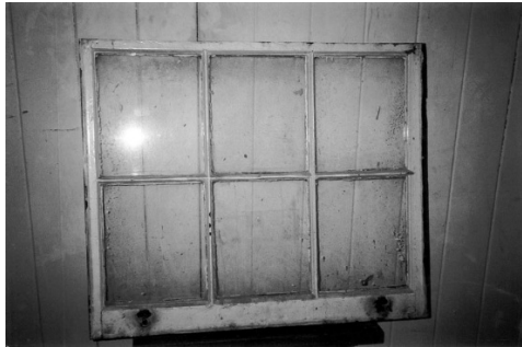
(a) Window sash removed
