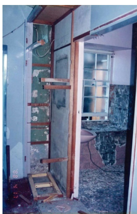
Figure 35 Room B2/B3 looking north (left) showing partition and tiling being removed, and north-east wall (right) after render removal, showing bricked up former doorway (NPWS 1997)
