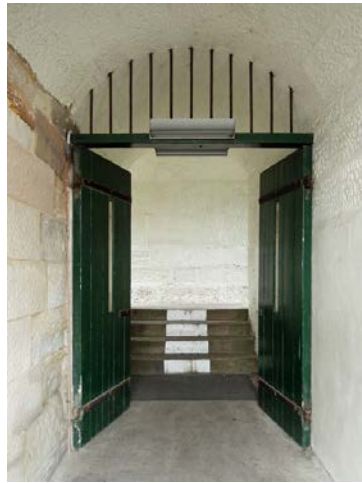
(b) Room B8: doors and steps to battery
