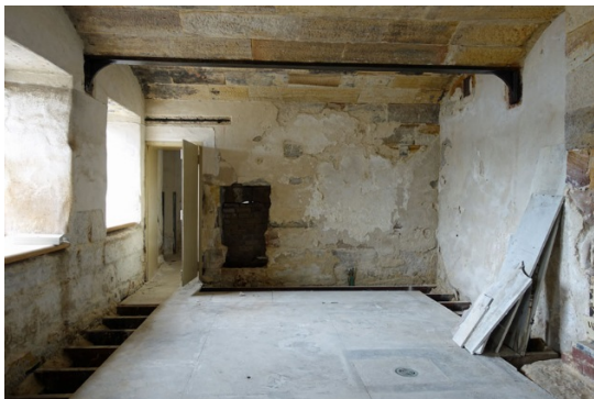
(c) Room B4 looking north-east
