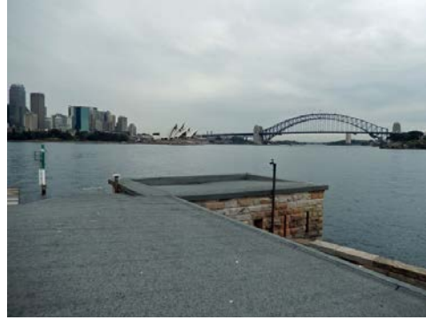
(b) Barracks roof looking west (2016)
