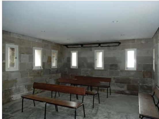
(b) Room W1 looking west
