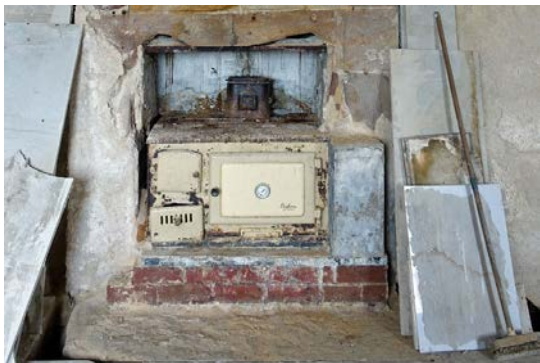
(e) Detail of fireplace in Room B4
