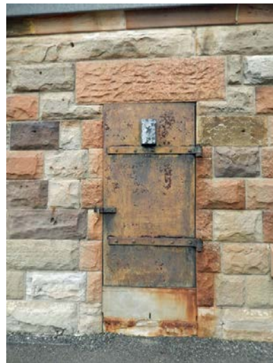
(f) Iron shutter, barracks wall (2016)
