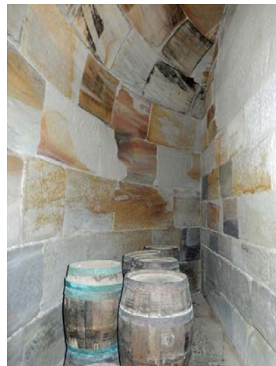
(f) Room TB1 looking east
