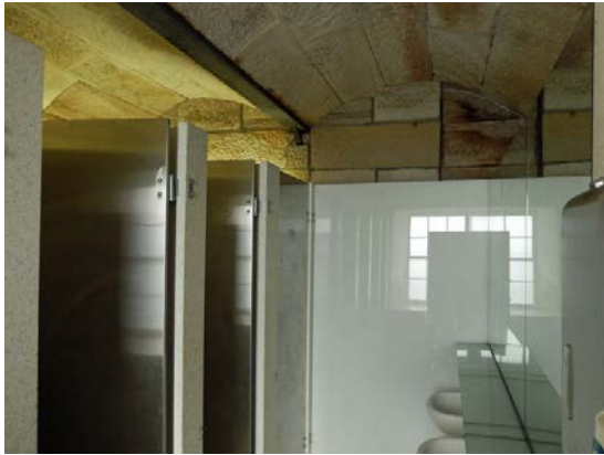
(a) Room B15 looking south-east
