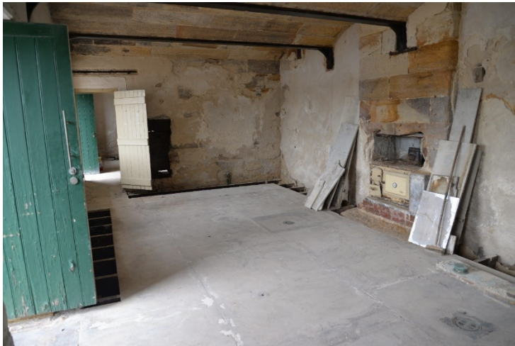
Figure 70 Interior view of barracks Room B4 looking east. Excavations were undertaken in this room during 1997–98 and consisted of the complete removal of floorboards and all subsurface deposits. The room served as the Fort Denison café/restaurant kitchen from 2000 (when the floor was replaced) until mid-2017 (Casey & Lowe 2018)
