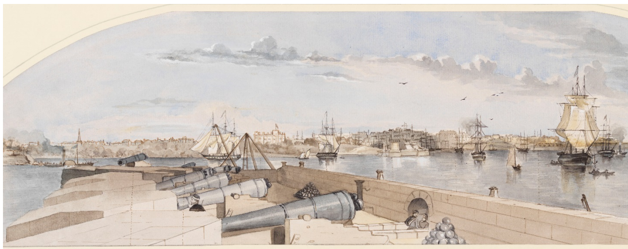
Figure 9 The 10-inch shell gun (left of image) and 32-pounder gun battery on Fort Denison, circa 1859. The image shows several enlisted men of the Royal Artillery garrison and the water tank pump (Wilson, State Library of NSW, a5325001u)
