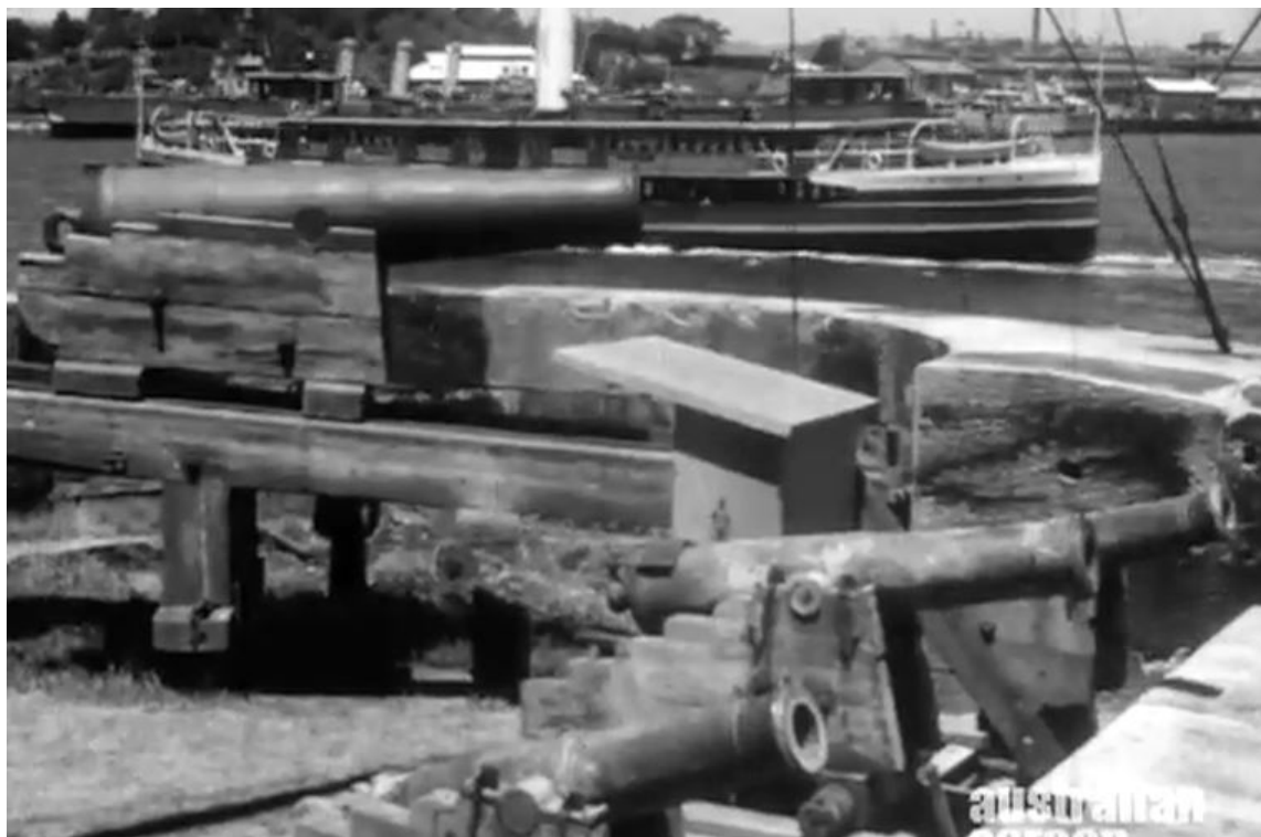
Figure 17 The 8-inch shell gun with original traversing carriage emplaced in the bastion. The brass howitzers, including the one o'clock gun, are on original garrison carriages (Australian Screensound 1936)
