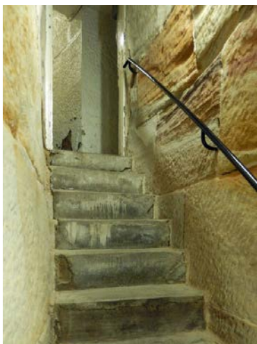
(e) Steps up from Room TB3
