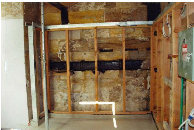
Figure 38 Room B2/B3 looking south-east, showing new framing to walls (NPWS 1998)
