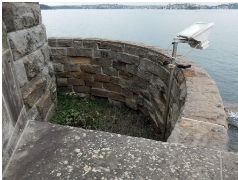
(e) Former ficus bed at base of tower
