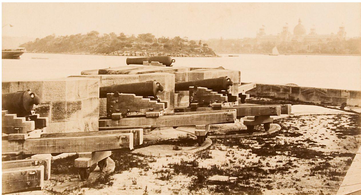
Figure 10 Fort Denison 1879, showing the 32-pounders on dwarf traversing carriages and the 10-inch shell gun en-barbette (91/1323-6 Collection: Museum of Applied Arts and Sciences. Photo: Chris Brothers)
