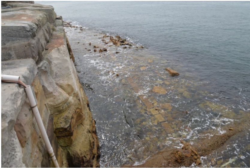
Figure 60 View looking north-east over the south-east face of the battery (from the bastion), showing the wet ditch and breakwater. Sandstone bedrock is visible underlying the parapet at left (Casey & Lowe 2018)
