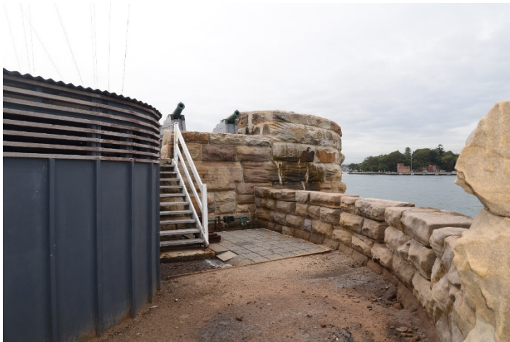
Figure 76 View of the bastion and the 1917 wall of the slip yard, looking east, with a modern shelter to the left (Casey & Lowe 2018)
