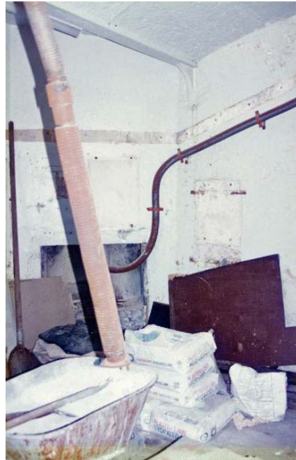
Figure 49 Room B14, showing former door to Room B15 (left) and work in progress to remove services (right) from former use as generator room (NPWS 1997)
