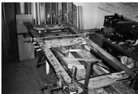
(g) Door frame patched
