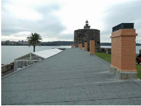
(a) Barracks roof looking north-east (2016)
