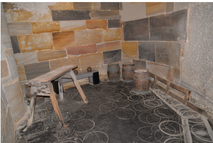
Figure 67 Interior of Room TB4, at the lowest (magazine) level of the Martello tower, looking south. The impressions of later display items (barrels and cases) are visible in the Seysell asphalt coat on floor (Casey & Lowe 2018)
