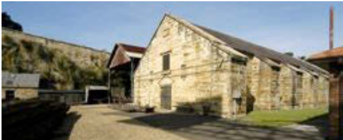
Figure 2.1 The Queen's Magazine is perhaps the most significant built structure on the island. It is unique, the earliest example of a military gunpowder magazine in Australia, largely intact and is an exceptional achievement in terms of construction finesse. It is located within its fortified wall, with all of the magazine buildings built in the 1830's still standing and retaining their relationships to each other (see Figure 2.2 below). It is also now located between the 1925-29 Scow Shed, 1948 and 1963 amenities buildings and a corrugated iron clad addition to the south end of the building from the 1940's. The 1943 Ship Repair Workshop and its extensions to the west largely cut off views between the harbour and the magazine. Each of these structures have their own significance in relation to the later shipyard development of the precinct, however, apart from the 1948 amenities building and the 1943 Ship Repair Workshop, none are now used in relation to the shipyard.
