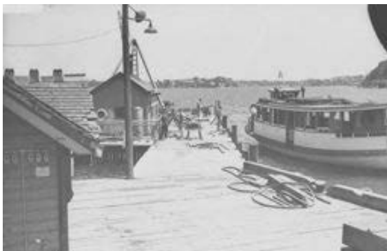
Figure 2.22 Wharf construction c1940.
