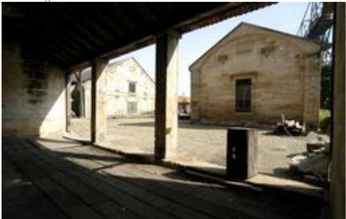
Figure 2.2 The Magazine Precinct, as viewed from verandah of the Stores Building (2 nd cooperage) (20), showing the relationship of the early magazine period buildings to each other. Paul Davies 2007.
