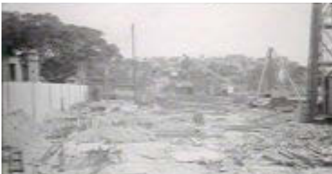
Figure 2.55 1947: Building construction: Goat island (Source: State Library of NSW, GPO 1 – 10054, MSBL958).
