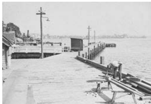
Figure 2.23 Construction of the ferry wharf. Undated
