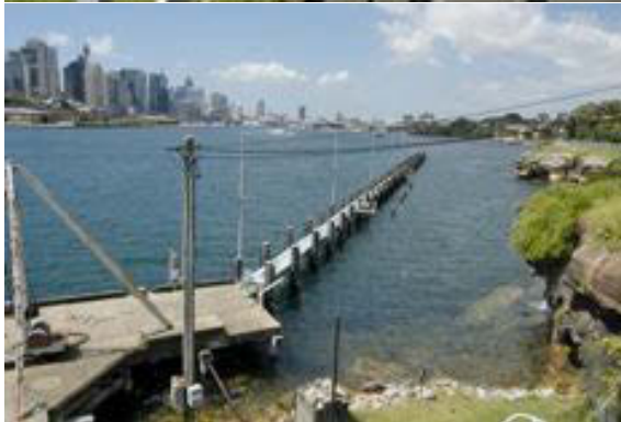
Figure 3.51 The view from the roof of the Port Emergency Services Building (45) looking south along the shoreline of the island towards the city and Darling Harbour. The flat roof of the building provides a large viewing platform with uninterrupted panoramic views.
