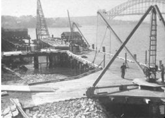
Figure 2.18 Reconstruction of the eastern wharf.
