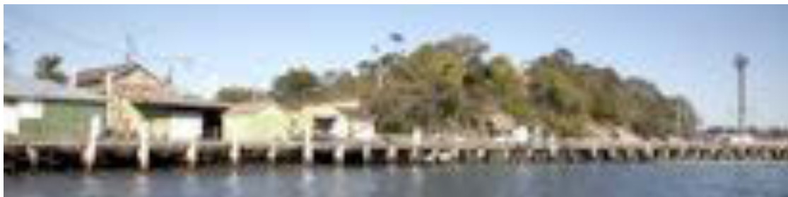
Figure 3.38 A close view of the ferry wharf (54a) and end of the northern wharf (55). This photograph illustrates the changes in visual setting of the wharves with the northern wharf closely related to built development along its edge and stepping up the hill where to the right the ferry wharf is set against the natural escarpment and the vegetated headland. MSB firefighting building (50), various sheds (56, 57) western end of Gear Shed (49) visible, with north elevation of the SHT Fire Brigade Barracks (46b) visible on the promontory behind. Note that the Harbour Master's Residence (39) is virtually invisible from this angle, whereas in the early 20 th century it was prominent from this direction.
