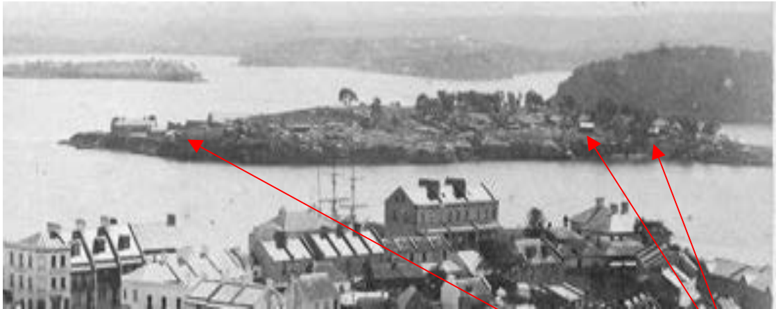
Figure 2.11 Detail of circa 1882 photograph taken from Sydney Observatory looking west shows the two 1870s explosives magazines (1 & 2) and the state of the south-eastern and eastern shore of the island at this time. An outbuilding (3) is visible behind the Barracks Kitchen. This photograph further illustrates the reduction in natural landscape on the island by the late nineteenth century. (Source: City of Sydney Archives image SRC 12220).
