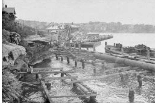
Figure 2.21 This photograph is entitled "New wharves". July 1944.
