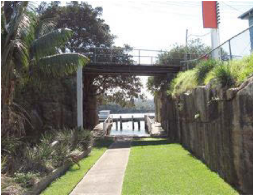
Figure 50: Bridge across 'Barney's Cut' or 'The Cut' - view N (2007)
