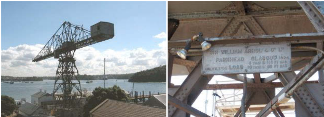
Figure 104: MSB cantilever tower crane – views NW & N (2007)
