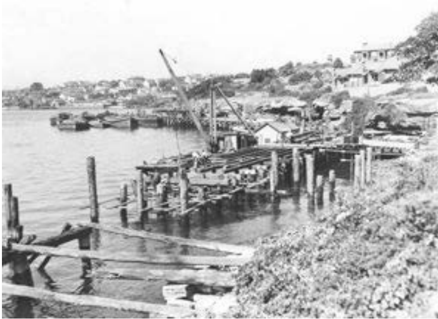
Figure 89: 'Wharf construction, Goat Island' (n.d.)
