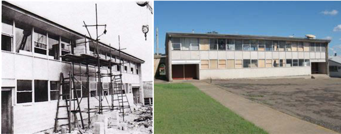
Figure 105: Amenities block under construction (1964) & the block today – view SSW (2007)
