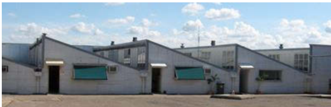
Figure 98: The MSB Shipwrights building - view WNW (2007)
