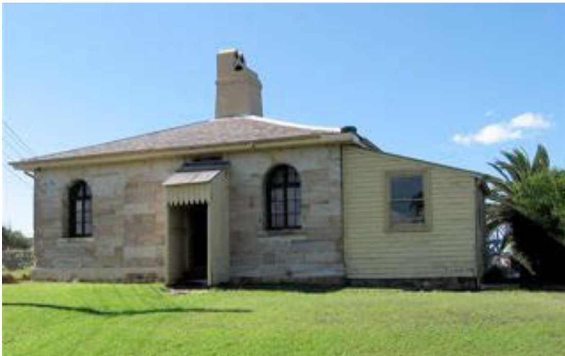
Figure 38: Water Police Station – view E (2007)
