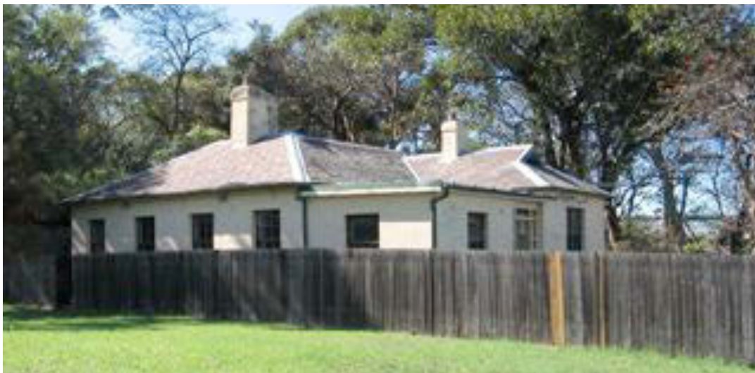
Figure 52: Cook house/guard room, converted to a cottage in 1924/5 – view NNE (2007) (Dan Tuck 2007)
