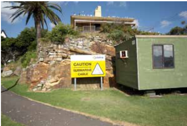
Water Police Station east elevation with intrusive metal demountable (59) below.
