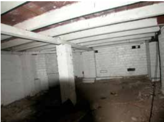
Detail, floor structure from undercroft
