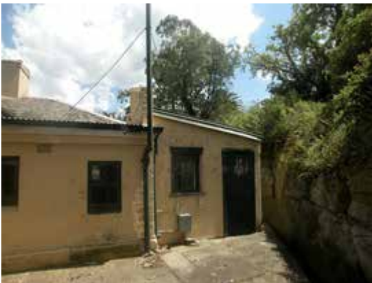
Detail of rear of east elevation, Kitchen cottage
