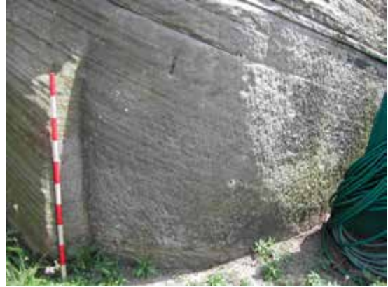
Detail, Lime Kiln
