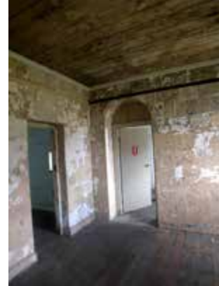
Interior, Water Police Station doorways
