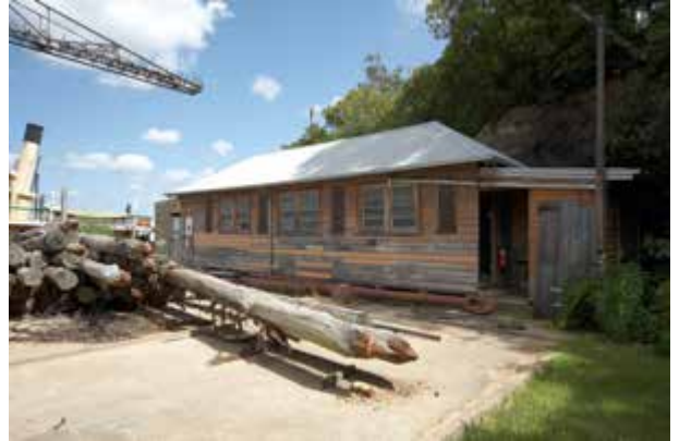
Timber store south elevation
