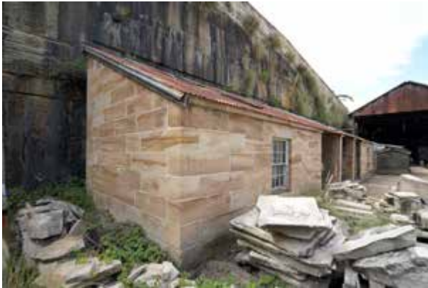
Stores building, north and west elevations
