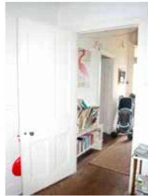
Typical internal 4-panel timber door
