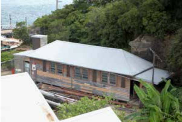
Timber store south elevation from above
