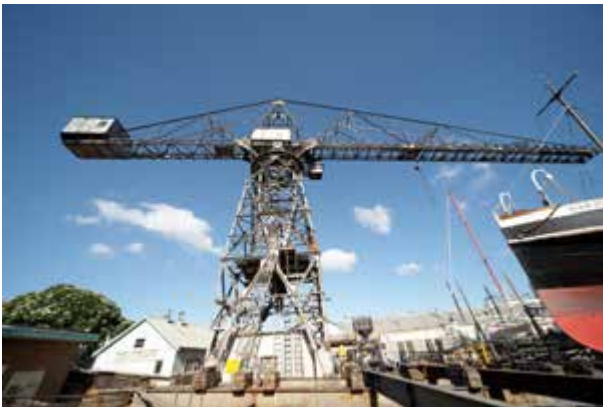
Close view of hammerhead crane
