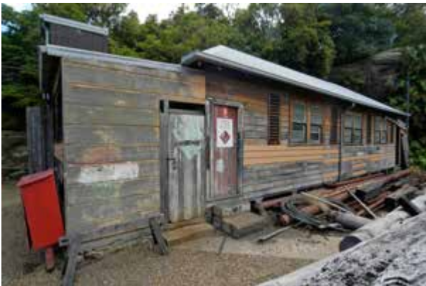
Timber store south elevation from west
