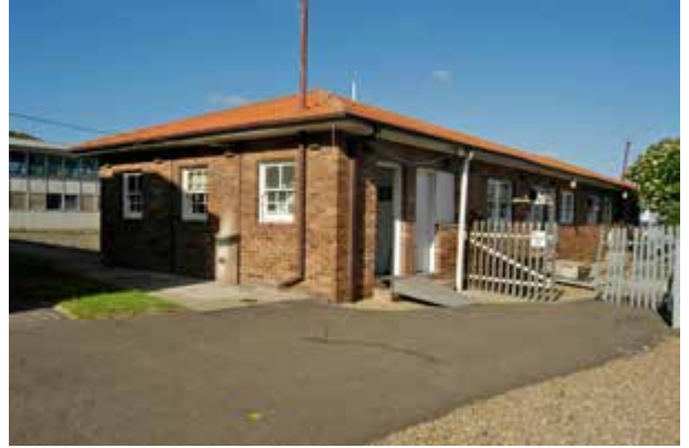
1948 Amenities building, east and north elevations
