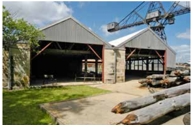
North elevation, Colonial Magazine, western and central bay
