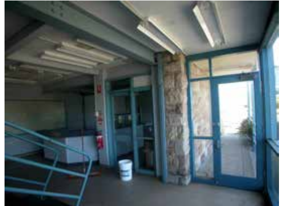
Ground floor interior, Port Emergency Services Building
