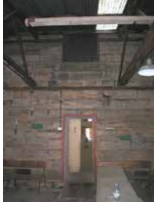
Doorway and door to southern elevation, from interior of southern addition to the Queen's Magazine. Note copper screen to southern window opening intact above the doorway.
