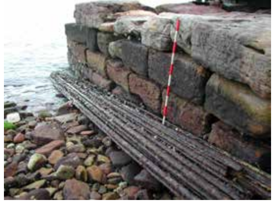
Detail, southern wall of stone jetty
