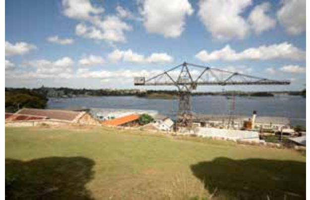
Distant view of hammerhead crane from the east
