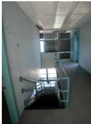
Stairwell, Port Emergency Services Building
