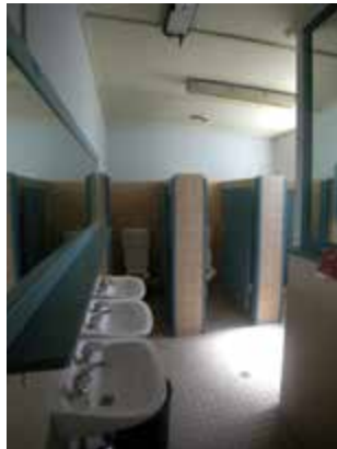
First floor bathroom with later fitout, Port Emergency Services Building
