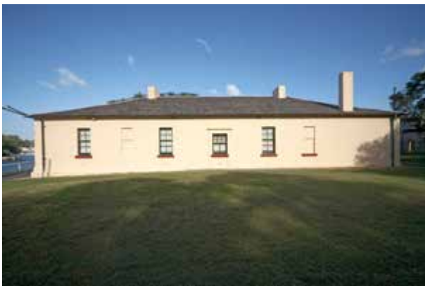
East elevation, Barracks
