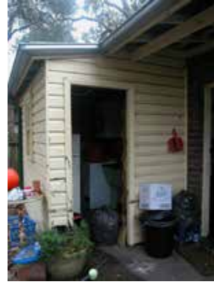
Southern elevation of weatherboard laundry
