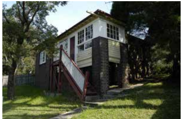
Detail, front and north elevations, Residential Cottage No. 4
