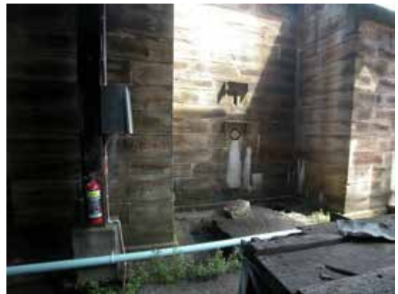
Detail, east elevation, Queen's Magazine, from within Scow Shed
