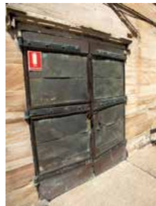
Copper-sheathed entry doors, north elevation, Queen's Magazine
