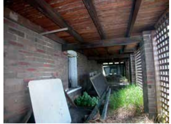
Detail, undercroft area beneath front verandah
