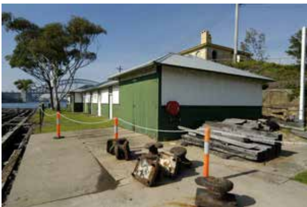
Gear Shed north and west elevations
