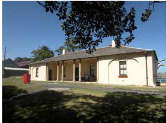
Detail, west elevation, Barracks
