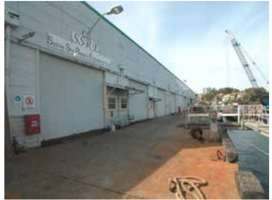
West elevation, looking south
