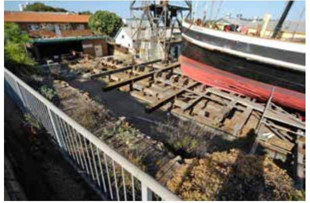
150 ton slipway in use. Repair workshop on left.
