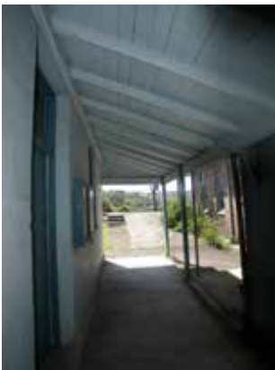
View along north verandah of Cottage
