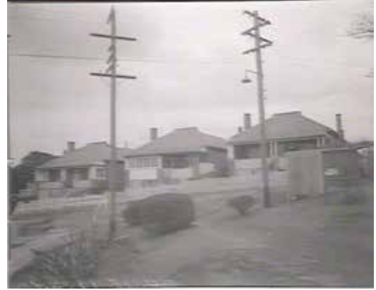
1968 photo of the three 1916 Residential Cottages (State Library image d1_10061). Residential Cottage No. 3 at left.
