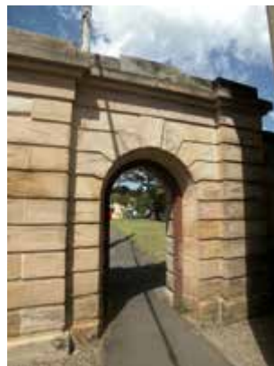
Entry arch from northern side
