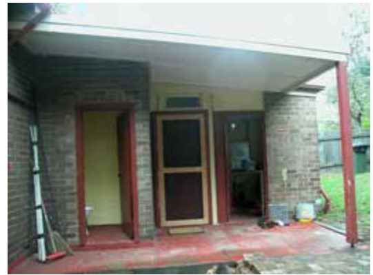
Detail, north elevation of rear brick wing
