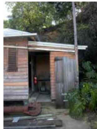
Timber store, detail of skillion section at east end
