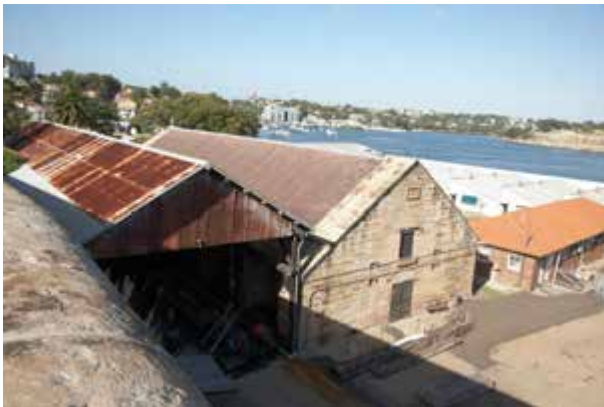
Scow Shed and Queen's Magazine from above, to east
