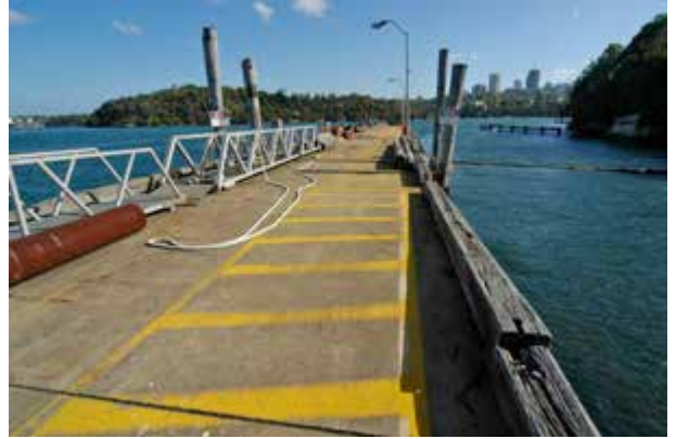
View of concrete decking on northern end of Broadside Wharf
