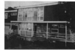
Figure No. 4. Photograph of the east elevation of the 1963 Fire Brigade Barracks prior to the major alterations to the building made in the early 1990s. (MSB Drawing No. C2081)
