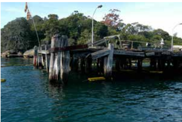
Detail of Coal Bunker platform from the west
