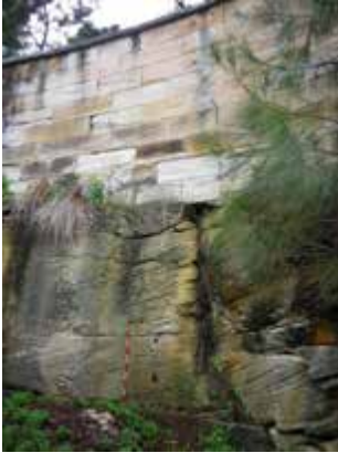
Magazine Quarry face and dressed stone wall above
