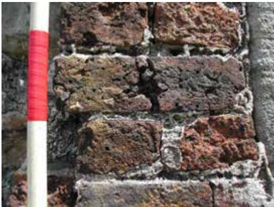
Detail, lime kiln
