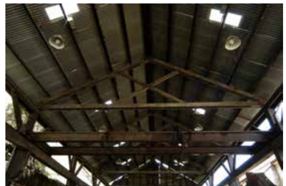
Scow Shed interior, detail of roof truss system
