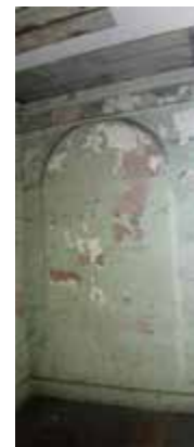
Interior, blocked up doorway to west elevation
