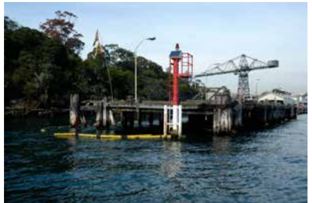
Coal Bunker platform from the north
