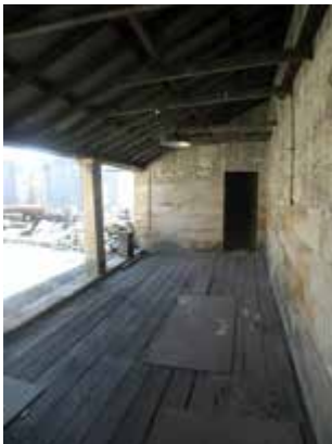
Stores building loggia, showing wide boards
