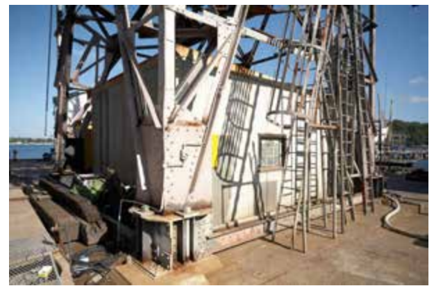
Detail, base of Hammerhead crane
