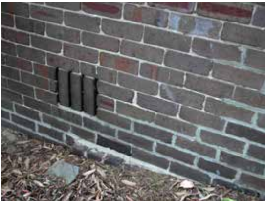
Detail, vent to footing
