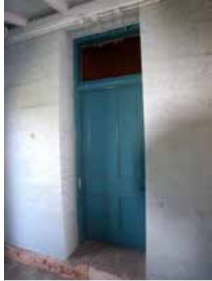
Cottage entry door (closed)
