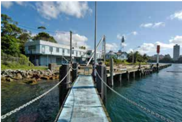
Port Emergency Services Building from Wharf Mooring Floating Plant
