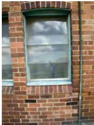
Fire Brigade Barracks, detail of altered window to north elevation
