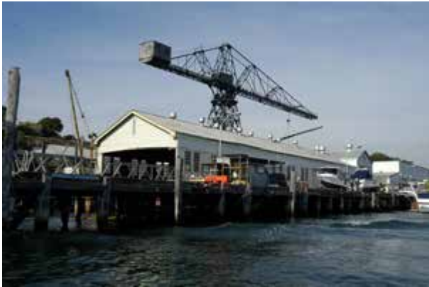
Slipway Workshop building in foreground, north and west elevations
