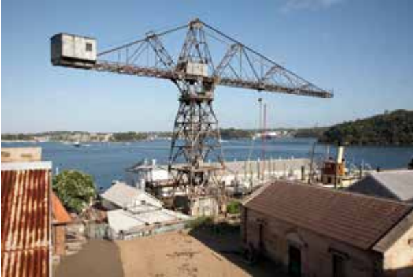
Hammerhead crane from the east
