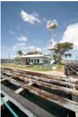
Dredge office from east
