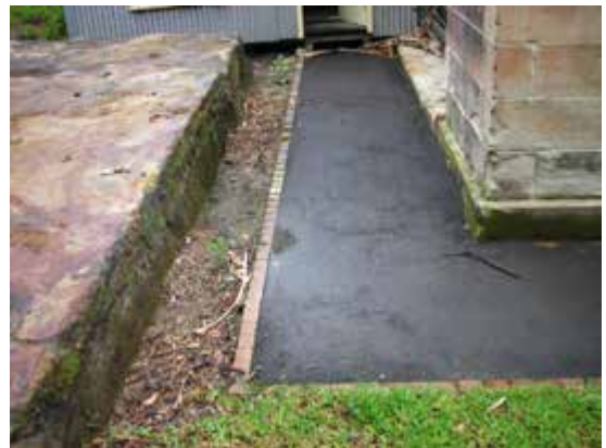
Detail of quarrying evidence near Stores Building (20)
