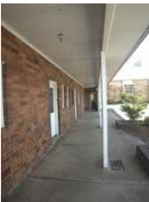
Detail of loggia, 1948 Amenities building
