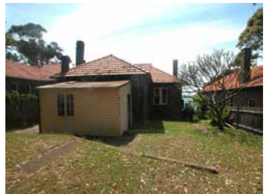
Rear elevation and south elevation from west, Residential Cottage No. 2, showing later rear weatherboard addition
