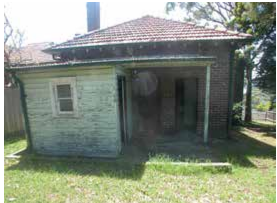
Rear (west) elevation, Residential Cottage No. 3
