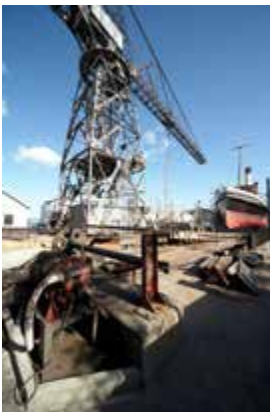
Base of Hammerhead crane
