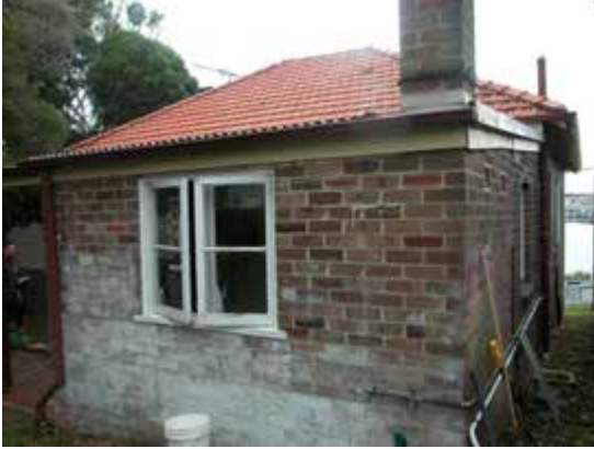
Detail, brick rear laundry extension
