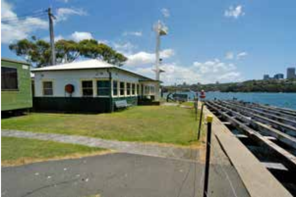
Dredge office, south and east elevations. Demountable (59) visible to left.
