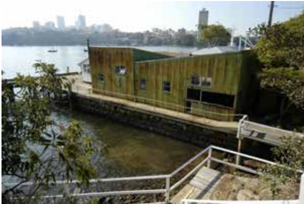
Firefighting building, west elevation
