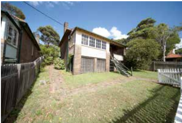
Residential Cottage No. 2, east elevation. Note partially enclosed front verandah
