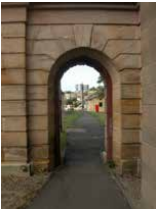
View south through the gateway in the Fortified wall
