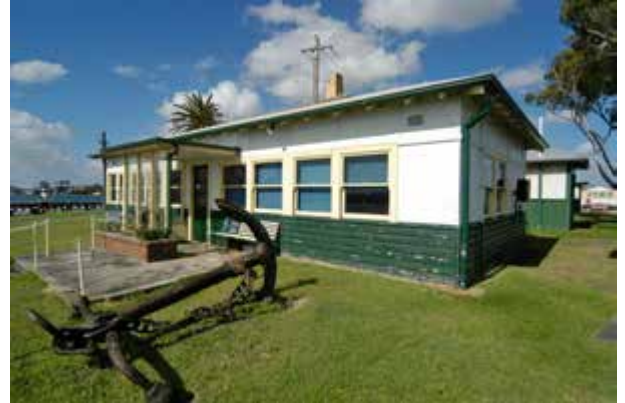
Dredge office, east elevation. Gear Shed (49) visible in background on right.
