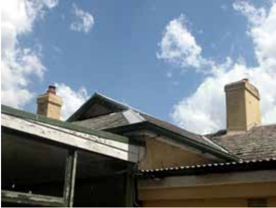
Roof and chimney detail, Kitchen cottage
