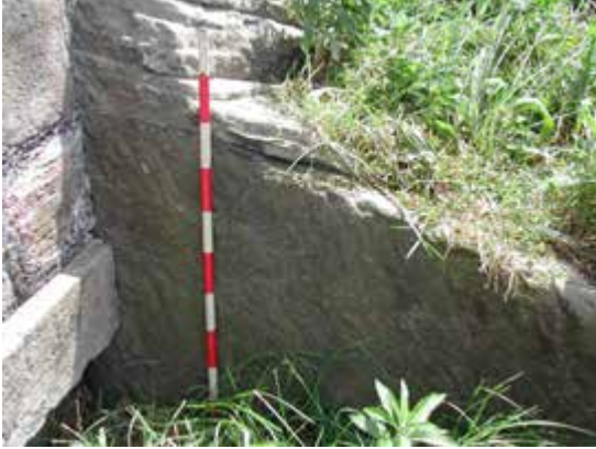
Detail, lime kiln
