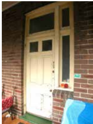
Detail of front door, fanlights, sidelight
