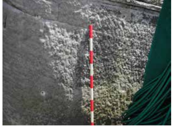
Detail, lime kiln
