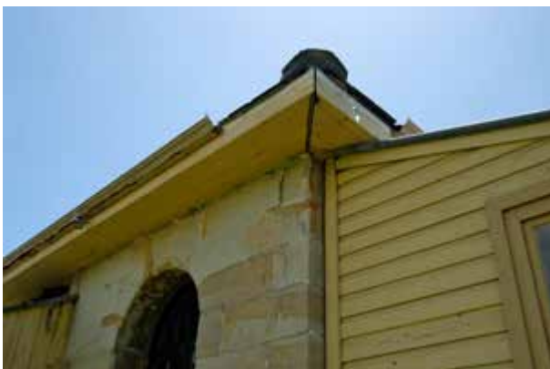
Water Police Station, detail of eaves
