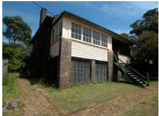
Front (east) and part of south elevation from the east, Residential Cottage No. 2
