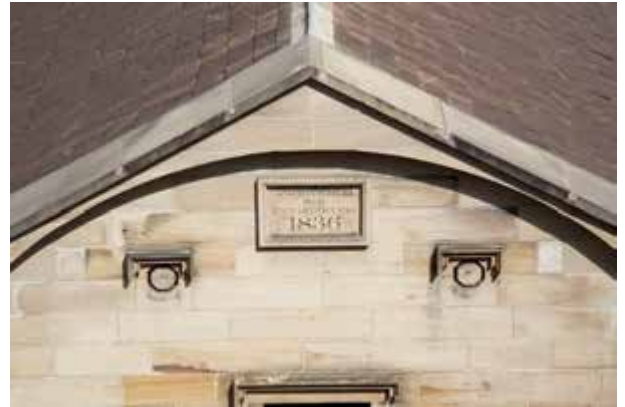
Detail of Cooperage east elevation, showing date plaque
