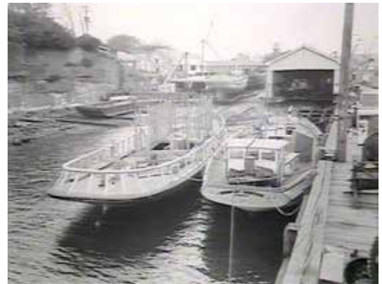
1953 photo, prior to construction of 500 ton slipway (which now occupies the area on the left of this photo). State Library image no. d1_10050.
