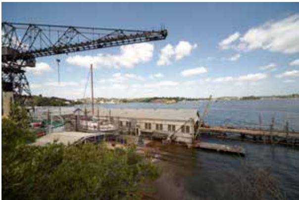
Roof of Slipway Workshop building visible at rear on right. Roof connects to roof of Repair Workshop (2)
