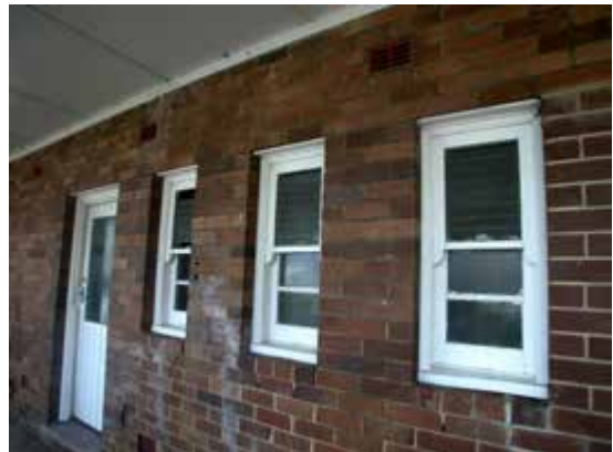
Window detail to loggia, 1948 Amenities building
