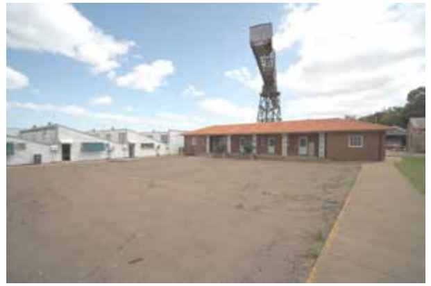
South elevation 1948 Amenities building. Ship Repair Workshop to left.
