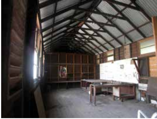
Timber store interior
