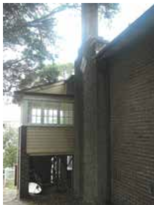
Detail, east end of north elevation, showing roughcast stuccoed chimney and verandah extending north of the remainder of this elevation
