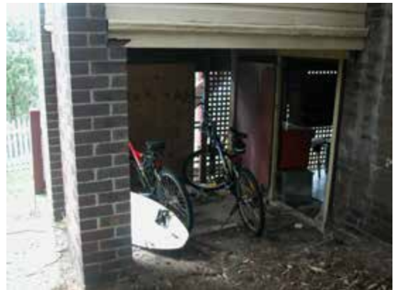
Detail, undercroft beneath front verandah
