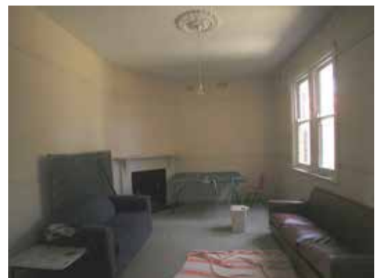
Interior, living area. Note ceiling rose and corner fireplace.
