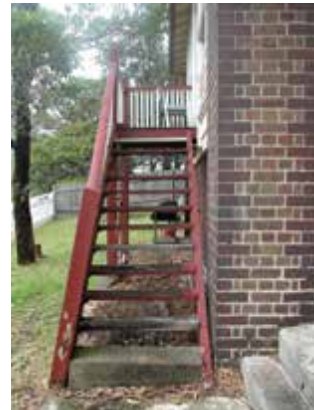
Detail, front stair from north, Residential Cottage No. 4
