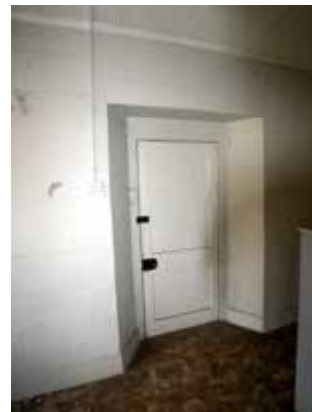
Kitchen cottage interior - Early opening into kitchen area (altered from a window)
