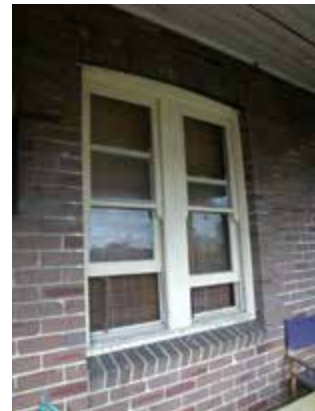
Detail of front windows to east elevation
