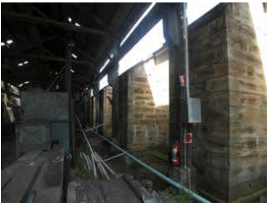
East elevation, Queen's Magazine, from within the Scow Shed
