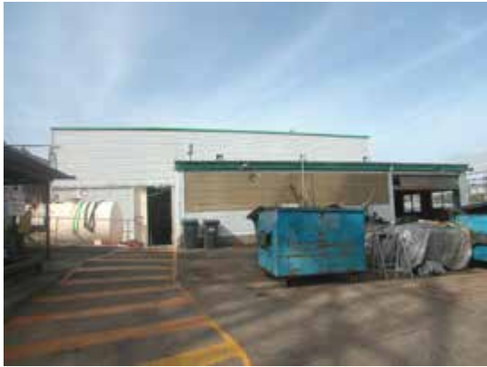
North elevation, with addition in foreground
