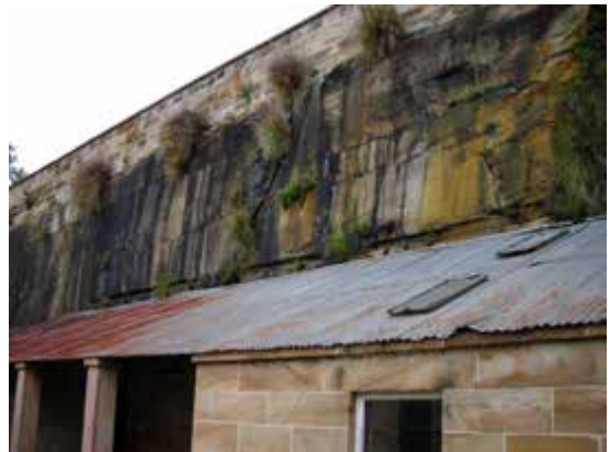
Magazine Quarry face with dressed stone wall above, behind Stores Building (20)
