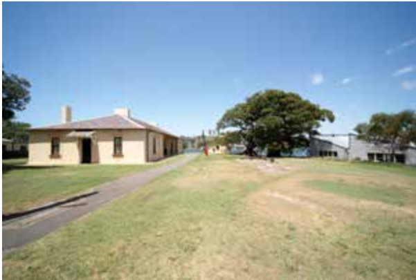
North elevation, Barracks, showing setting with Transformer house and Ship Repair Workshop to west (right)
