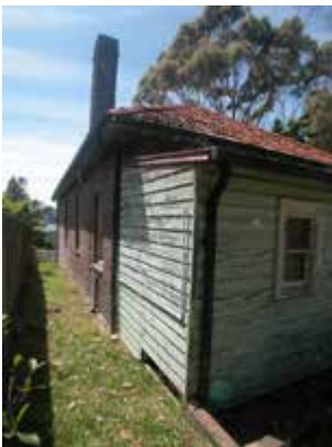
North elevation from the west, Residential Cottage No. 3
