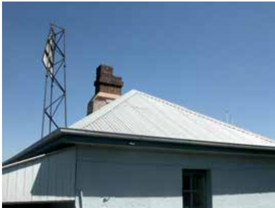
Roof and chimney detail
