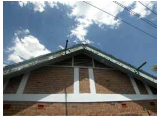
Detail, gable end, west elevation, Fire Brigade Barracks
