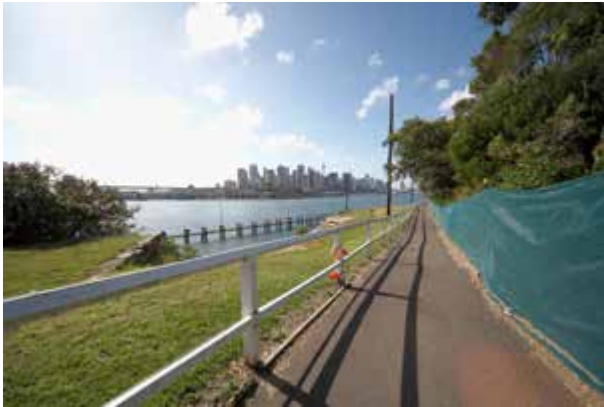
Wharf Mooring Floating Plant from Magazine Walk
