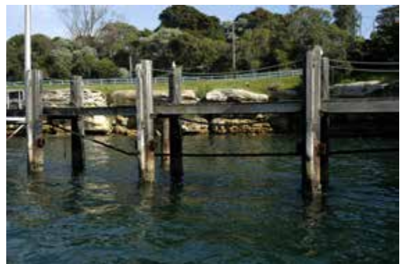
Detail, Wharf mooring floating plant
