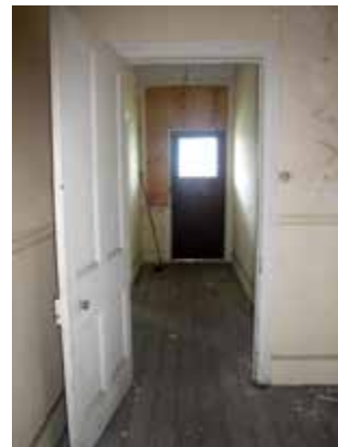
View towards front door, Residential Cottage No. 3. Note modern flush front door, plywood over fanlights, sidelight
