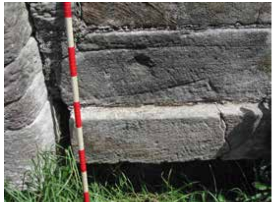
Detail, lime kiln
