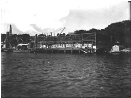
c. 1948-49 photo of Ship Repair Workshop under construction (from MSB Archives)
