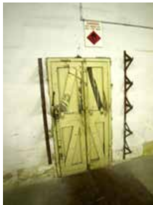
Doorway and doors to southern end, interior of Queen's Magazine
