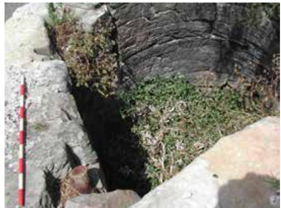
Detail, lime kiln
