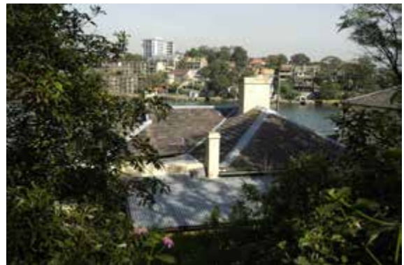
Roof detail, Kitchen cottage
