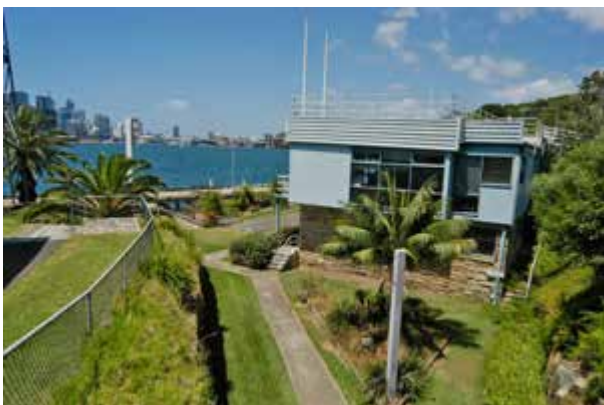
North elevation, Port Emergency Services Building
