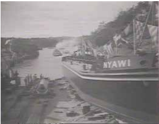
1955 photo showing coal bunkers in background at left (State Library image GPO 1 - 10060, GPO original locations or series - MSBL952)
