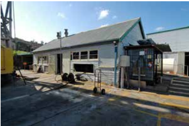
150 ton slipway winch house
