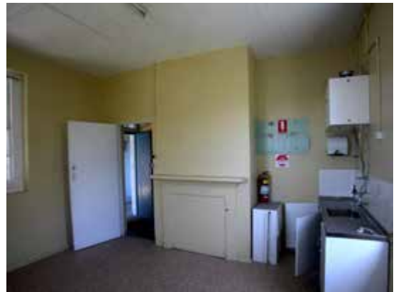
Northern room of cottage, later entry door with entry vestibule visible through it, original hearth, later kitchen fitout
