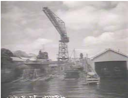
1966 photo with all slipways in use. Hammerhead crane also in place by this stage. State Library image no. d1_10058).
