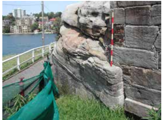
Detail, lime kiln
