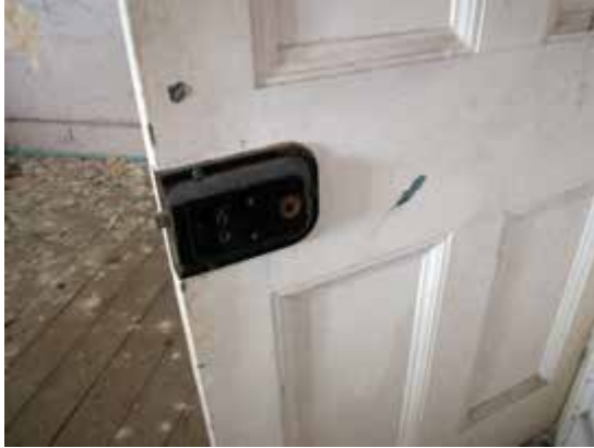
Typical internal timber 4 panel door with original door furniture, Residential Cottage No. 3
