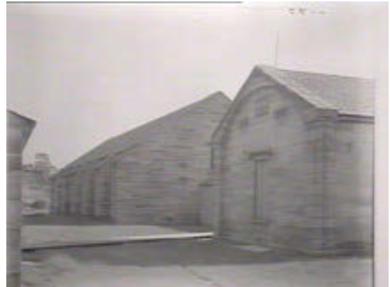
1918 photo showing east elevation of the Cooperage. Timber shutters are visible in the northern window opening (State Library image d1_13441)
