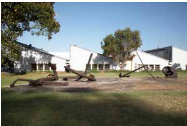
East elevation, from area in front of Barracks (25)
