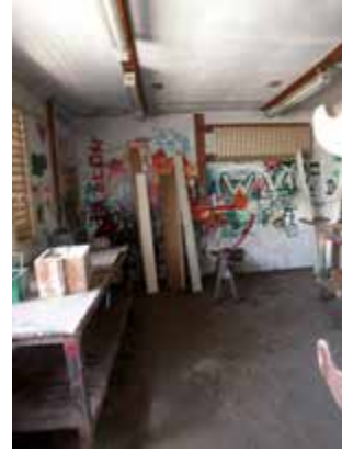
Interior, Timber store, room at western end
