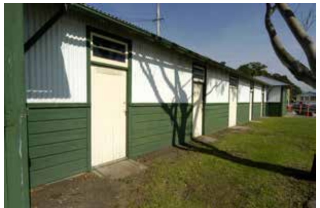
Gear Shed north elevations. Each door is labelled with the use of the room eg. "Launch room" in foreground, left.
