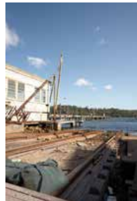
150 ton slipway looking north. Repair workshop on left.
