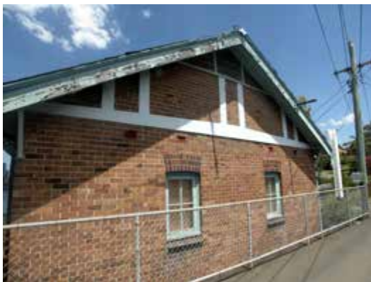
Detail, west elevation, Fire Brigade Barracks
