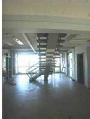
Open tread stair, Port Emergency Services Building
