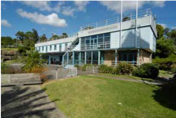
East elevation from north, Port Emergency Services Building
