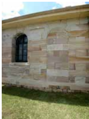
Water Police Station, blocked up doorway to west elevation
