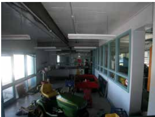
Ground floor interior, Port Emergency Services Building
