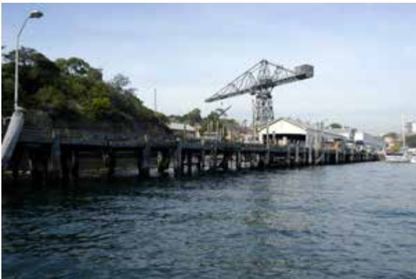
Northern end of Broadside wharf, view from northwest.
