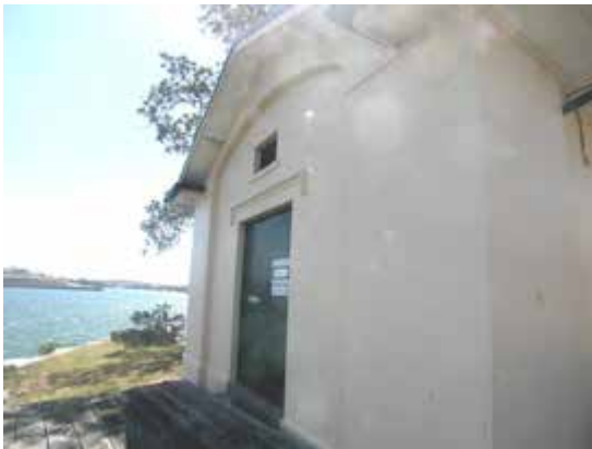
Transformer house, south elevation, facing the harbour
