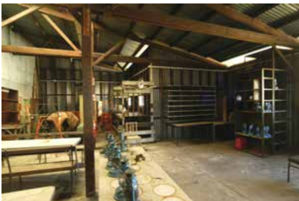
Interior, east end of Southern addition to Queen's Magazine
