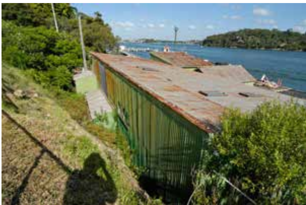
South elevation and roof of Firefighting building from above
