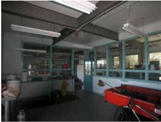
Interior, ground floor, Port Emergency Services Building
