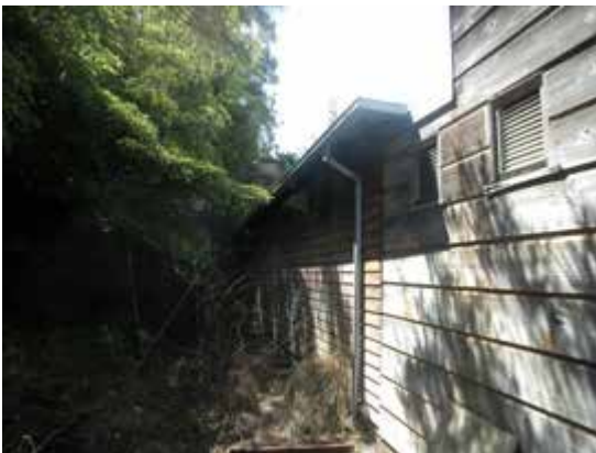
Timber store north elevation
