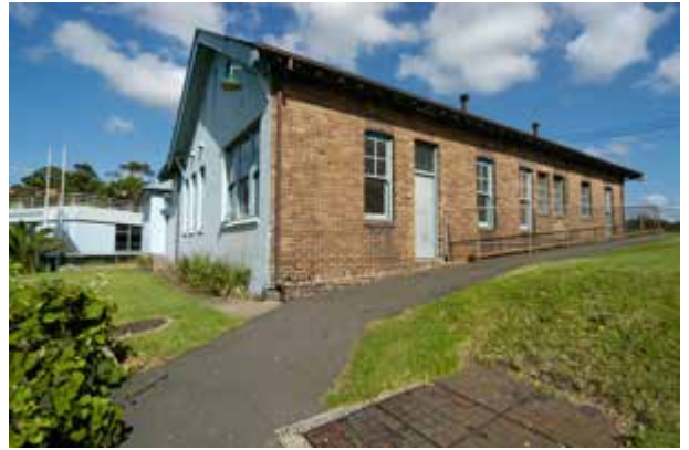
Fire Brigade Barracks, east and south elevations
