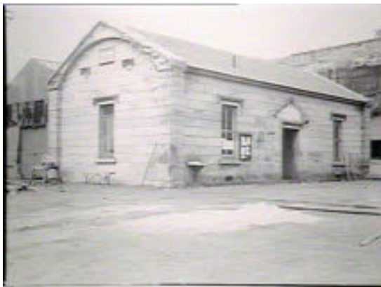
1943 photo of the west and south elevations of the Cooperage (State Library image no. GPO 1 - 10038, GPO original locations or series - MSBL965)
