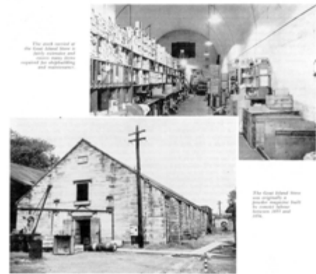
1962 images of the exterior and interior of the Queen's Magazine (images from , Port of Sydney , Official journal of the Maritime Services Board of NSW, page 27, Vol. 8, No. 1, March 1962, held at the National Maritime Museum Library)
