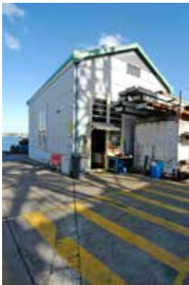
Repair Workshop extension
