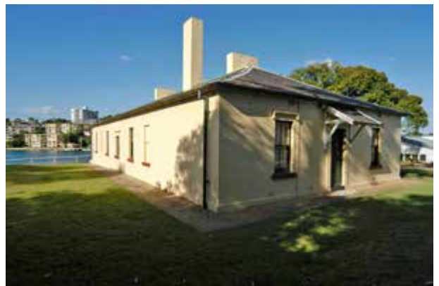
North and east elevations, Barracks
