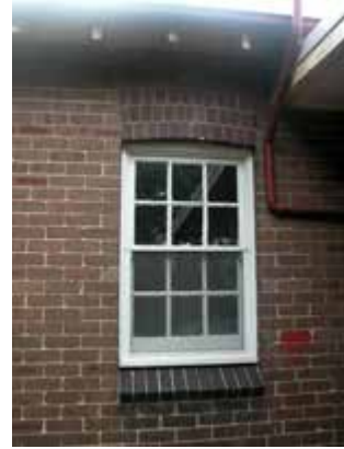
Rear window, timber-framed, double hung with 6 panes to each sash
