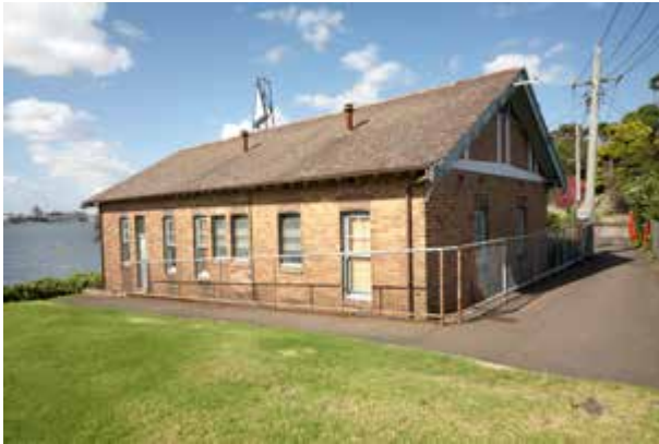
Fire Brigade Barracks, north and east elevations
