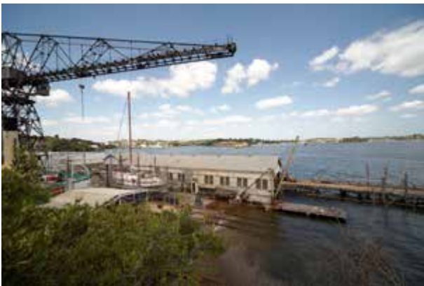
150 ton slipway from east
