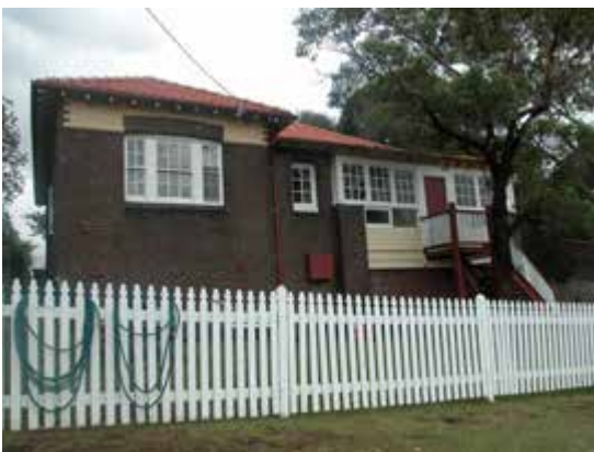
Detail front (east) elevation, Residential Cottage No. 4
