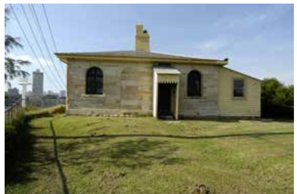
Water Police Station west elevation
