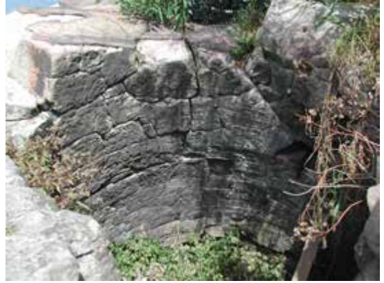
Detail, lime kiln
