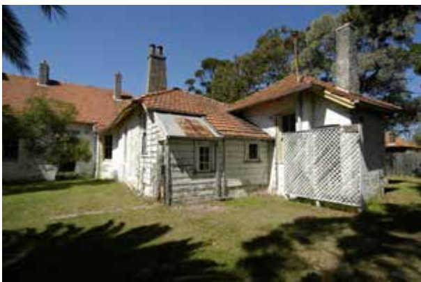
Detail, southern end of west (rear) elevation, showing weatherboard addition
