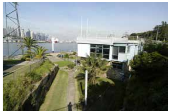
North elevation, Port Emergency Services Building, from bridge over Barney's cut. Walkway to roof deck visible on right.
