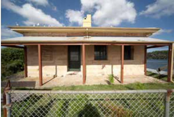
Water Police Station east elevation
