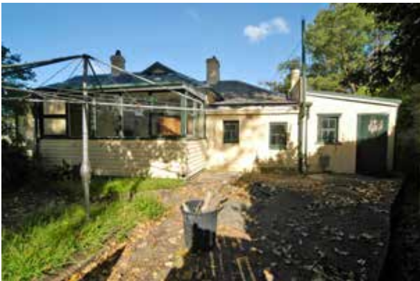
East elevation, kitchen cottage
