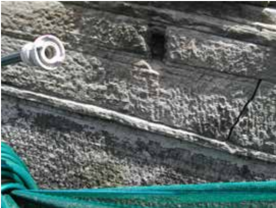
Detail, lime kiln
