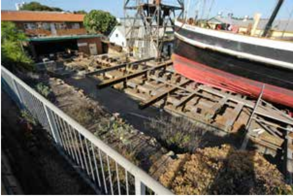
500 ton slipway from east. Winch house to left.
