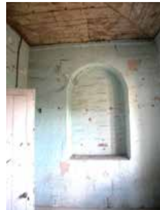
Interior, Water Police Station. Bricked up window to east elevation.
