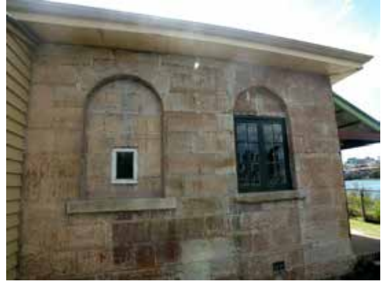
Water Police Station, eastern end of south elevation. Later windows to original police cells.
