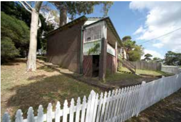
South elevation and part east (front) elevation, Residential Cottage No. 3, taken from the south
