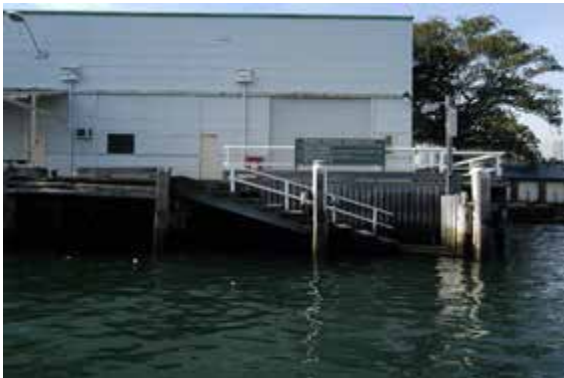
Southern end of west elevation
