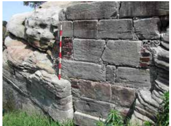
Detail, lime kiln
