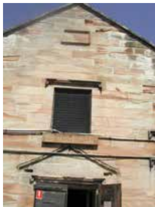
Detail, north elevation showing copper screen to window opening
