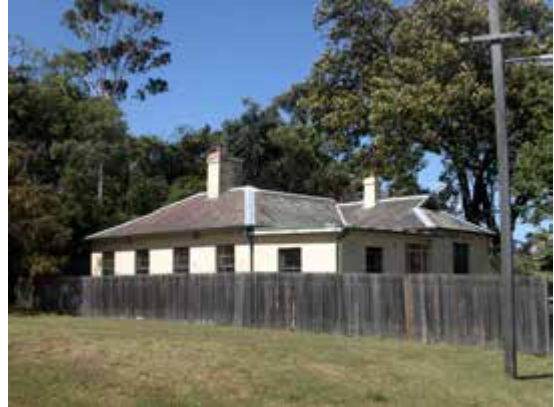
West and south elevations, Kitchen Cottage.
