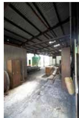
Interior, Firefighting building
