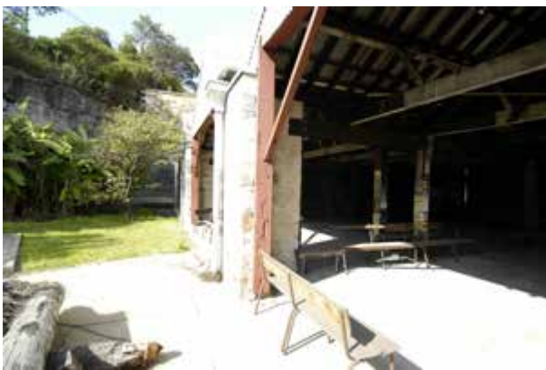
Colonial Magazine north and west elevations
