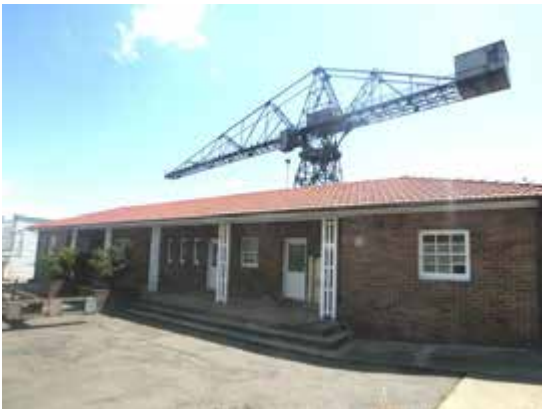
South elevation 1948 Amenities building. Note loggia with treillage posts,
