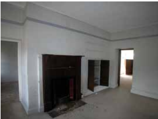
Kitchen cottage interior - Central room, Kitchen cottage. Early hearth with later chimneypeice
