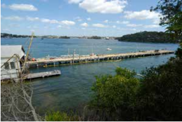
Northern end of Broadside Wharf, north of the Slipway Workshop Building (3)
