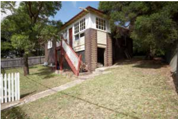
Front (east) elevation and north elevation, Residential Cottage No. 4
