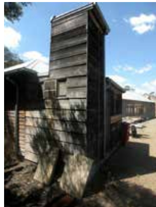
Timber store western end. The "tower" is to house a water tank for showers.
