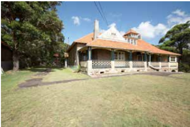
East and south elevations, Harbour Master's Residence
