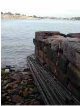
Detail, southern wall of stone jetty
