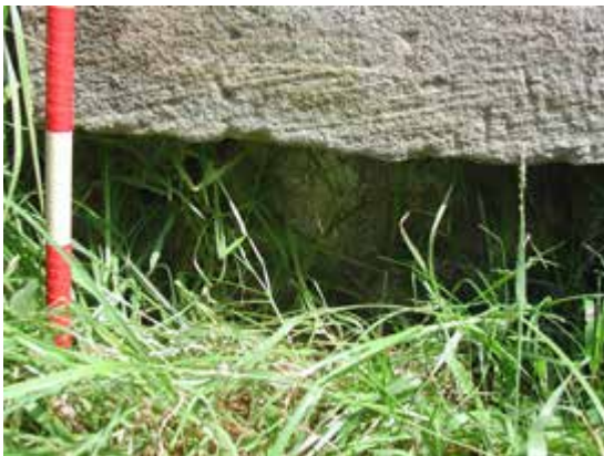
Detail, lime kiln
