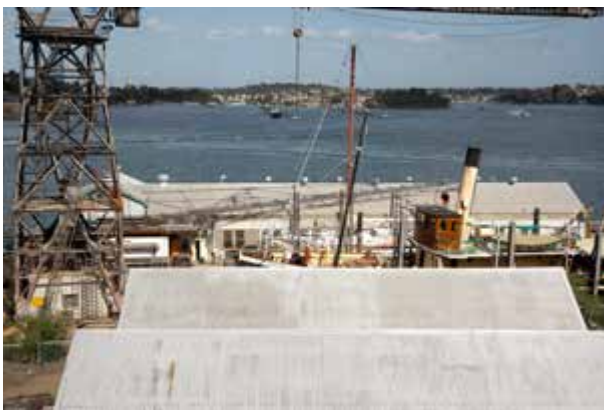
Repair Workshop Addition and Repair Workshop at left and centre, behind the hammerhead crane and slipways
