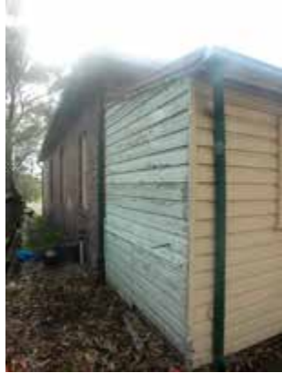
Northern elevation from rear (west) with weatherboard laundry in foreground
