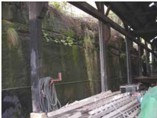
Detail, east side of Scow shed interior showing quarry face
