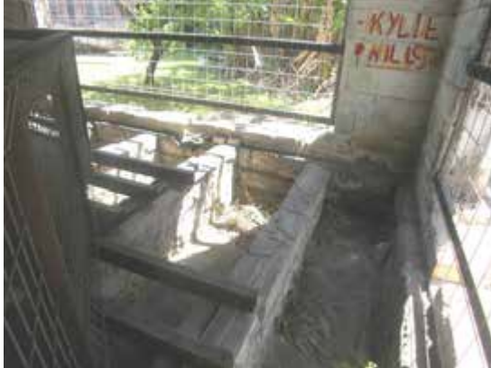
Exposed floor structure in eastern bay
