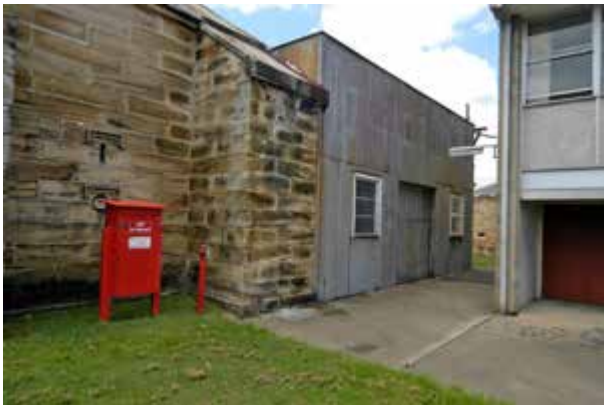
West elevation of Southern addition to Queen's Magazine. Part of west elevation of Queen's Magazine visible to left.
