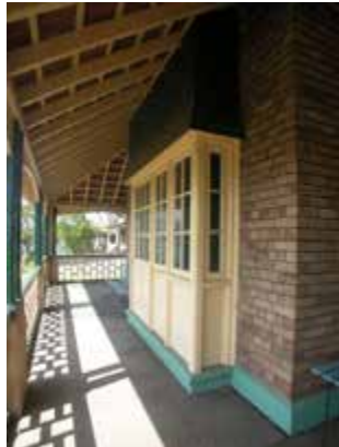
View down front verandah from north
