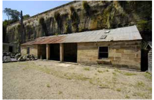
Stores building, west elevation
