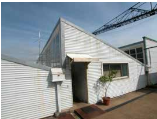
Part east elevation, from within magazine complex
