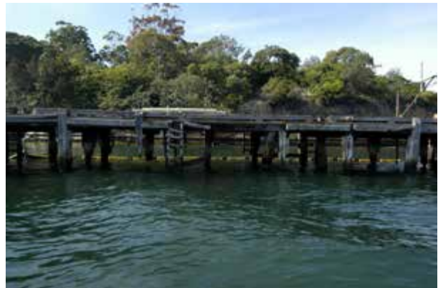
Detail, northern end of Broadside wharf
