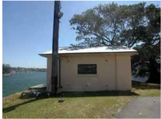
East elevation, Transformer house
