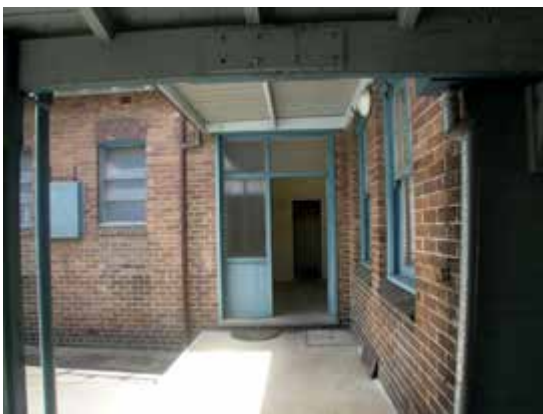
Fire Brigade Barracks, main entry door on south elevation
