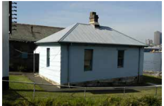
North and west elevations
