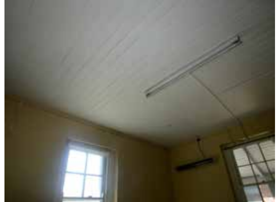
Northern room, detail of timber tongue & groove ceiling
