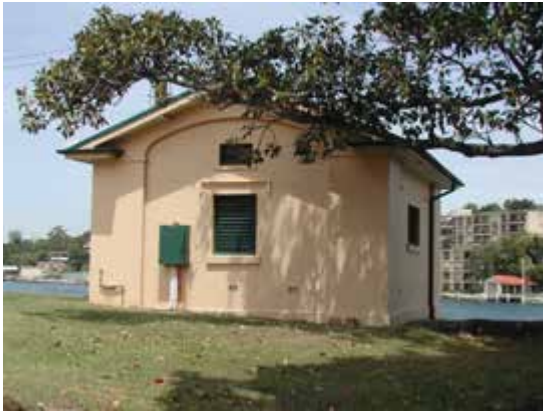
North and west elevations, Transformer house
