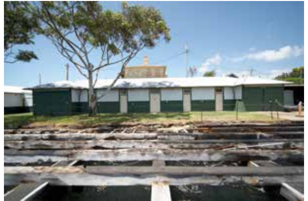
Gear Shed north elevation. Water Police Station visible above.
