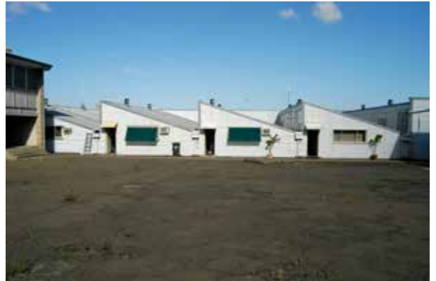
East elevation, as seen from within the magazine complex
