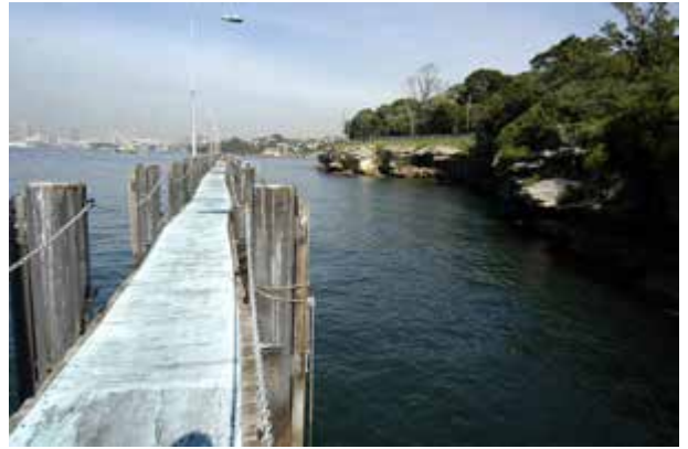
Wharf Mooring Floating plant from north looking south
