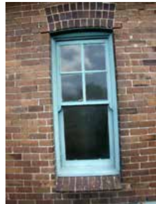
Detail, original window to north elevation, Fire Brigade Barracks
