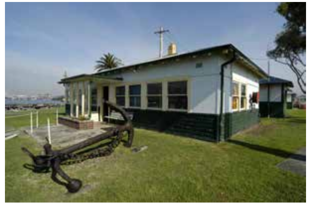
Dredge office, east and north elevations
