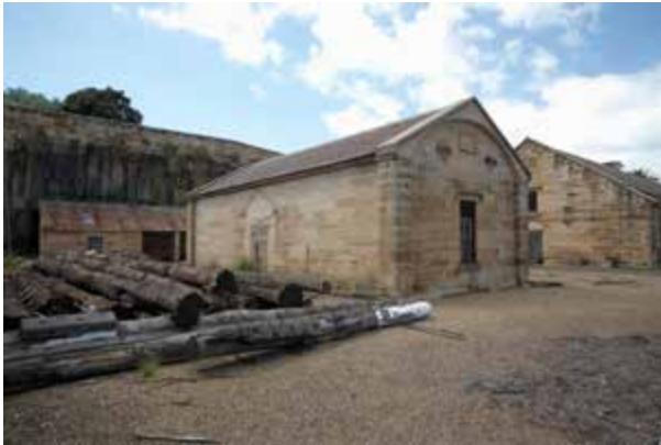
North and west elevations of the Cooperage
