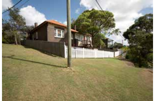
Front (east) and south elevations, Residential Cottage No. 4, with Residential Cottage No. 3 visible to north (right)
