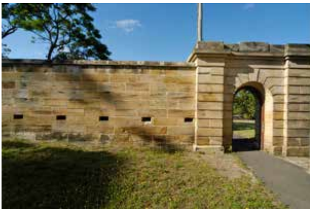
Fortified wall and entry from northern side
