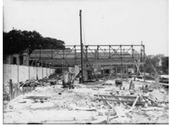
c. 1947-48 photo of Ship Repair Workshop under construction (from MSB Archives)
