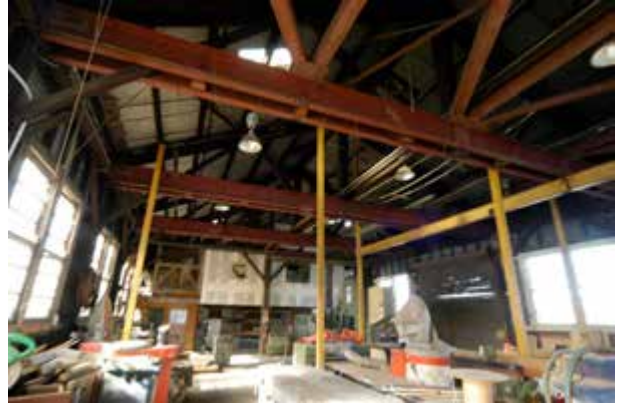
Interior, Repair Workshop and Repair Workshop extension
