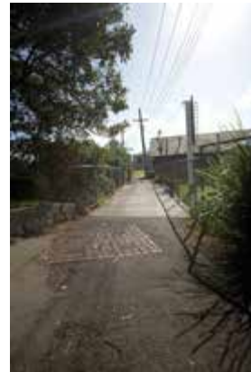
Looking across the bridge over Barney's Cut
