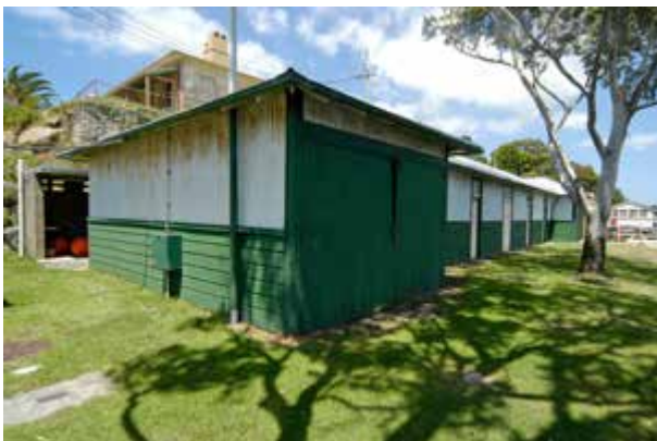
Gear Shed east and north elevations. Water Police Station visible above
