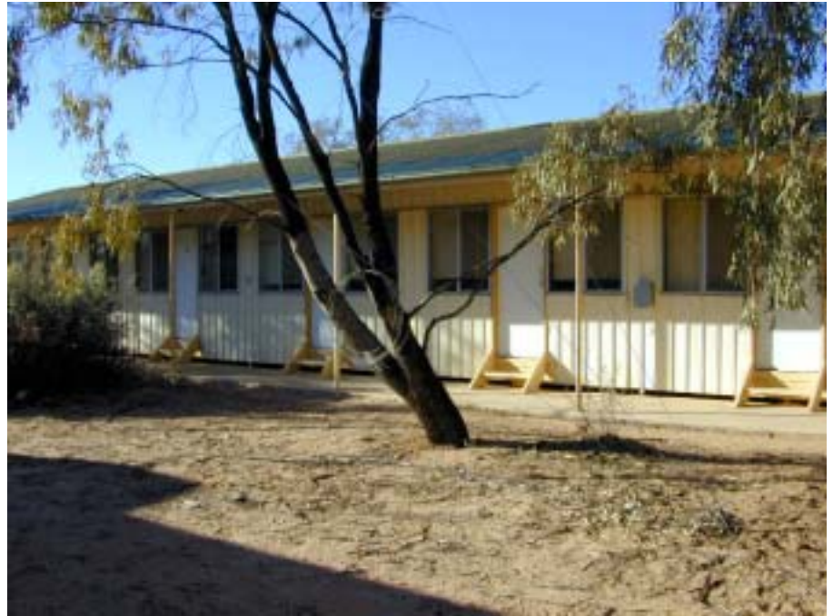
Figure 86 The c1950s shearers' quarters, north elevation. PF 2002 photograph
