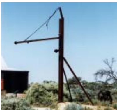
Figure 51 Crab winch and boom for loading bales of wool. PG 2001 photograph
