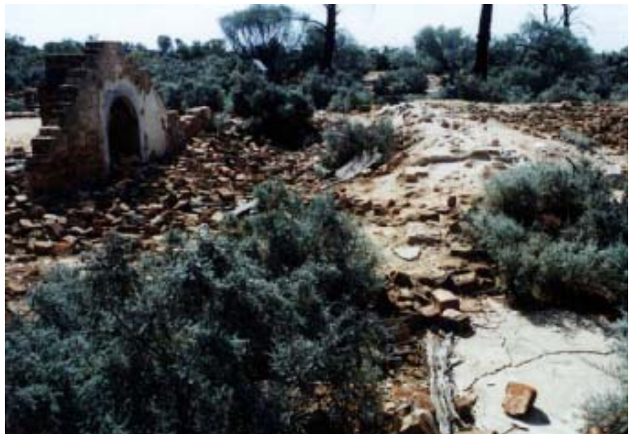
Figure 35 Homestead ruin. The most prominent structure standing is the chimney on the left. Note the trunk of the dead palm tree. The tops of the former walls have become the safest place to walk. PG 2001 photograph
