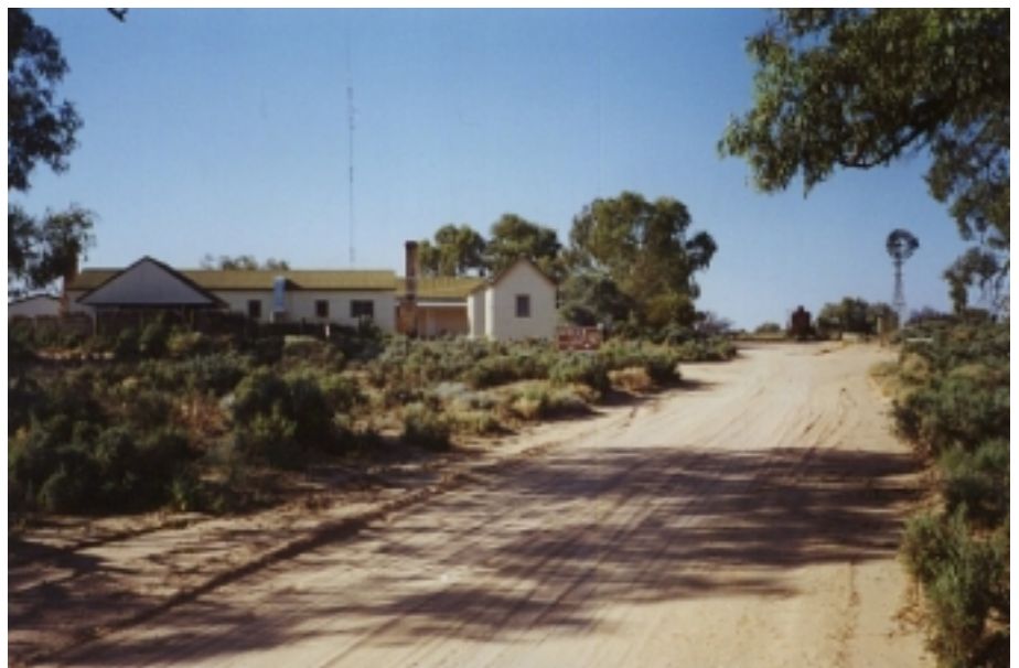
Figure 5 At the Kincheega woolshed and Shearers' Quarters; the road south and unidentified buildings [the former Shearers' Quarters]. BN 2001 photograph
