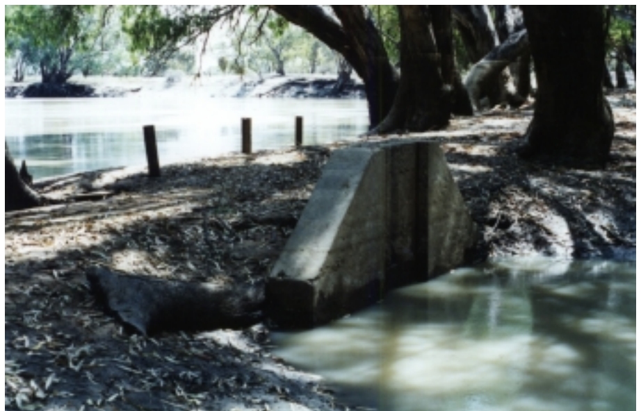
Figure 25 The Homestead Billabong Regulator. PF 2001 photograph
