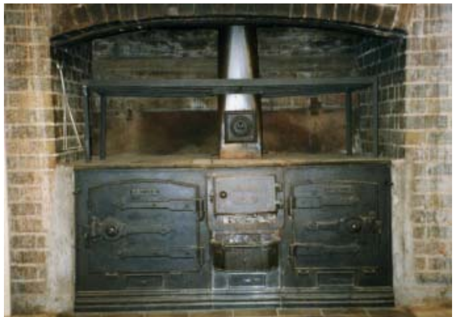
Figure 98 Cast iron stove in the kitchen area of the cookhouse. Note how the Metters door is too short for the firebox. PF 2001 photograph
