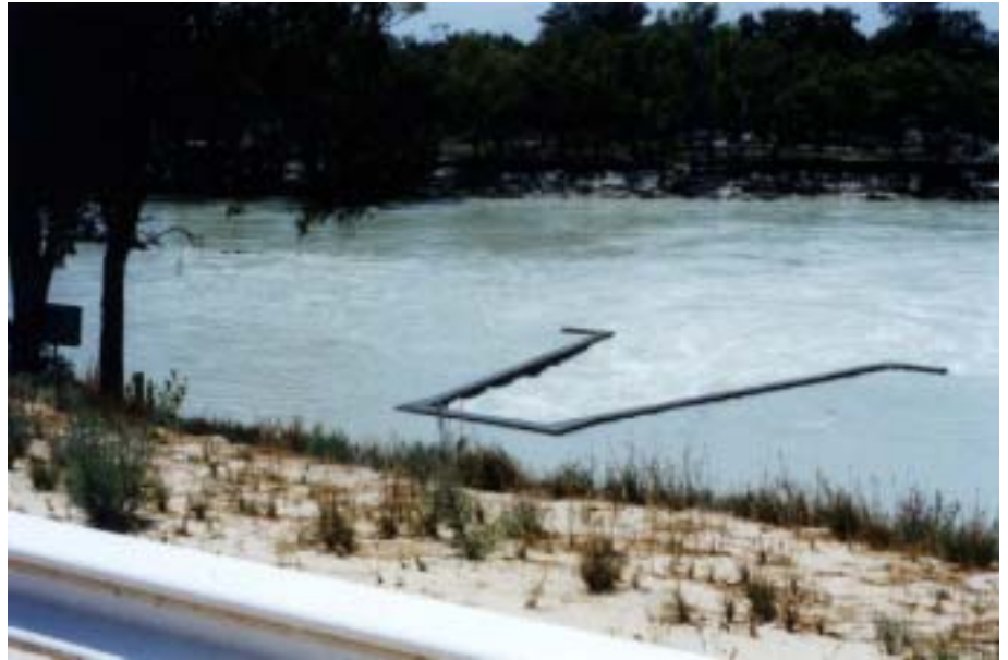
Figure 5 The Regulator at high river levels. PG 2001 photograph
