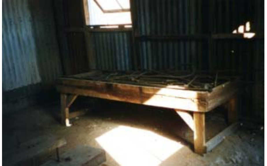
Figure 71 'Bed' in Engine Room with tools on it. AF 2001 photograph
