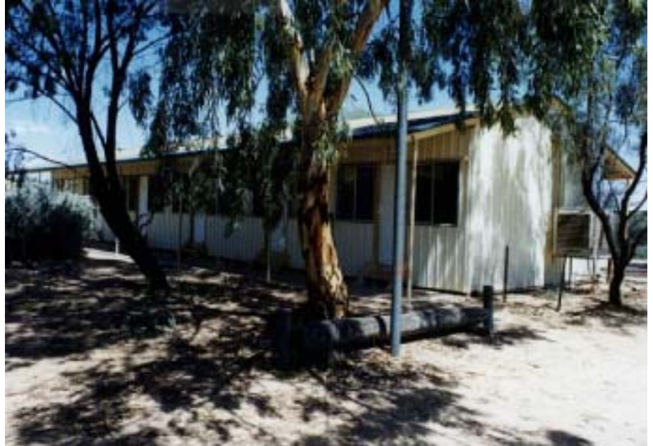
Figure 4 Recent tree planting in shearers' quarters precinct PG 2001 photograph
