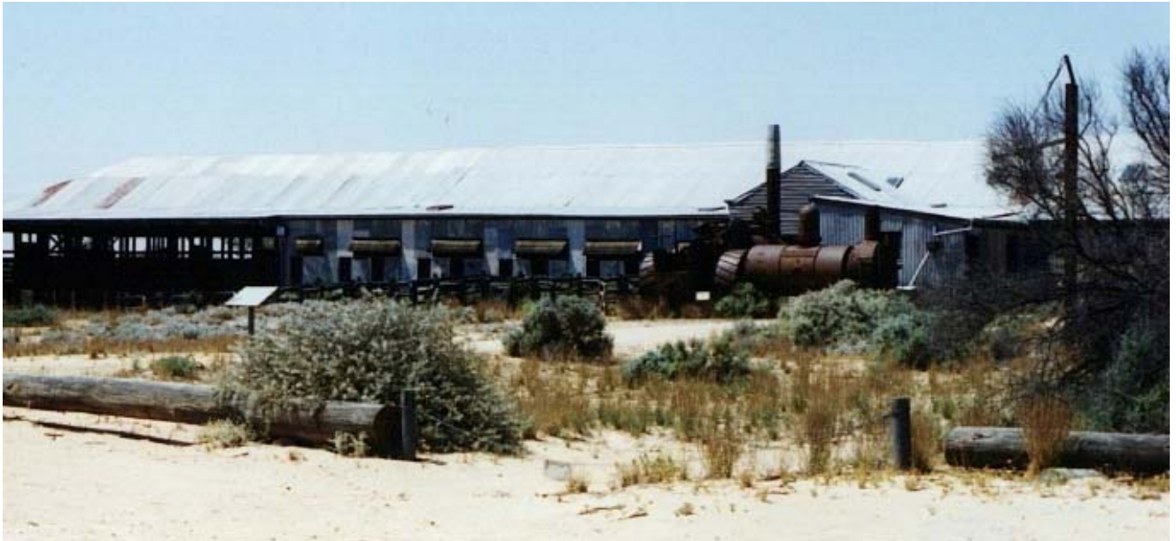
Figure 41 Locomotive boiler and old steam plough still in situ adjacent to the engine room, north elevation. During shearing time this part of the site would have been very much a rural industrial landscape. PG 2001 photograph
