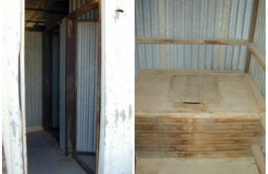
Figure 131 & 132 The 'long drop' toilet block, interior. PF 2002 photographs
