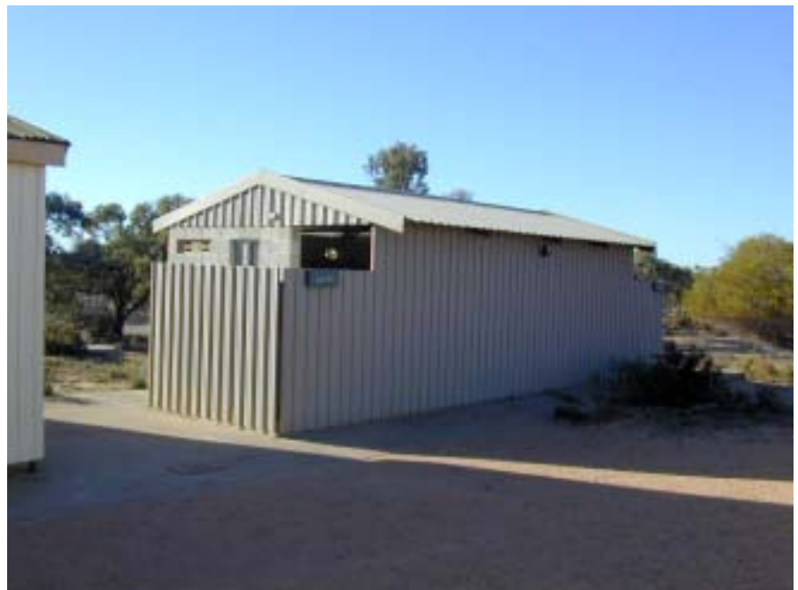
Figure 134 The modern toilet block from the north-west. PF 2002 photograph
