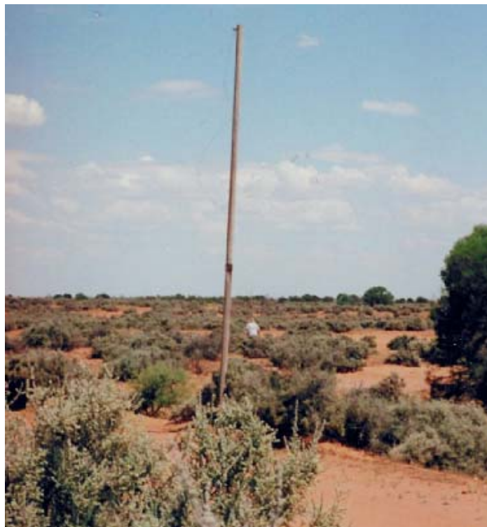
Figure 17 Telegraph pole of galvanised pipe SMT 2001 photograph
