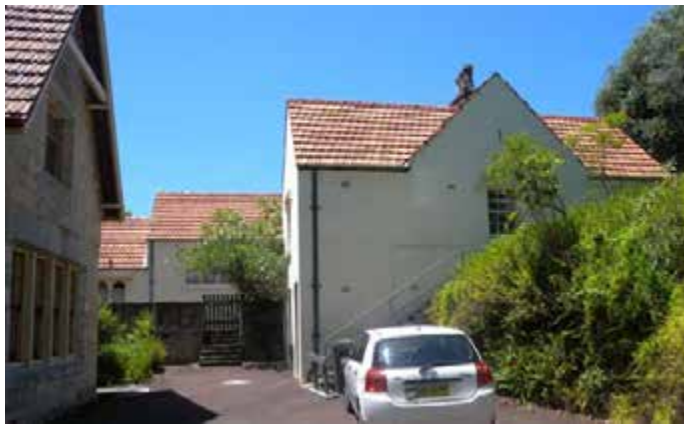
View of the west end of Margaret Harper with the west elevation of the former laundry prominent in the view and walled stone courtyard in the centre background. Source: Author October 2010.
