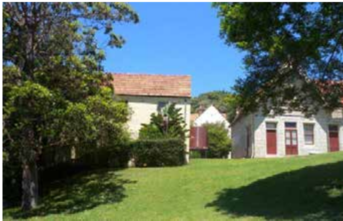
View of Margaret Harper from the north with the former sun terrace in the foreground now planted out. Source: Author October 2010.
