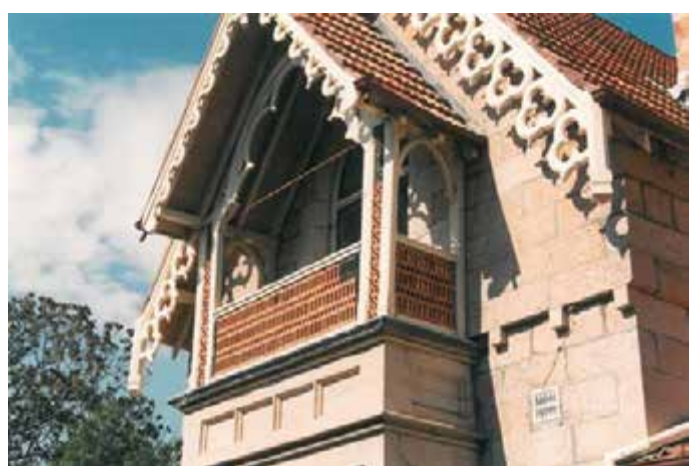
Terra cotta balustrade on upper northern balcony.
