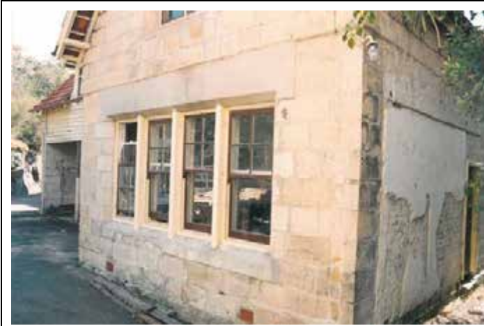
Hospital phase window alterations to stables wing.
