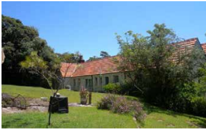
Looking north west to the south elevation and the lawn showing the 1975 opening with its sliding doors and the surviving original windows and the smaller bathroom windows. Source: Author October 2010.
