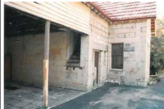
Alterations to stair and doorways in stables wing.
