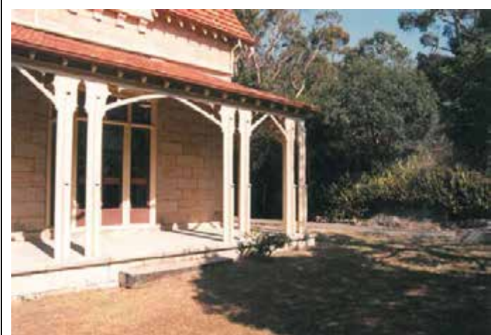
North west verandah with enclosure removed by NPWS.
