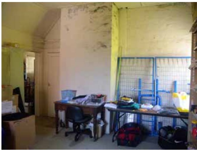
Looking south in the former Drying Room. Source: Author October 2010.
