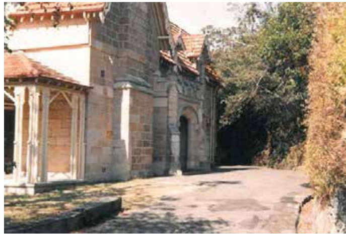
Main entry porch with medieval gothic detailing.
