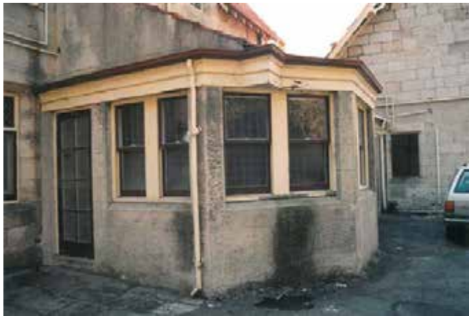
Southern room added by Tresillian Vaucluse in 1939.
