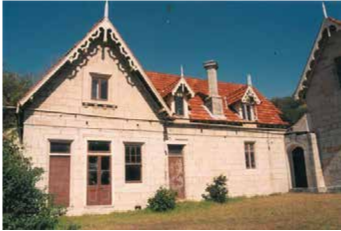
Original southern verandah linking kitchen wing.
