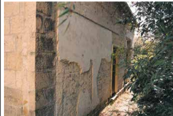
Surviving wall plaster from hospital phase verandah.
