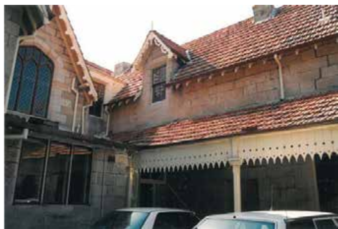
The two storey stables with terra cotta roof tiles.
