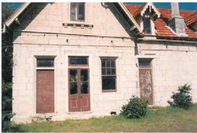
Alterations to stables for access to old verandah.
