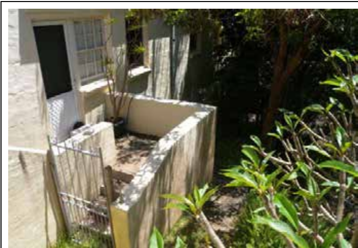
View of the dog-legged stairs leading from the 1975 terrace. Source: Author October 2010.
