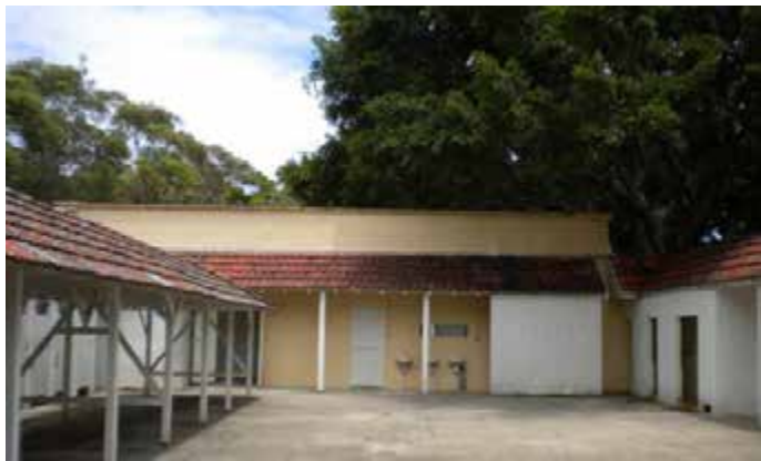
The Men's changing area looking west. Source: Author January 2011.
