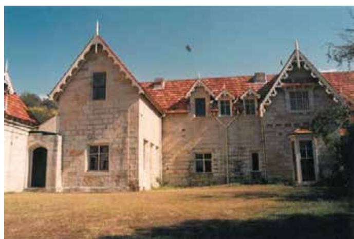
Second storey added onto the rear wing in the 1870s.
