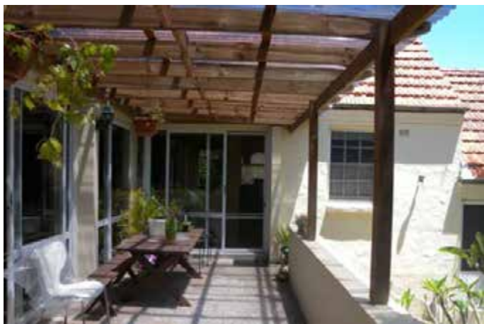
Looking west along the 1975 terrace towards the east wall of the building showing the larger openings formed in 1975. Source: Author October 2010.
