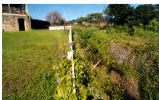
Fig 4.14 The only exposed section of the moat is that around MH29. This area is in poor condition and is substantially overgrown. PAUL DAVIES PTY LTD 2002
