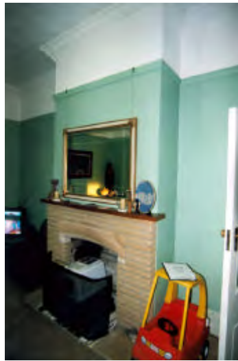
Fig MH29.19 Fireplace in 29.03. The original fire insert and surrounds have been modified to c1930s stone facing. PAUL DAVIES PTY LTD 2002
