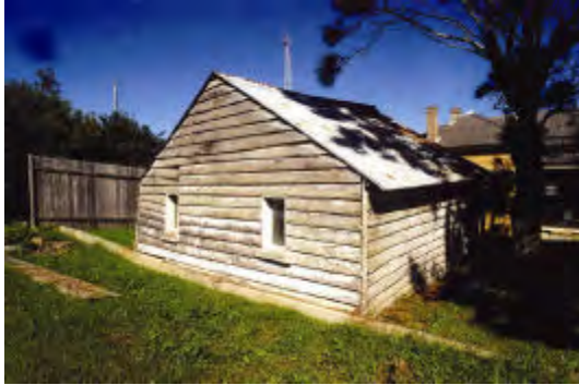
Fig MH34.2 Coal store from the north. PAUL DAVIES PTY LTD 2002
