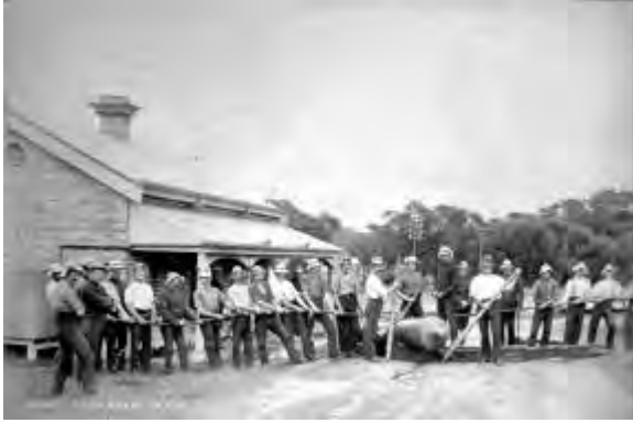
Fig MH32.7 Crew with cannon in front of Guardhouse c1892. The building is face brick, has a chimney, and in detail one can see the two thin windows in the wall under the verandah. NPWS Slides 1892
