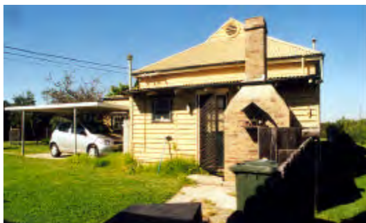
Fig MH31.6 View along what was battery road showing fence line and chimney structure. . PAUL DAVIES PTY LTD 2002
