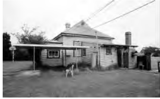
Fig MH31.3 Further view from north showing carport and kitchen addition with chimney. Note open vent to roof. PAUL DAVIES PTY LTD 2002
