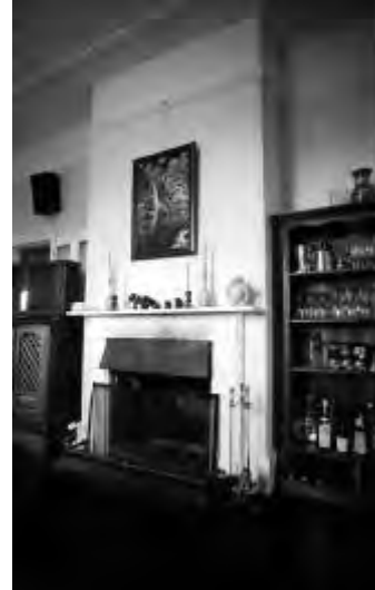
Fig MH29.15 A rendered chimney with white marble fireplace surrounds. Note later picture rail and ceiling with timber trims. PAUL DAVIES PTY LTD 2002
