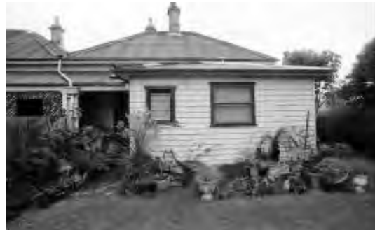
Fig MH29.9 In contrast with the earlier kitchen addition, the later kitchen has later window openings and a flatter roof pitch. The left window appears a remnant from its bathroom use. PAUL DAVIES PTY LTD 2002
