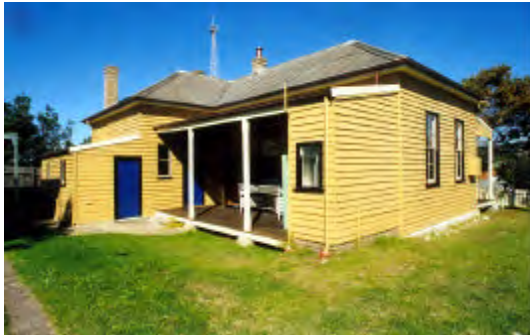
Fig MH26.4 View from north showing bathroom additions. PAUL DAVIES PTY LTD 2002
