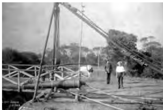
Fig 4.18 The original entry to the site was funnelled through this timber bridge. NPWS Slides
