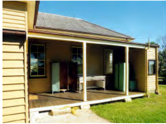
Fig MH26.3 Rear verandah. PAUL DAVIES PTY LTD 2002
