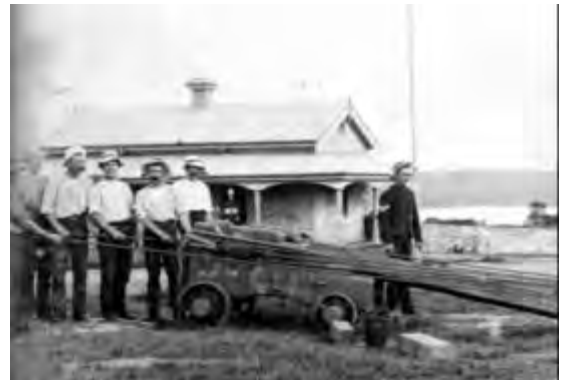
Fig MH32.10 Another oblique view showing the west window opening and extent of the verandah. The supervisor stands under the verandah. NPWS Slides 1892
