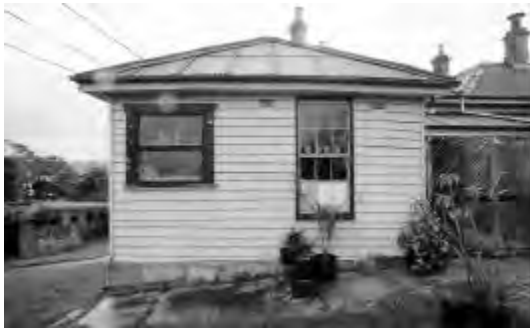
Fig MH29.8 View of southern kitchen/laundry addition showing one salvaged window and one later window. PAUL DAVIES PTY LTD 2002
