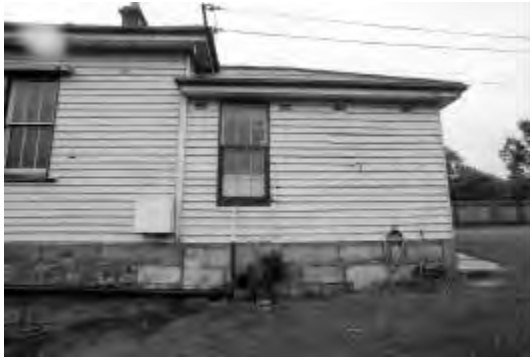
Fig MH29.6 Side view showing the southern kitchen addition. The stonework is distinct, but still of a high quality, and the window is a salvaged 12 pane original window. PAUL DAVIES PTY LTD 2002
