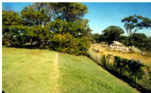
Fig 4.12 The section of the outer moat adjacent the tennis courts. This was once the site of the stables building. The moat has been infilled and built up to the head of the defensive wall, largely obscuring an important site feature and potentially endangering the wall condition. The fill used may contain sections of demolished buildings. PAUL DAVIES PTY LTD 2002
