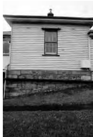
Fig MH29.5 Side view showing the 12 pane windows in a weatherboard wall on the roughly coursed stone basement wall. The eaves have been reclad, but retain the original form. PAUL DAVIES PTY LTD 2002
