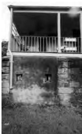
Fig MH29.11 Mass concrete infill with loopholes. PAUL DAVIES PTY LTD 2002
