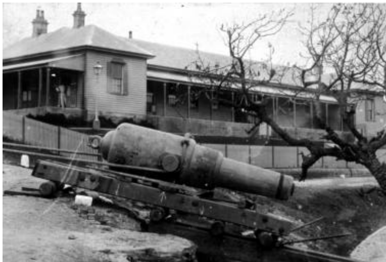
Fig 4.7 Barracks, located at South Head with a substantial similarity to MH27. This photo is the best indication of the form, materials and typology of MH27. NPWS Slides
