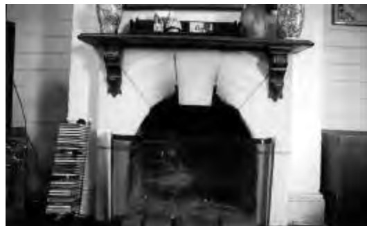
Fig MH31.18 Altered fireplace. The detailing, style and materials would date from pre-1940. PAUL DAVIES PTY LTD 2002
