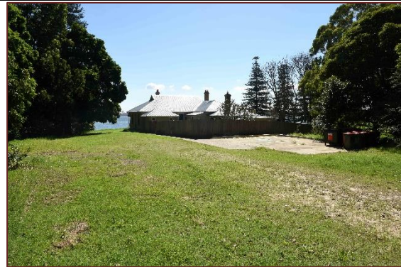
Plate 13. Looking north across the dune crest landform element that the historic complex is located on.
