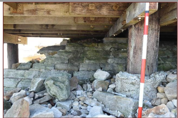
Plate 19. Sandstone sea wall beneath the modern jetty.
