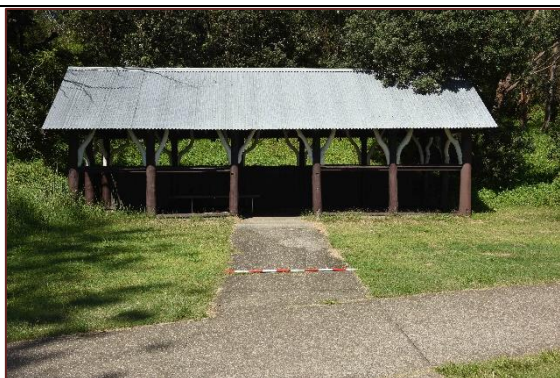
Plate 20. Concrete pathway that was constructed in 2009.
