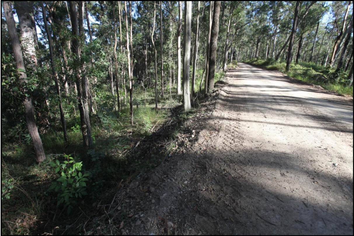
Figure 29: Wittigs Road, facing east with cut and fill road construction visible on slope.
