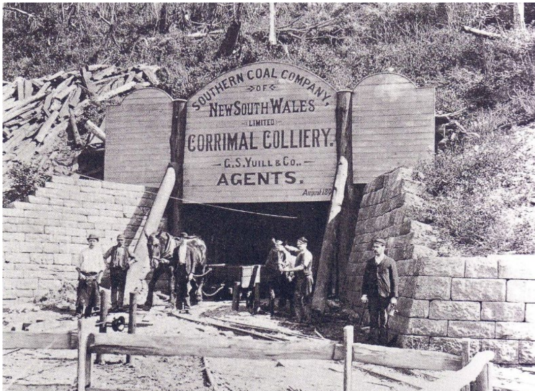
Plate 8: Corrimal Colliery pit top – Daylight Portal and adit (source: website-Illawarra Coal)
