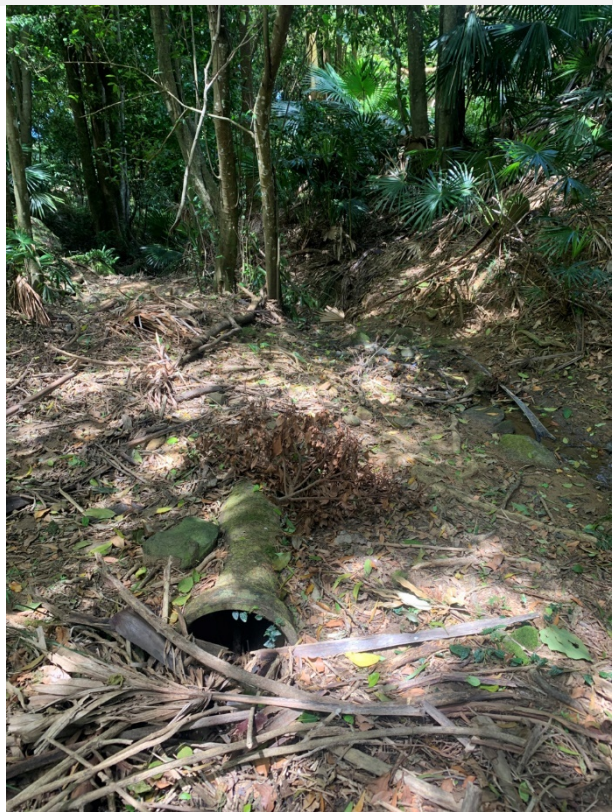
Plate 16: View of Feature 8 steel pipe used for culvert.
