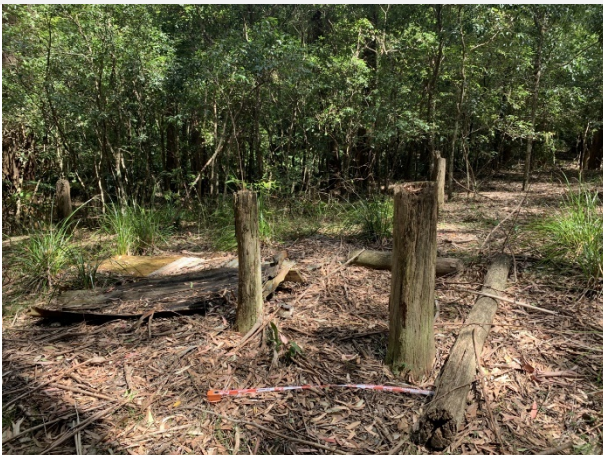
Plate 11: View of Feature 3: collapsed lean-to structure, with evidence of recent re-use as a shelter.
