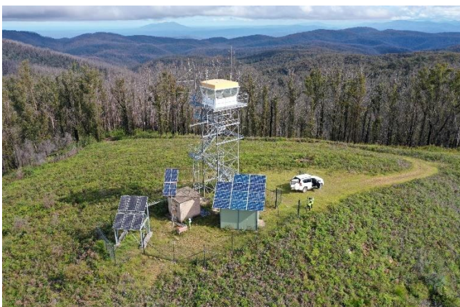
Aerial view to the existing radiocommunications facility and fire lookout tower
