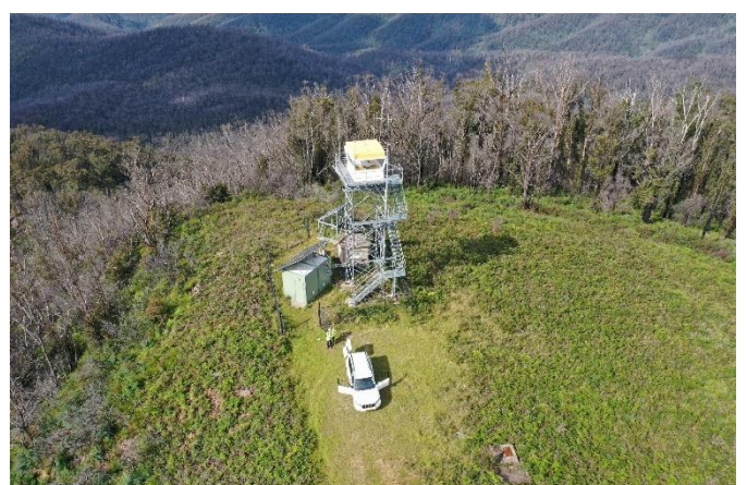
Aerial view to the existing radiocommunications facility and fire lookout tower
