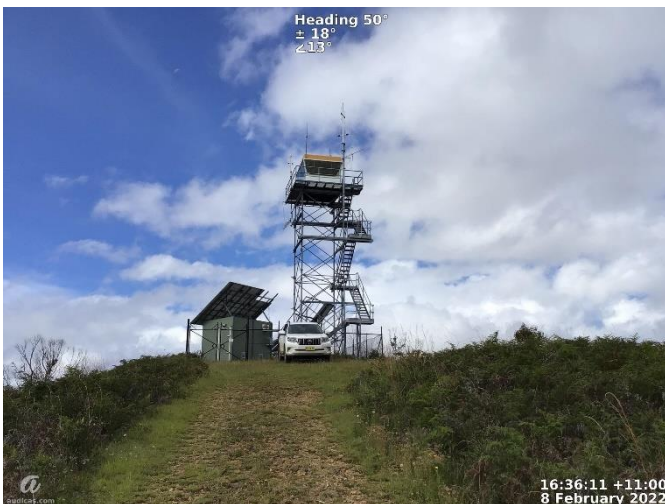
View to the existing radiocommunications facility and fire lookout tower facing north-east
