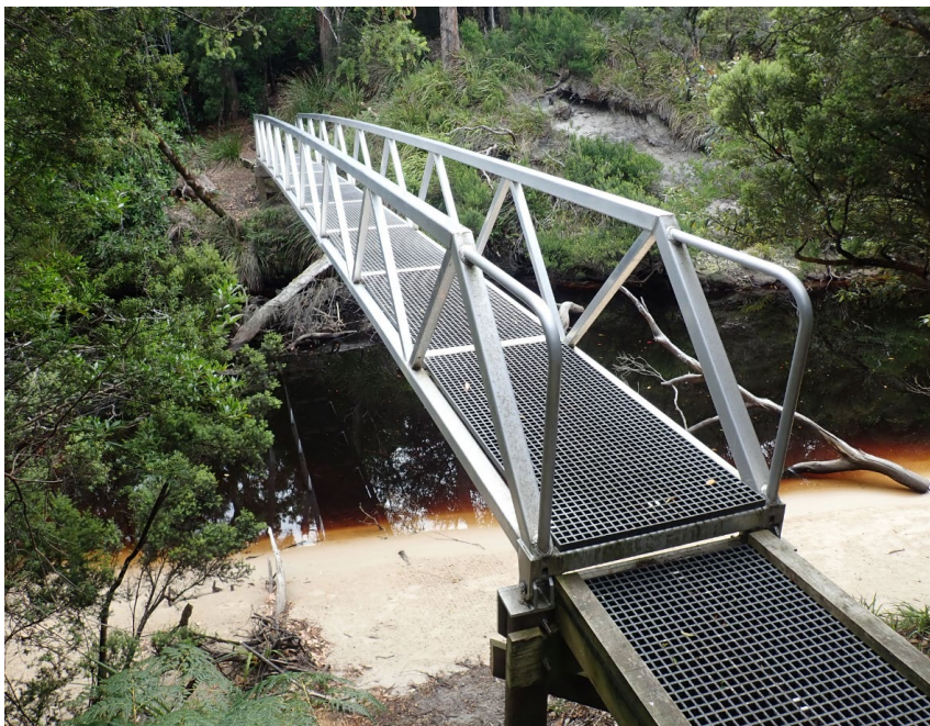
Figure 12 Example of type 4 pedestrian fixed bridge (Photo: Tasmanian PWS)
