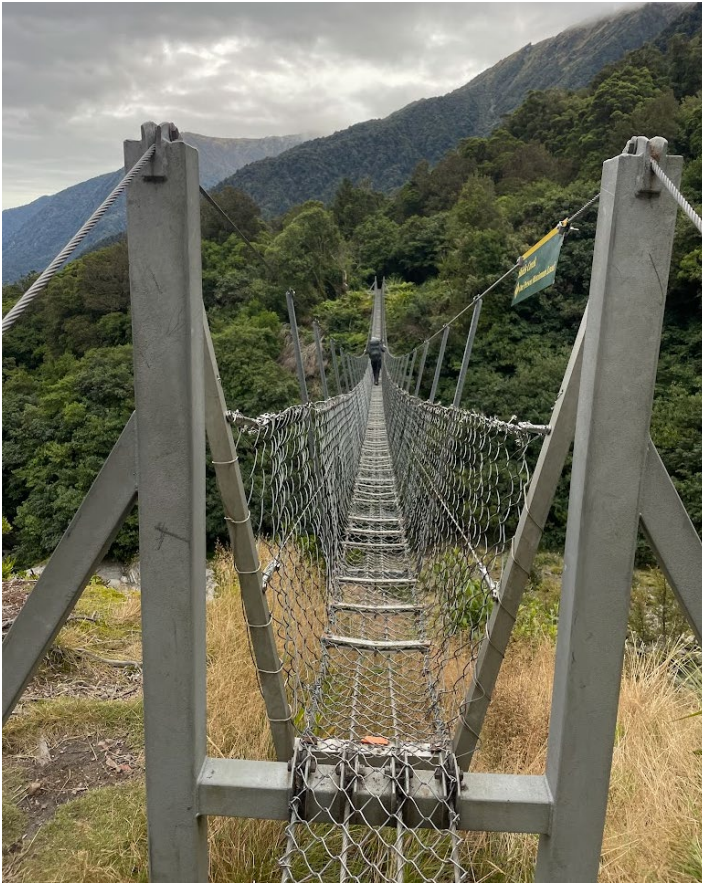
Figure 13 Example of type 4 pedestrian suspension bridge (Photo: NZ DOC)
