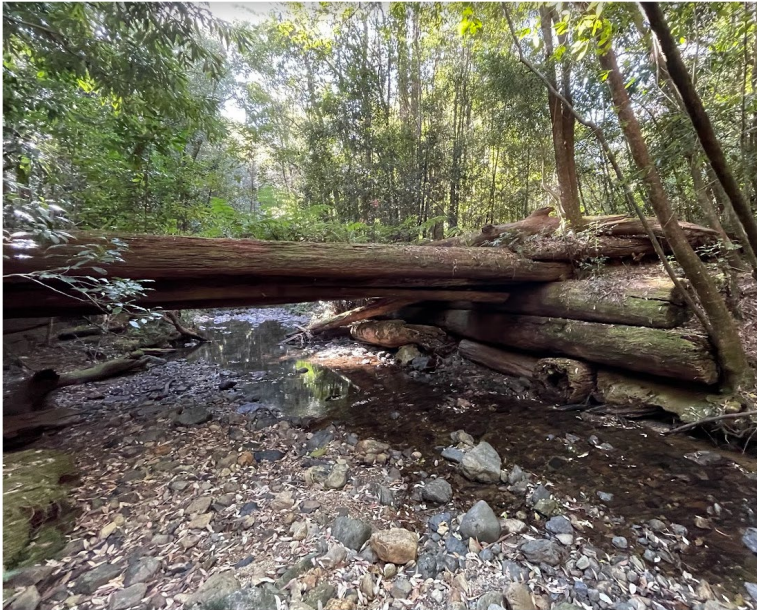
Figure 46 Existing Bridge at Urumbilum picnic area
