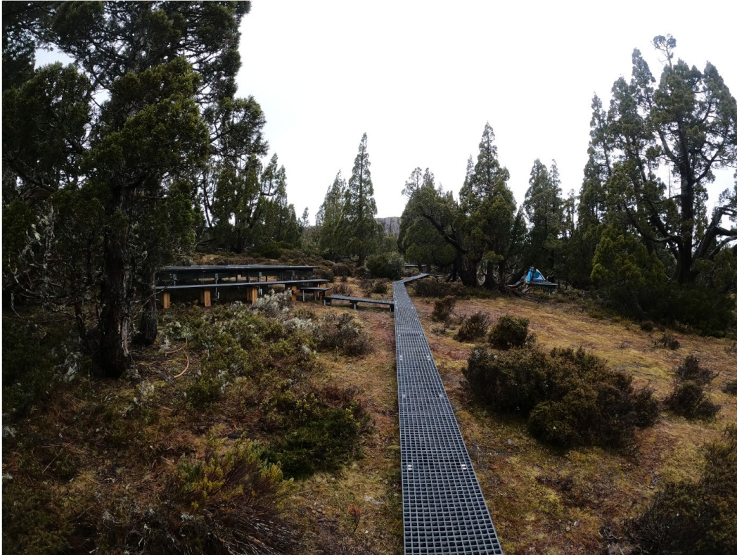
Figure 33 Example of elevated camp boardwalks and camping platforms – Walls of Jerusalem, Tasmania
