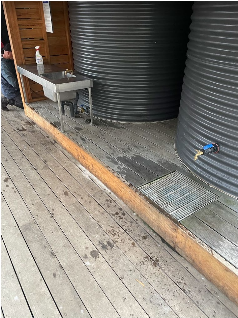
Figure 31 Example communal hut external water/dish washing facility
