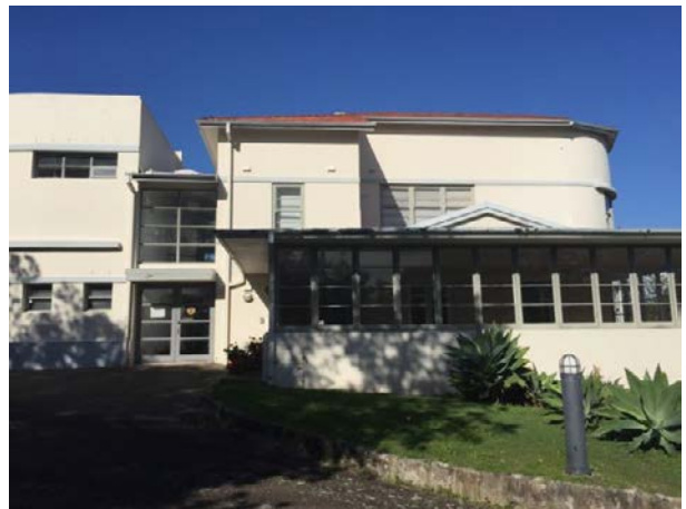
Plate 37. Front of the building – largely sealed for car-parking.
