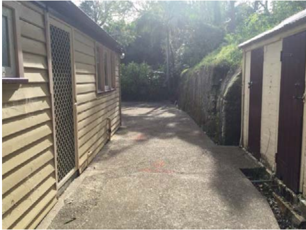
Plate 42. Rear of the dwelling with sandstone ~2m high.
