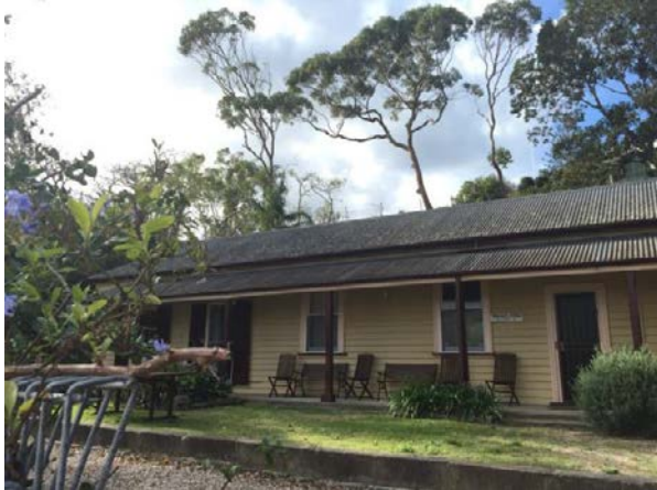
Plate 38. Front of Constables Cottage
