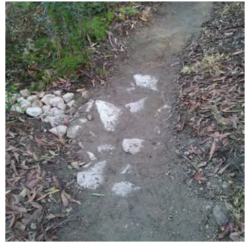
Hardened Spoon drain with HSW
