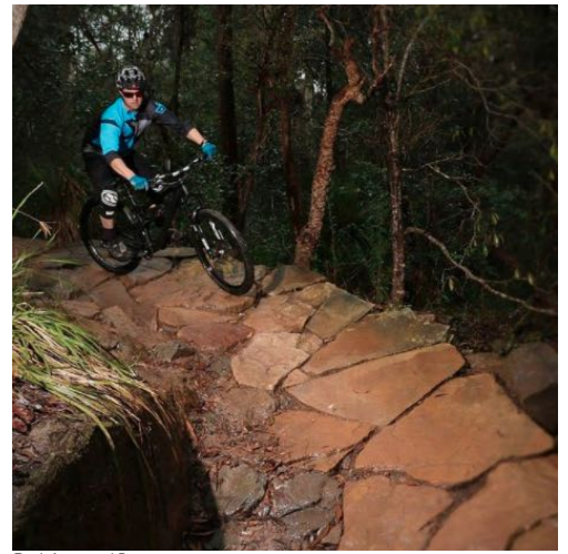
Rock Armoured Berm
