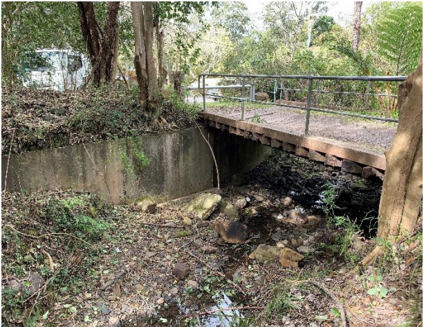
Plate 41: Footbridge in Memorial Pathway (Source: Niche)
