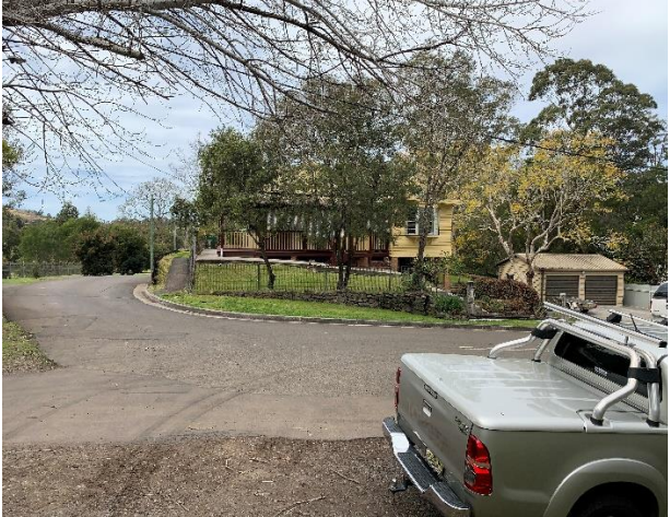
Plate 39: View of Listed Cottage from Memorial Pathway (Source: Niche)
