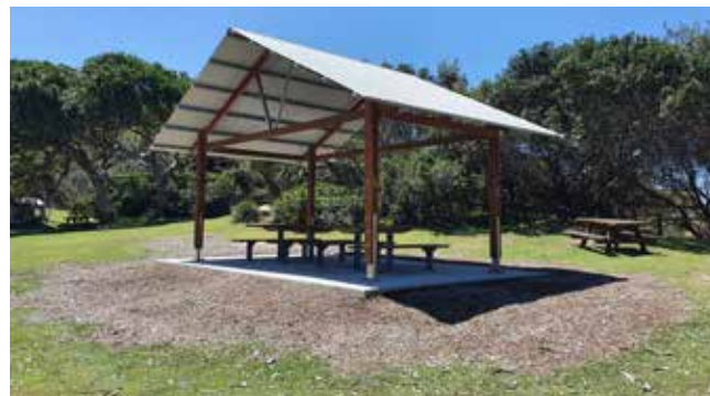
Little Bay - Shelter style to be used throughout the precincts
