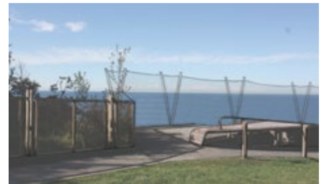
Porous lookout points using webnet mesh
