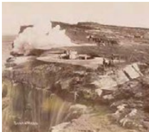
View of the South Head fort 1900–1910, showing the 2 1876–77 gun emplacements
