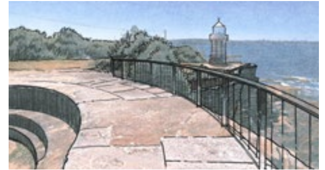
Balustrade with timber handrail
