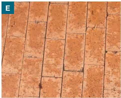
Existing (E) track condition, red brick paving
