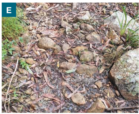
Existing (E) track condition, informal "wild" track
