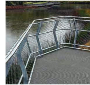
FRP mesh floor, galvanised steel handrail, steel balustrade
