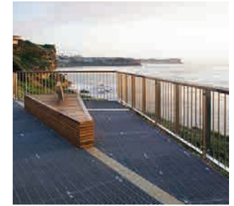
FRP mesh floor, timber handrails, steel balustrade and timber handrail
