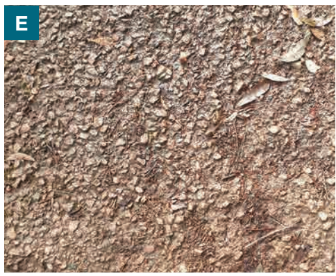
Existing (E) track condition, concrete with local stone aggregate
