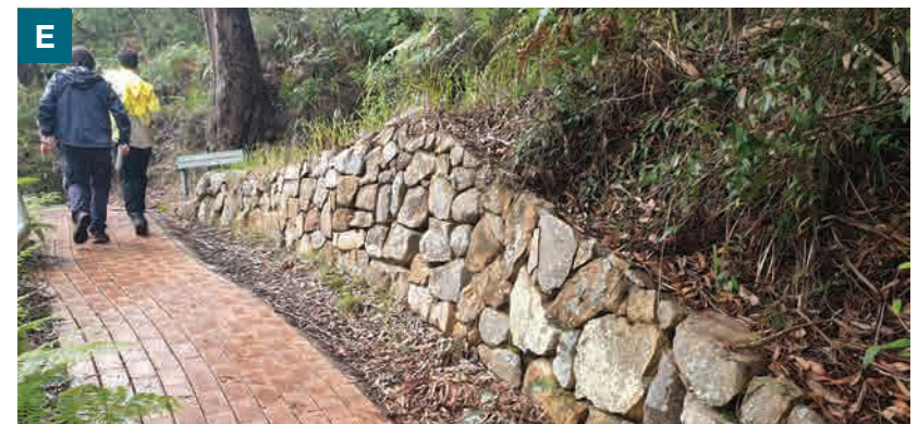
Existing walkway to Tomaree Summit
