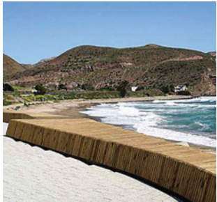
Steel frame timber batten surfer bench
