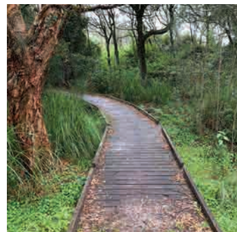
Timber boardwalk structure
