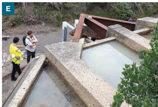
Gun Emplacement structure at Tomaree Head
