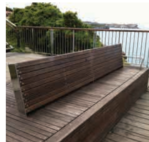
Steel frame timber batten seats
