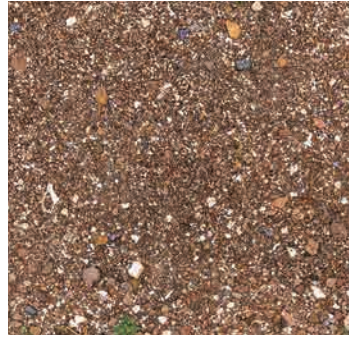
Residual eroded and crushed stone build up
