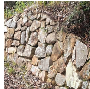
Stone retaining wall
