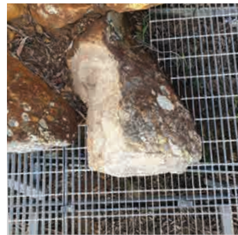
Grate cut around rock face
