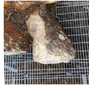
Grate cut around rock face
