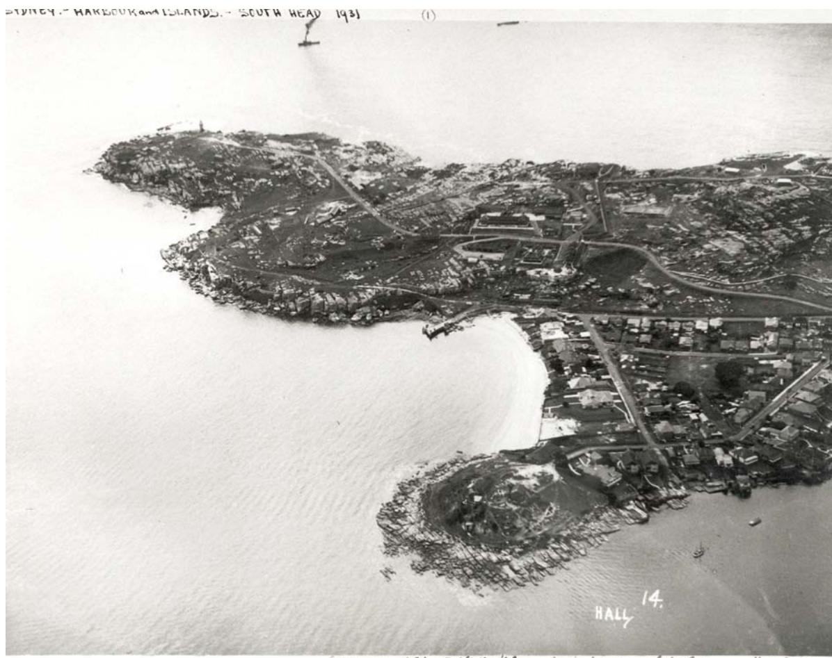
A 1931 aerial photograph showing the extent of fortifications at South Head and Green Point.
