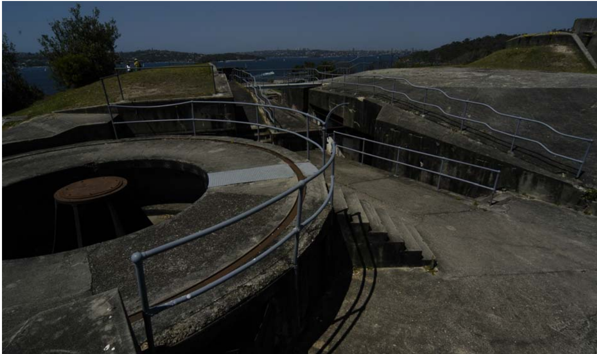
Figure xxi Outer Middle Head showing the extensive network of tube rail fencing installed in the past to protect visitors, however while some edges are fenced most are not. The fence in the immediate foreground for example protects a low drop-off, but other gun emplacements do not have fencing with a similar drop-off. Inconsistencies in approach may expose NPWS to claims as this fence clearly recognises a risk and that should be applied consistently. A better approach would be to remove some of this fencing and to only provide fencing where risks are high.
