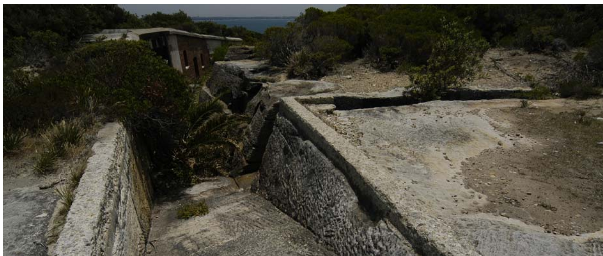
Figure xviii Regrowth at Henry Head in areas of stone cutting that are causing serious deterioration to very significant stonework, to access and interpretation.
