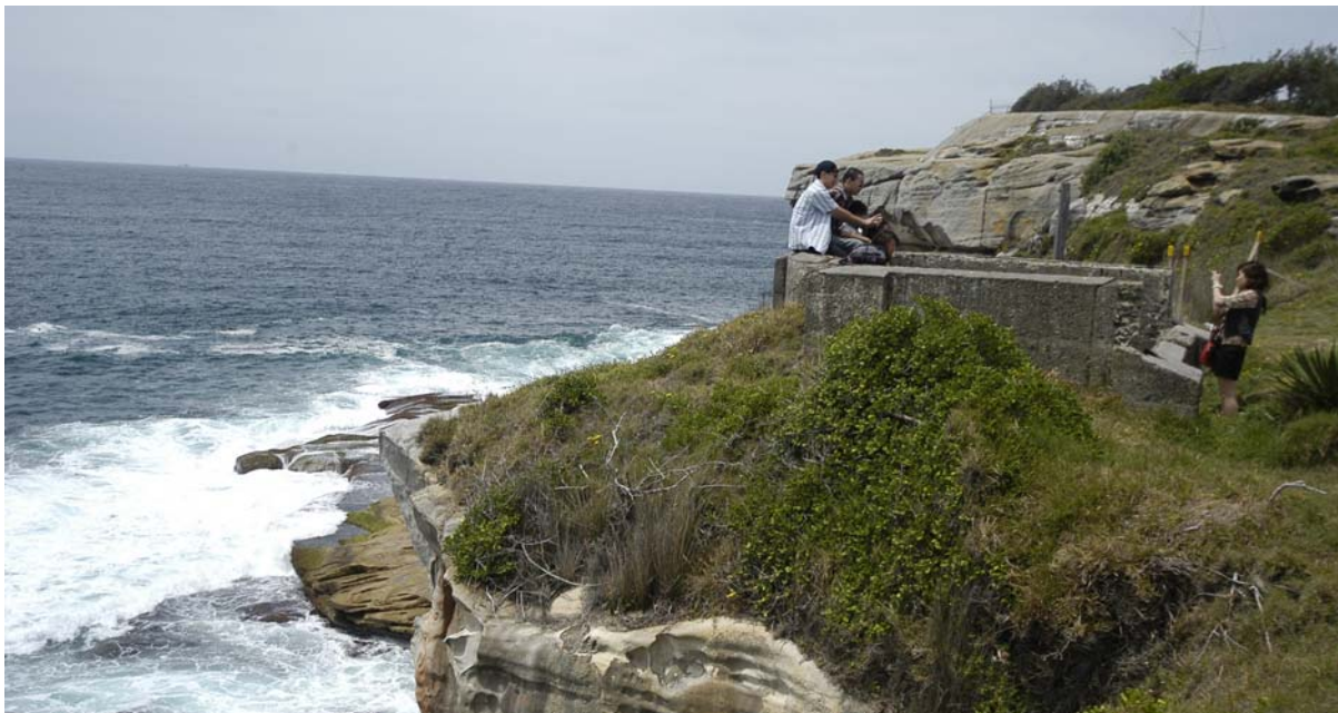
Figure xxii South Head adjacent to Hornby Light showing the difficulties of unprotected access to cliff top features. This is a highly visited location that is used for many photographs and has high risk due to the dangerous behaviour of visitors. Here consideration of a barrier, possibly low and behind this popular photo location would reduce risk.
