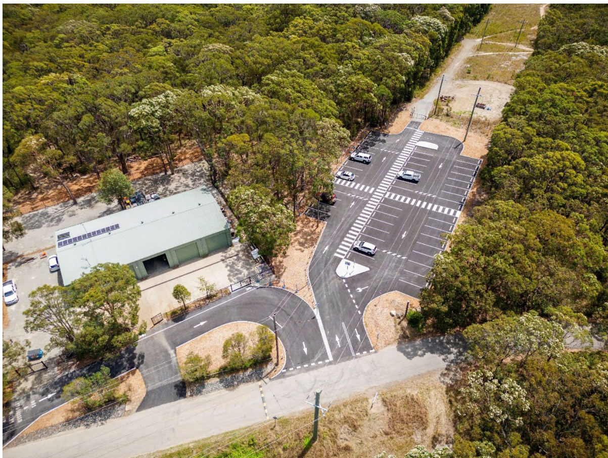
Photo 13 Angophora visitor node car park and NPWS works depot, Glenrock State Conservation Area. John Spencer/DCCEEW
