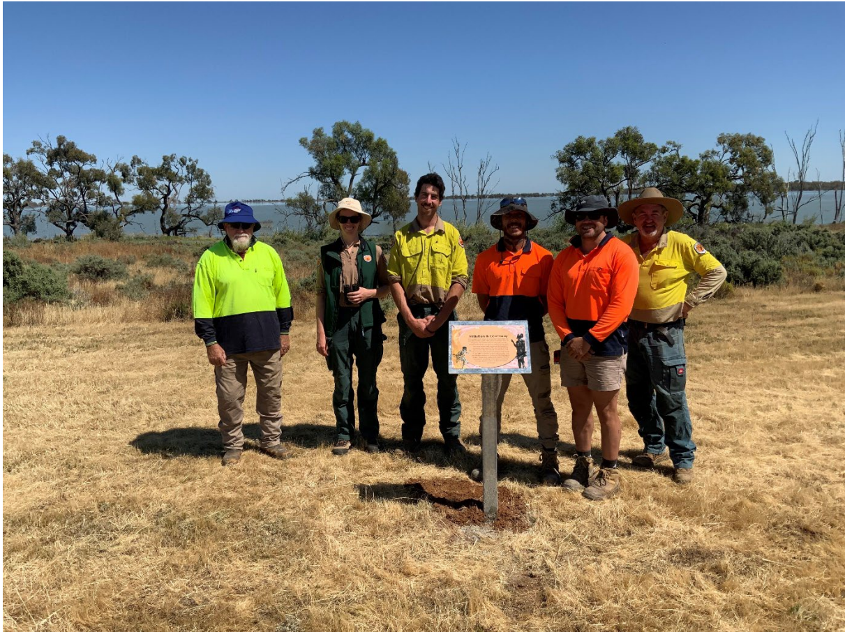
Photo 2 Mawambul and NPWS working together to install signage at Ita Lake Cultural Centre, Kalyarr National Park. Gary Currey/DCCEEW
