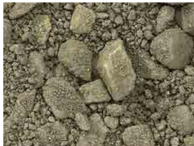
P2 Crushed Rock Gravel Footpath
