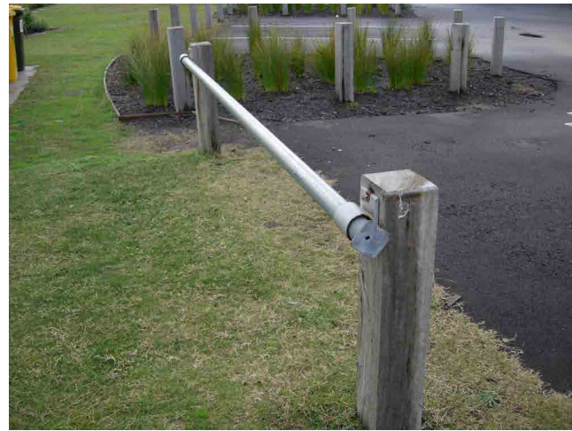
B2 Slip rail vehicle barrier
