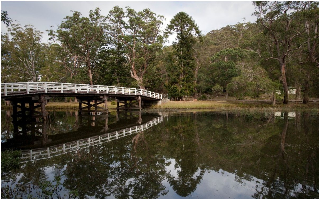
Photo 12 Varneys Bridge and Currawong Flat Picnic Area, Audley. Nick Cubbin/DPE
