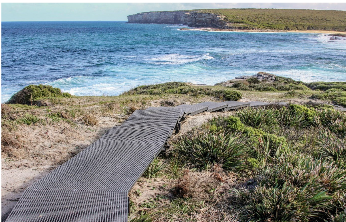
Photo 19 New board walk on the Coast Track, Royal National Park. David Croft/DPE
