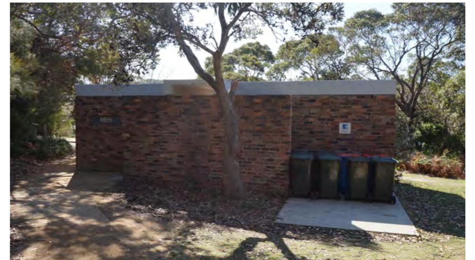
Fig22. Toilets and bins (CONTEXT 2015)
