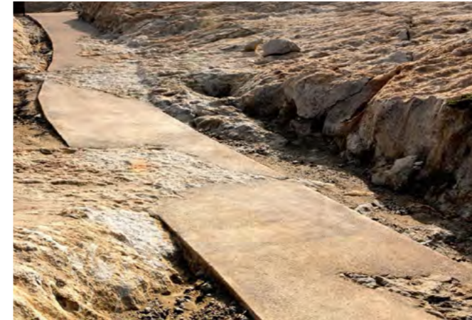
In situ concrete
