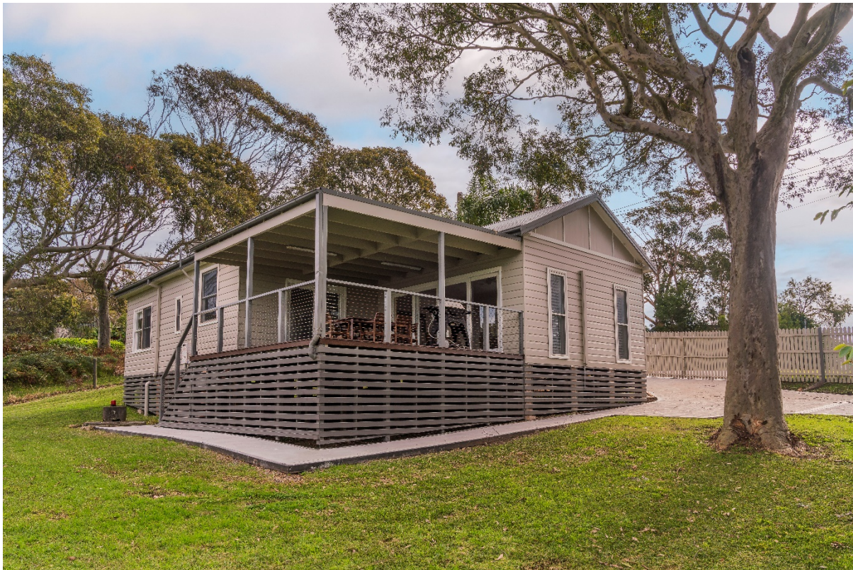
Photo 5 Baileys Cottage. John Spencer/DPE
