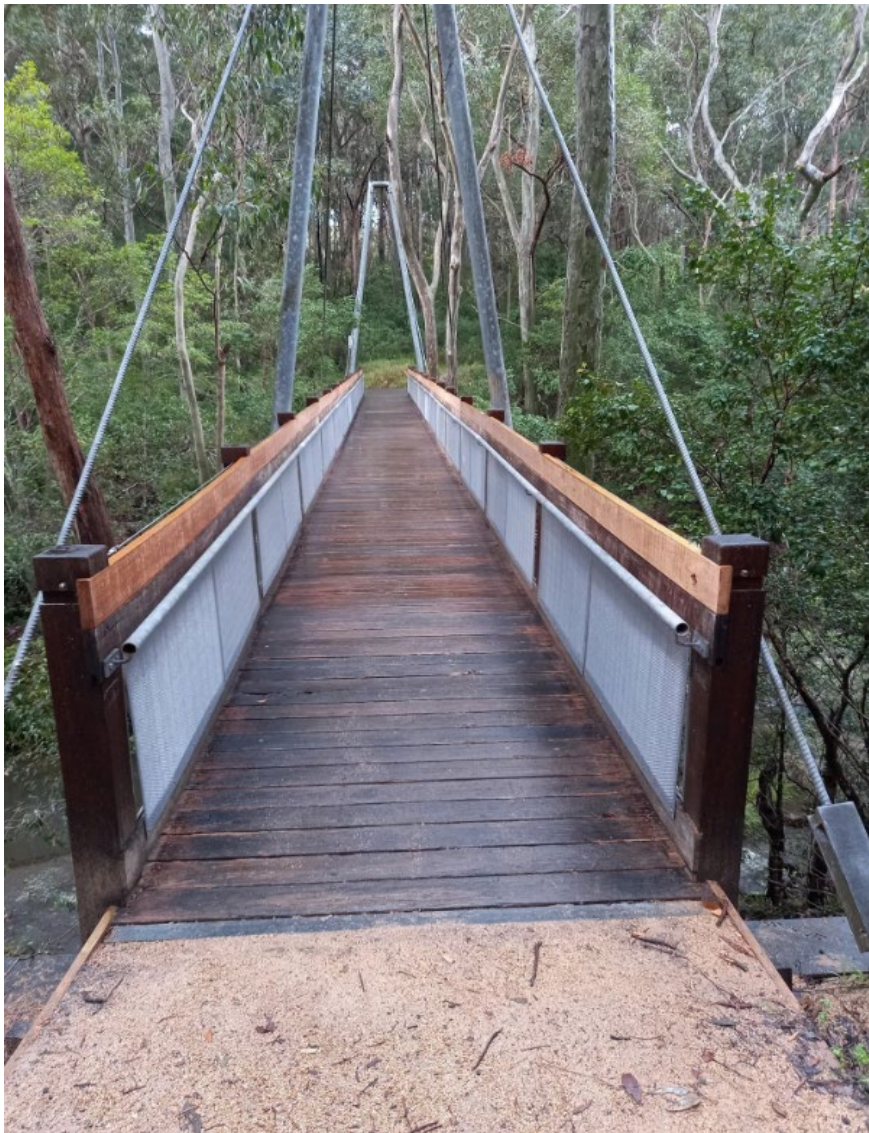
Photo 8 Yuelarbah Track – bridge over Flaggy Creek. Simon Rosenthal/DPE
