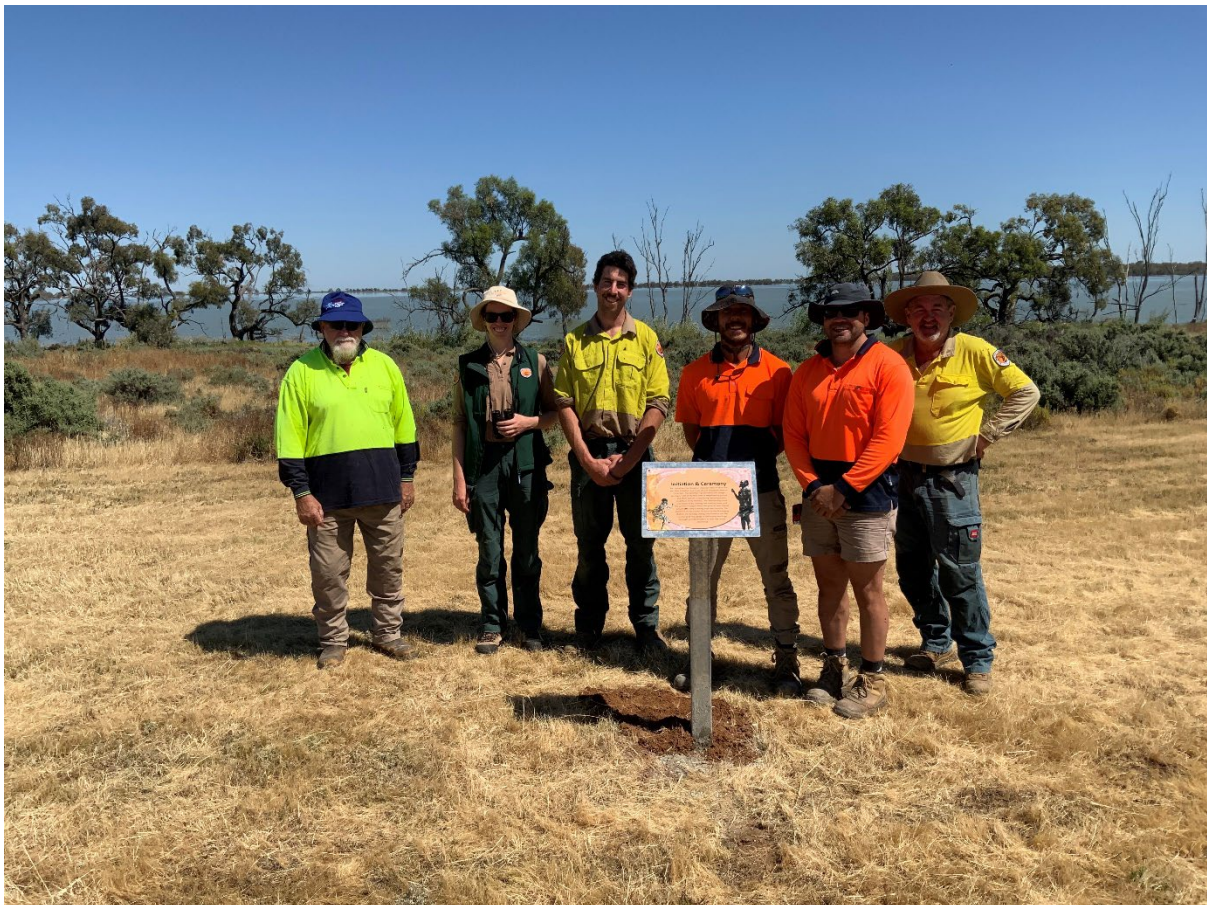
Photo 1 Mawambul and NPWS working together to install signage at Ita Lake Cultural Centre, Kalyarr National Park. Gary Currey/DCCEEW
