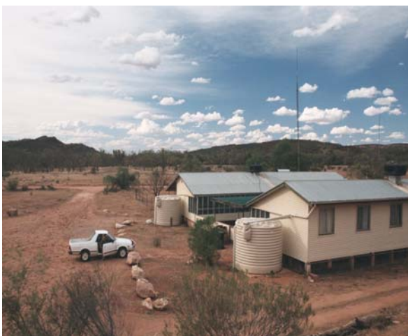
Shearers’ Quarters - an accommodation, discussion and social area.
