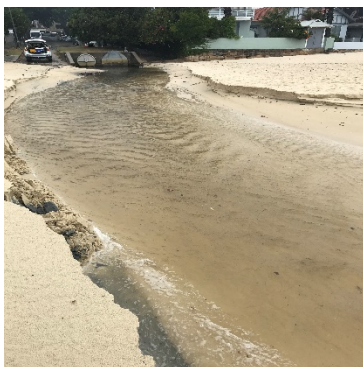
Stormwater drain flow Photo: Beachwatch/DPE
