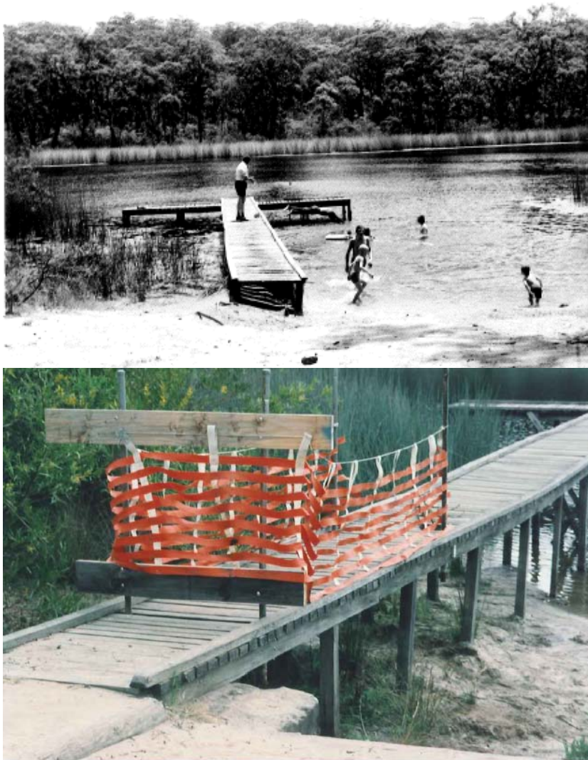
Figure 5-5. Upper photograph, taken by Vorst in May 1974 showing water level relative to jetty (source: Fanning) and lower photograph, taken late 1997 shows jetty relative to concrete wall (source: NPWS).
