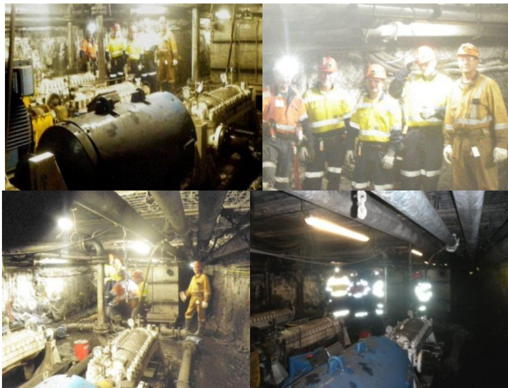
Figure 6-30. Committee inspection of Tahmoor Mine and Pit Bottom pump station.
