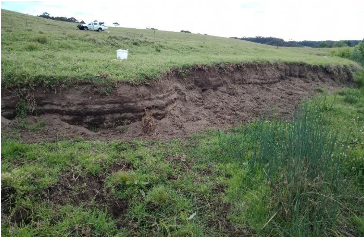
Photo 11 Bank erosion at site VC4 (U Pinto, 4 November 2019)
