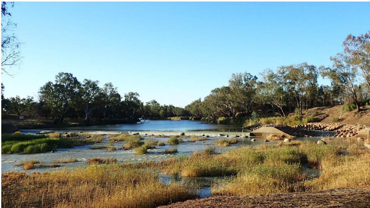
Figure 19 Brewarrina weir and fishway Photo: David Preston (DPIE)
