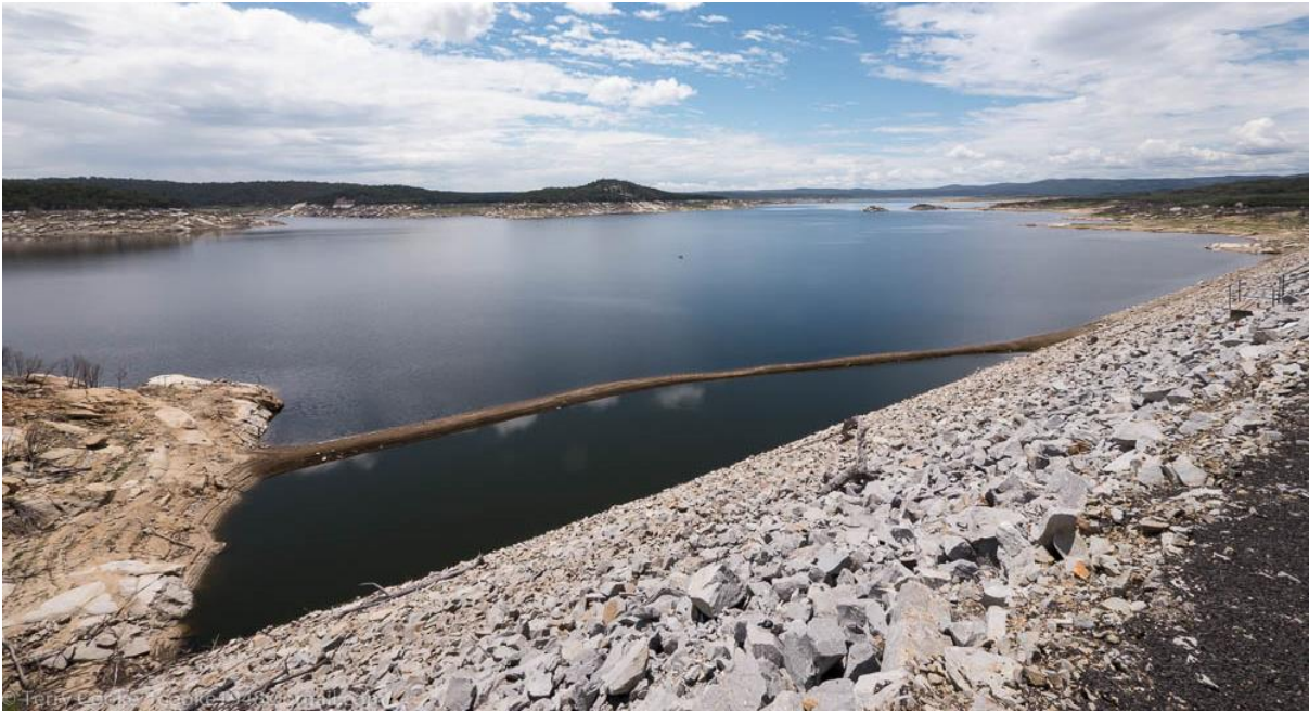
Figure 14 Copeton Dam on the Gwydir River Photo: T. Cooke
