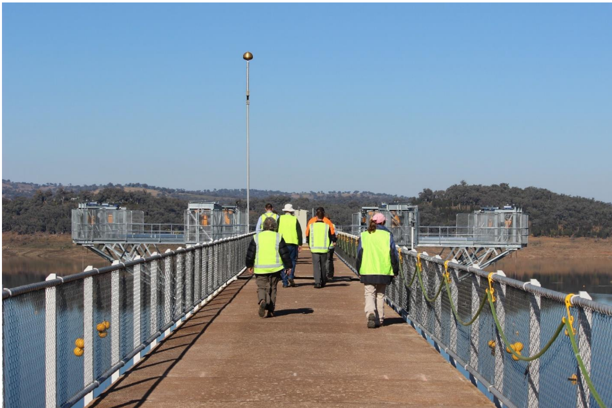
Figure 14 Burrendong Dam offtake tower with cold water curtain Photo: Tim Hosking/DPIE
