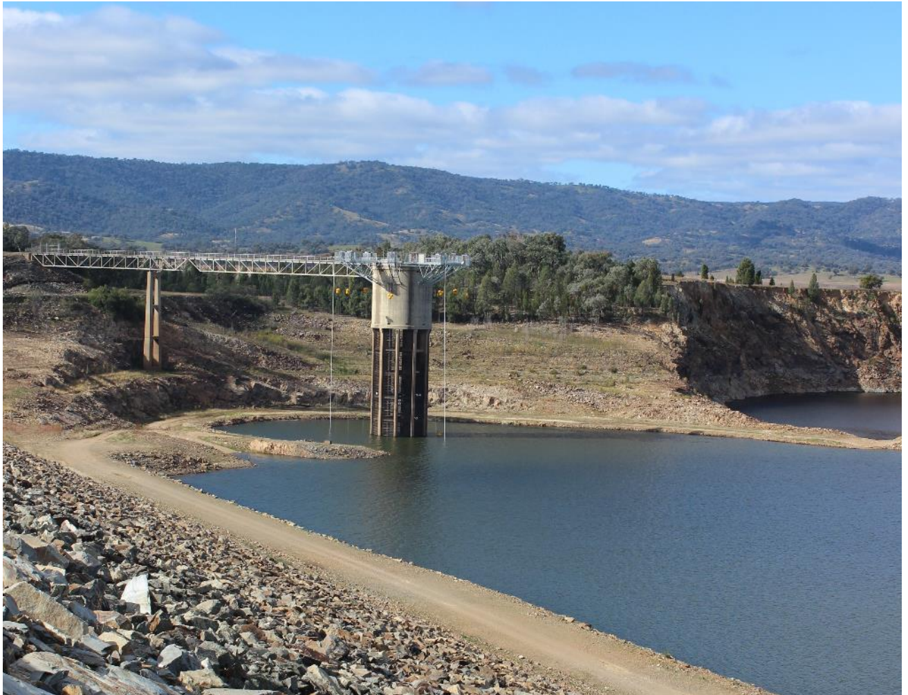
Figure 9 Burrendong Dam offtake tower with cold water curtain Photo: Tim Hosking/DPIE
