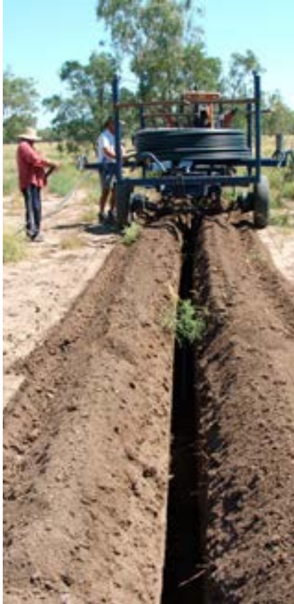
Installing underground waterpipes to save water. DPIE.
