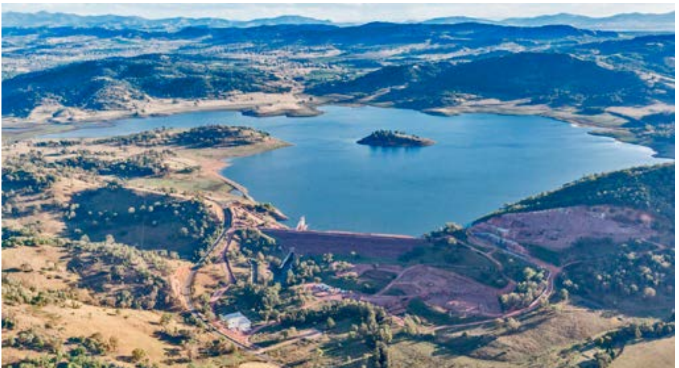
Chaffey Dam, Tamworth. WaterNSW.
