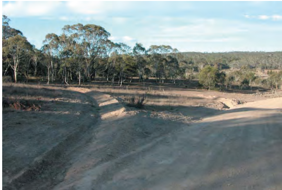
Figure 10. A mitre drain
