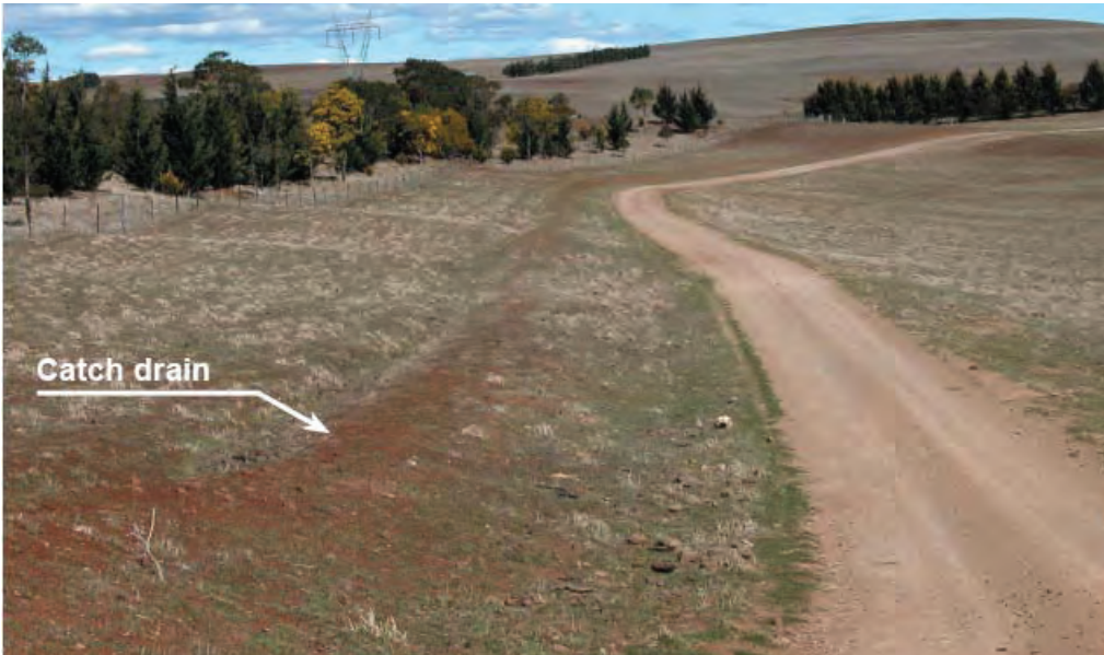
Figure 17. A well-formed catch drain
