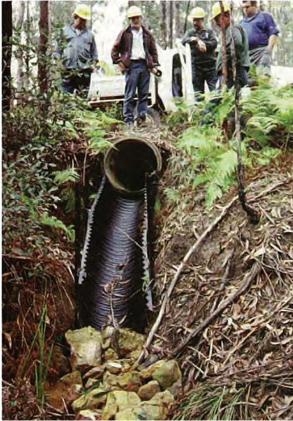
Figure 18. Drop down structure with rock energy dissipator
