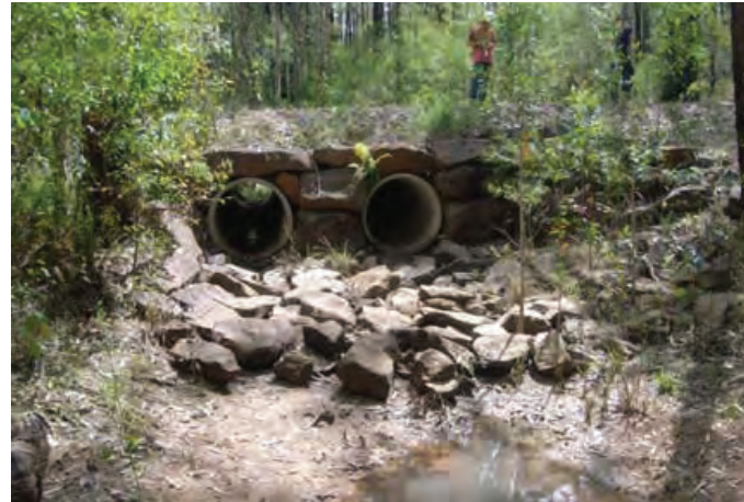
Figure 23. An example of a culvert crossing
