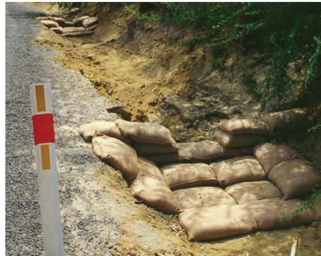
Figure 32. An example of a sandbag check dam
