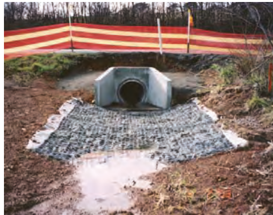
Figure 27. Outlet dissipation structure
