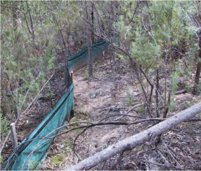
Figure 34. Sediment fencing
