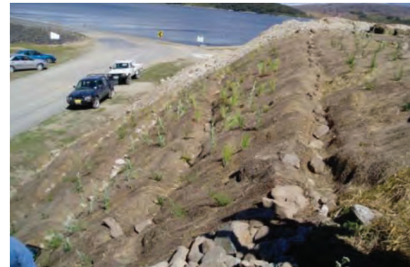
Figures 40 and 41. Spoon drains on batters
