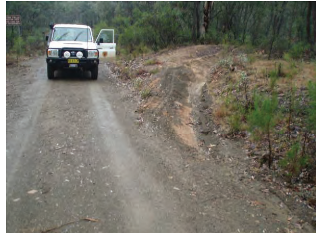
Figure 11. A well-formed mitre drain used in conjunction with crowning crossfall
