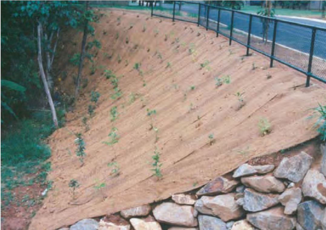
Figure 31. An example of erosion control matting used to stabilise a batter
