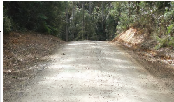
Figure 5. Crowning of the road surface
