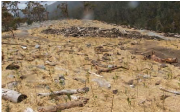
Figures 38 and 39. Offset cross logs with tubestock
