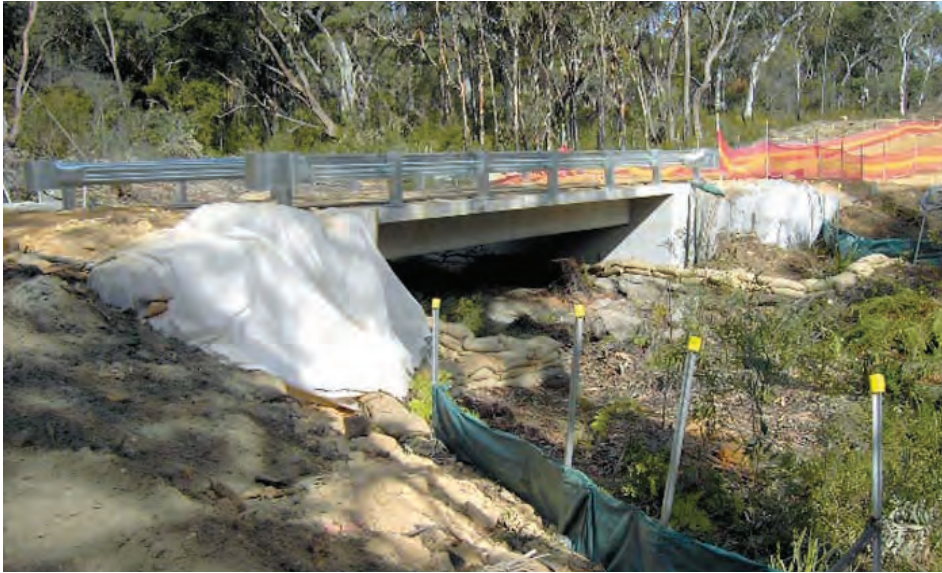
Figure 20. Erosion and sediment control measures around bridge abutments
