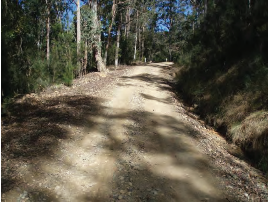
Figure 7. An example of effective infall drainage
