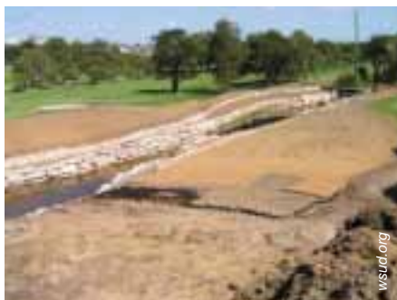
Jute matting prevents bank erosion – wetland reconstruction, Strathfield
