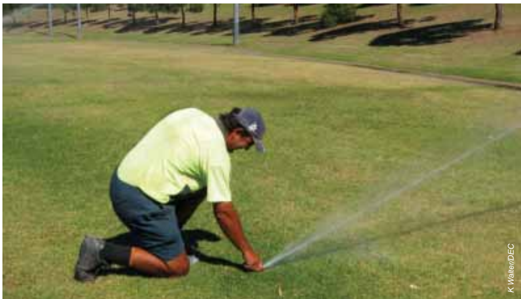
Checking the stormwater irrigation system at Greenway Park, Cherrybrook
