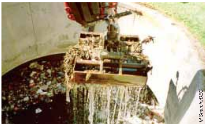
Trash removal, Centennial Park
