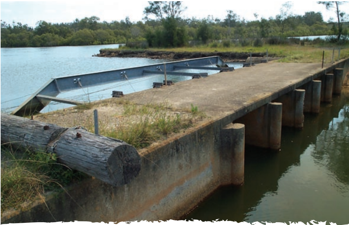
Floodgate Yarrahapinni, Macleay River (DECC)
