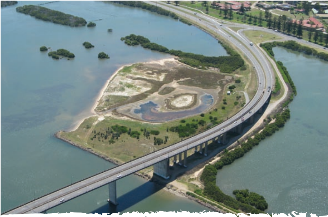
Wader roost constructed at Stockton Sandspit (Kooragang Wetland Rehabilitation Project)
