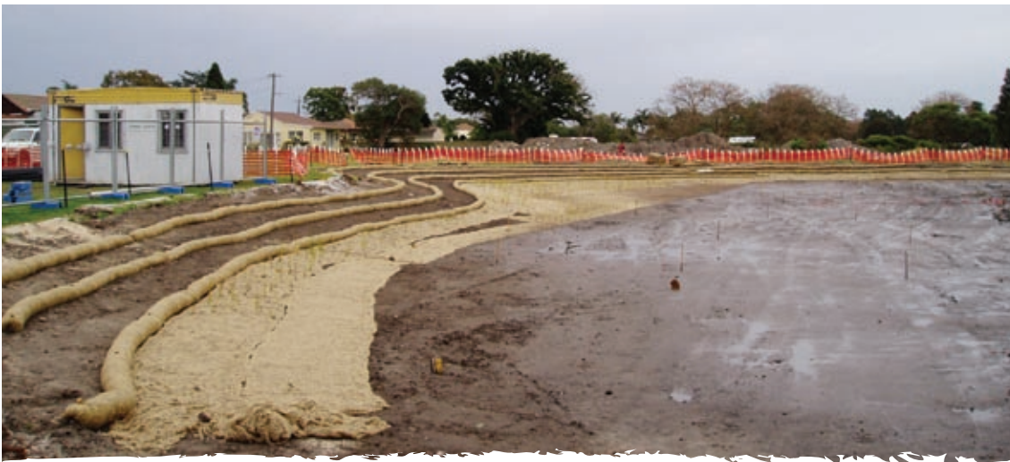
Construction of saltmarsh at Scott Park, Rockdale (DECC)
