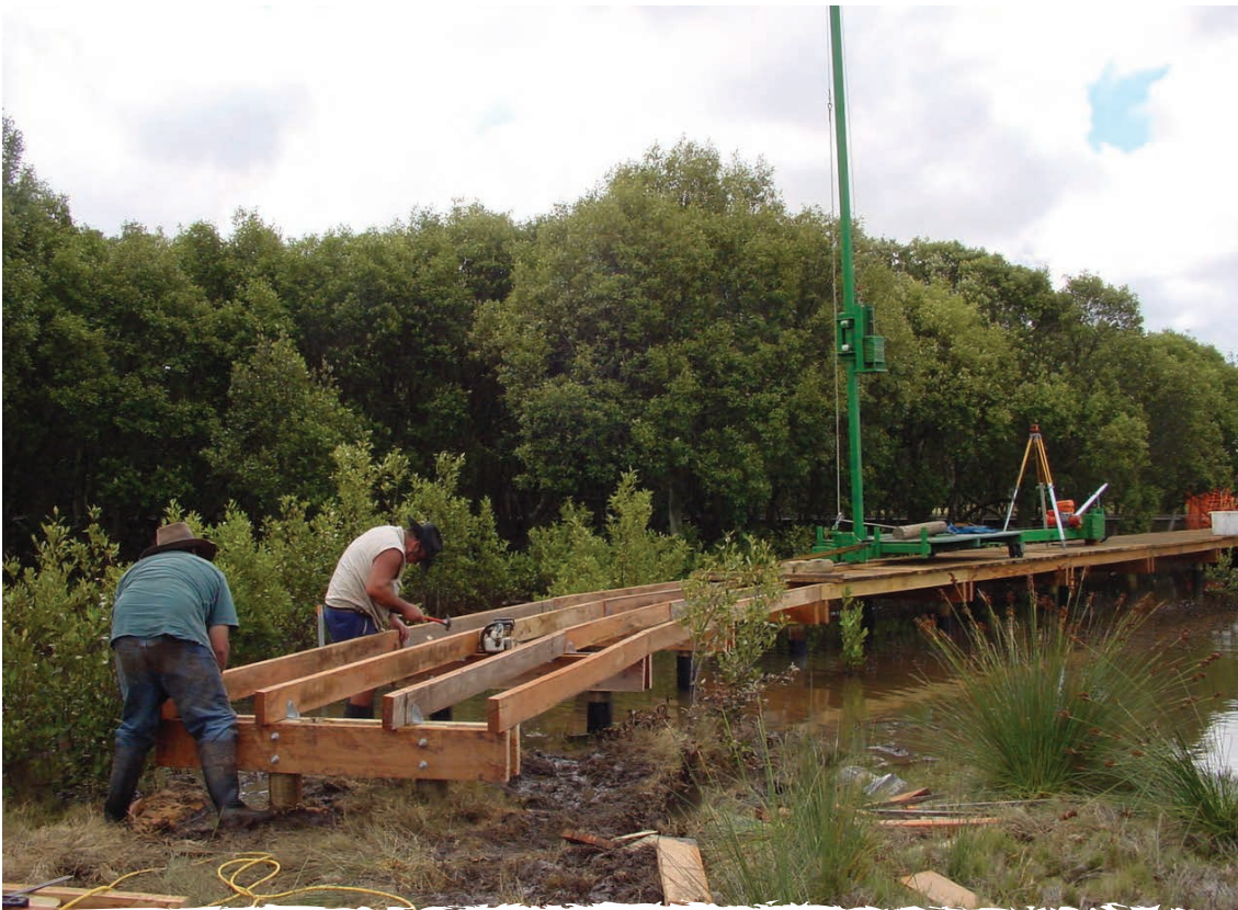
Boardwalk construction (Kooragang Wetland Rehabilitation Project)
